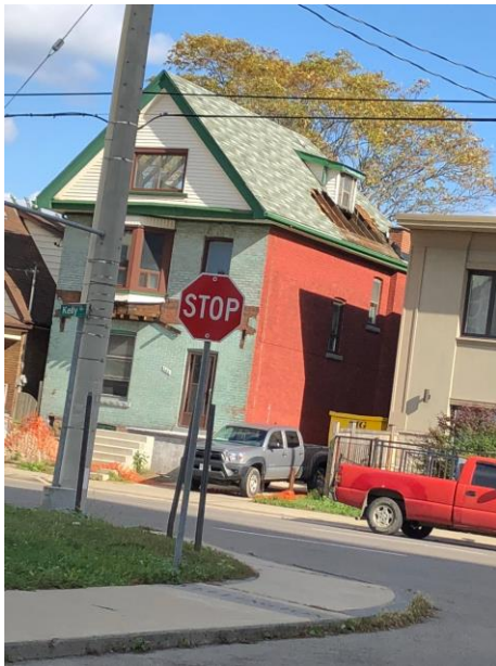
144 Wellington Street North (Before) Source: Applicant
