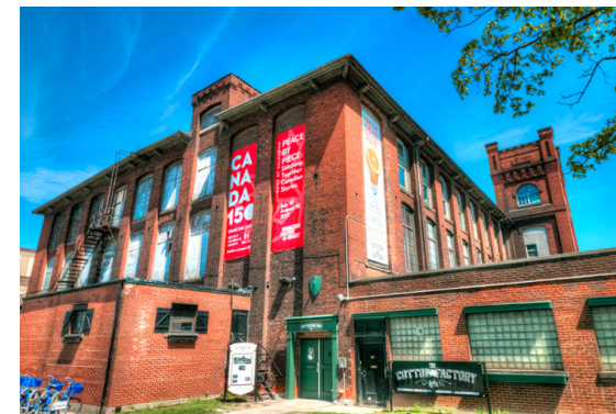
The former Imperial Cotton Co. has been transformed into the "Cotton Factory": a creative industries complex, with space for workshops and small manufacturing, office space for creative professionals, and studios for artists
