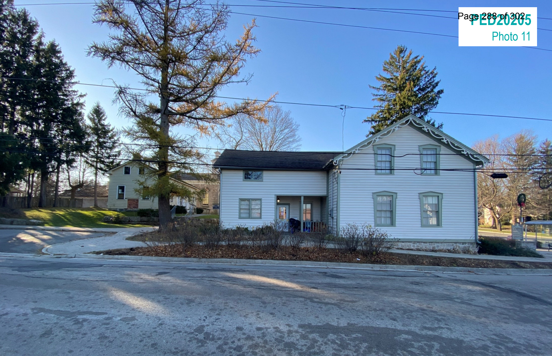
314 Wilson Street East
