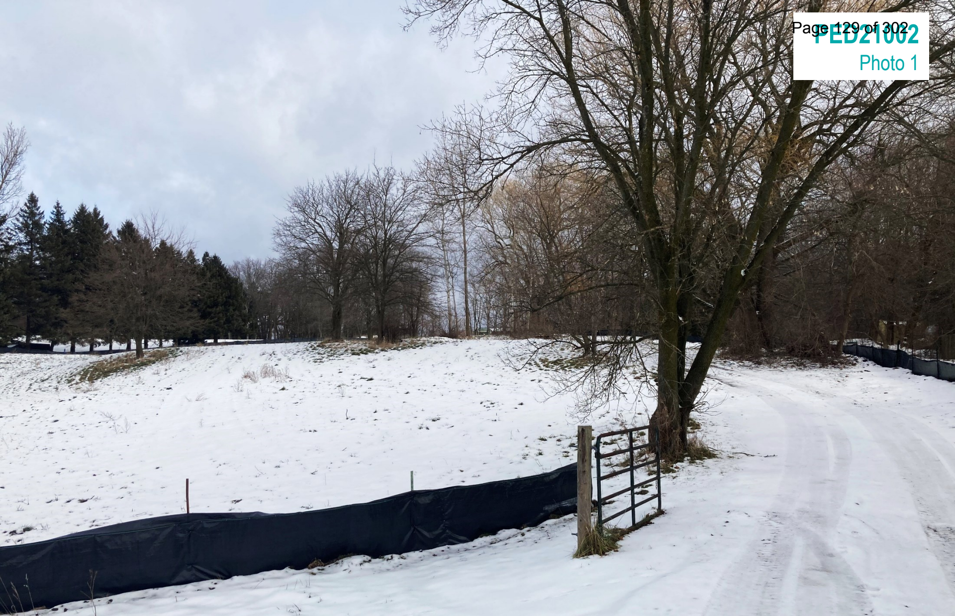
Looking east from site entrance along Highway 52 North
