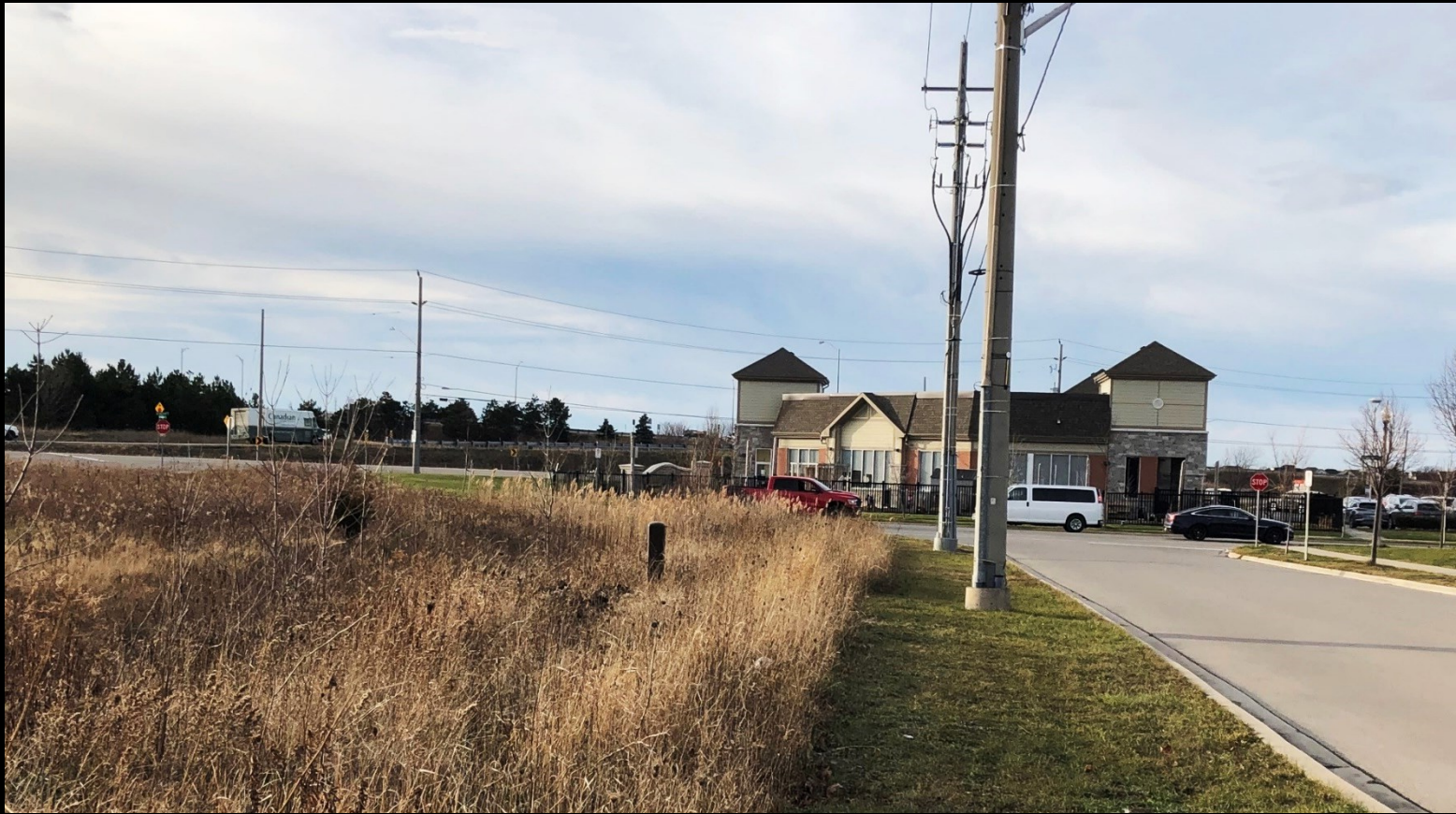
Commercial plaza to the west
