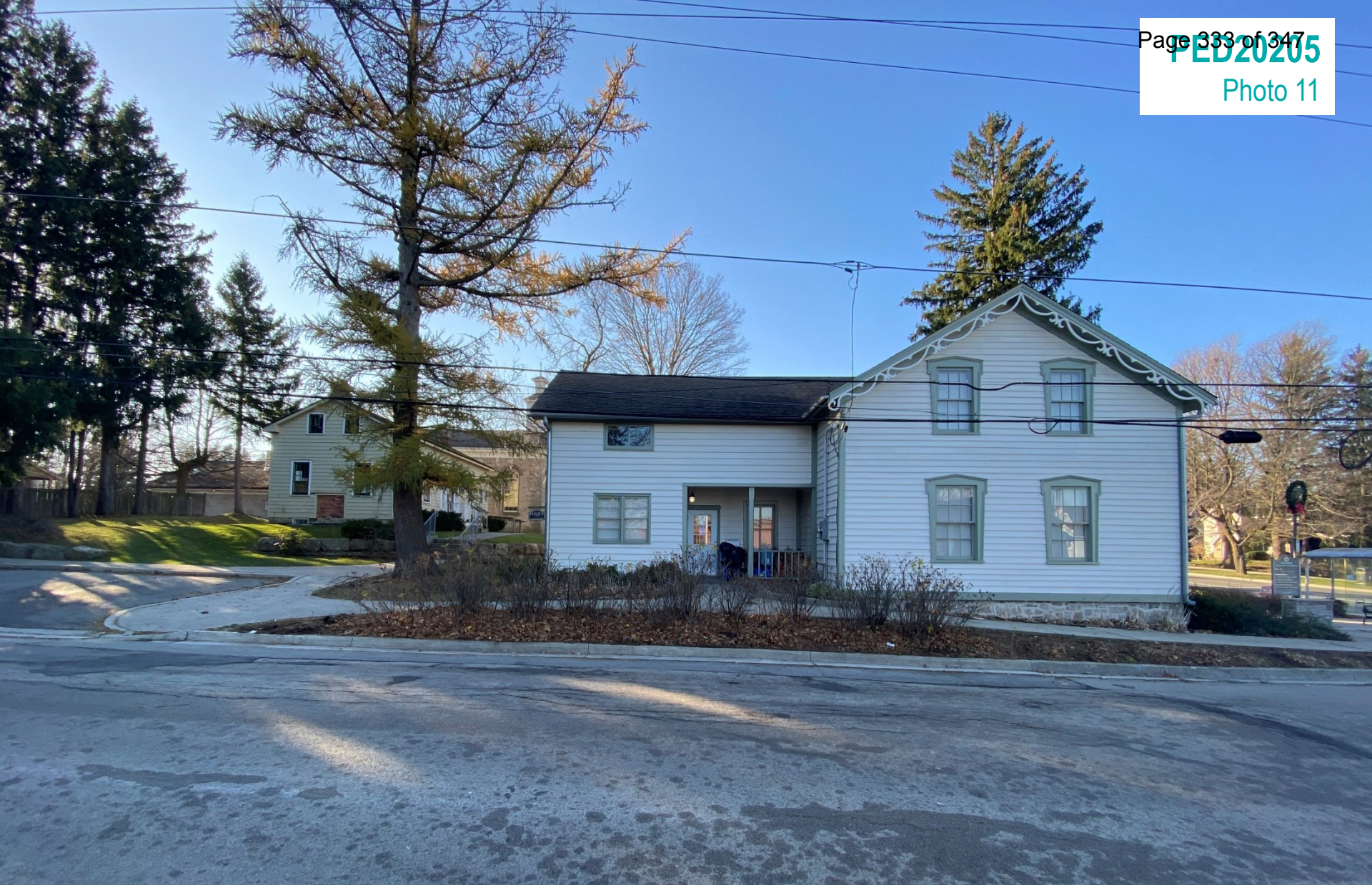
314 Wilson Street East
