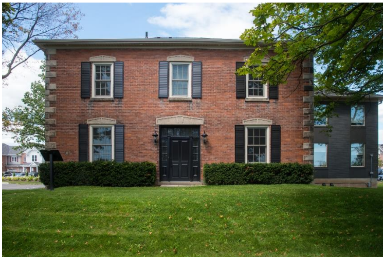
493 Dundas Street East (Front of Property) Source: Applicant
