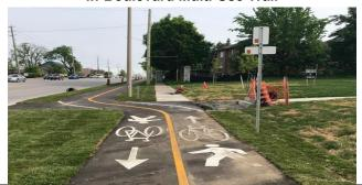
An in-boulevard multi-use path is a twoway travelled path shared by cyclists and pedestrians. These facilities are physically separated from motor vehicle traffic because they are placed above the curb (typically) with a horizontal buffer that may also be used for snow storage.
