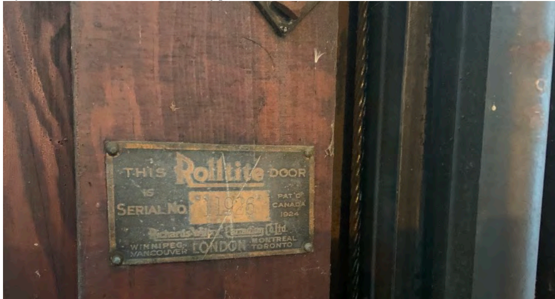
03.12 Builders Plate: "This Rolltite Door" Serial No. 11926 Pat. "D" Canada 1924 Richards Wilcox Canadian Co. Ltd. Winnipeg Vancouver London Montreal Toronto Two doors have sequential number plates. They were likely installed in 1924, 1925 or 1926.
