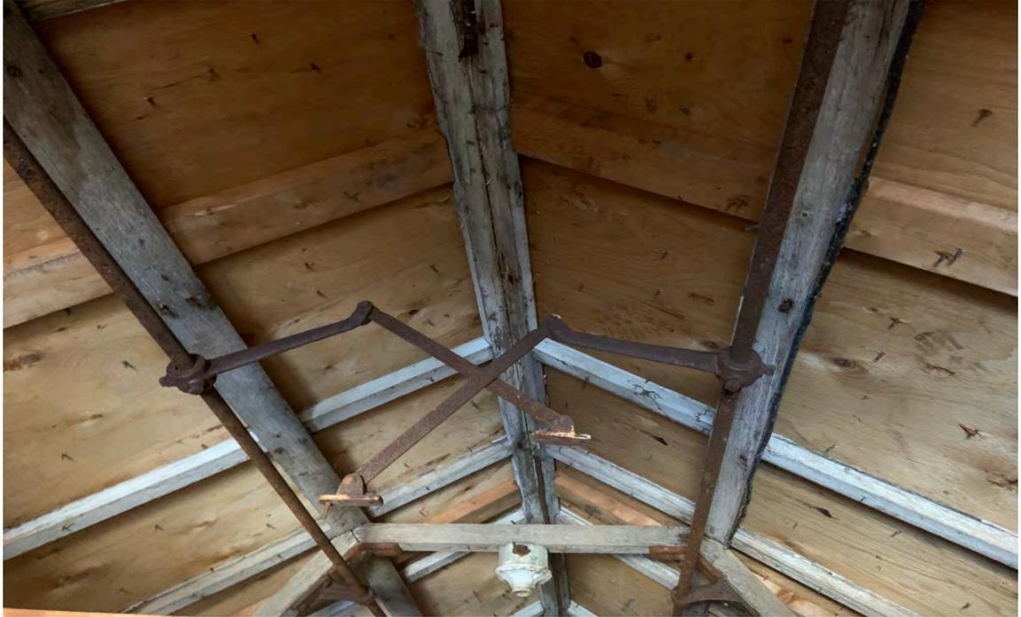
**02.34** A block with a ceramic lightbulb socket is screwed to the center of each collar tie to provide electric light to the space below. The fixtures appear to be contemporary to the early knob and tube type wiring. Note new plywood sheathing on roof to support shingles.
