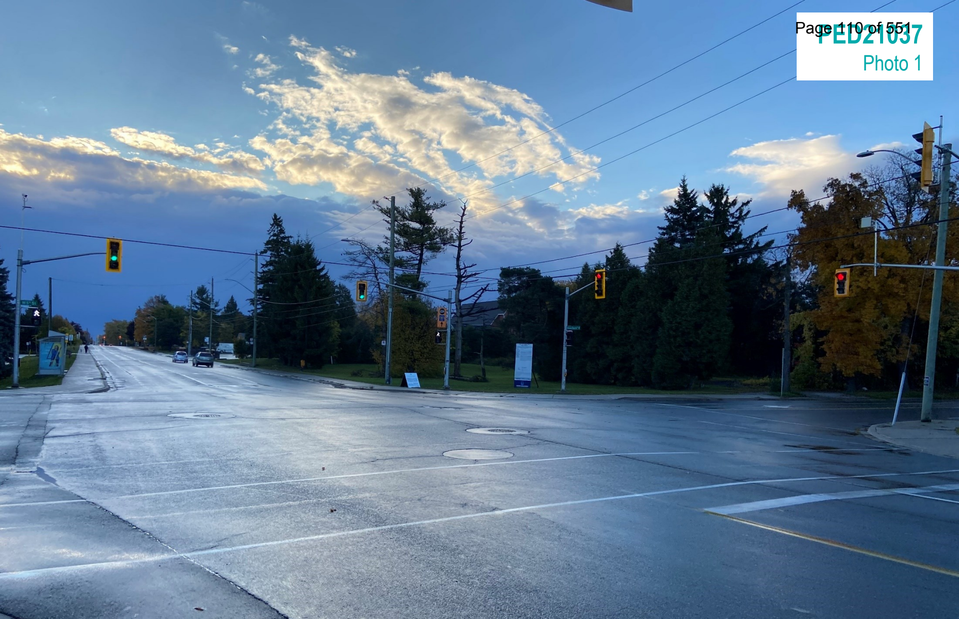
89 Stone Church Road West (looking south east)
