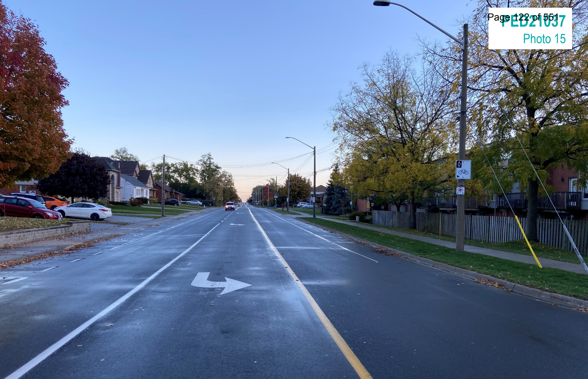
West 5 th Street (looking north)
