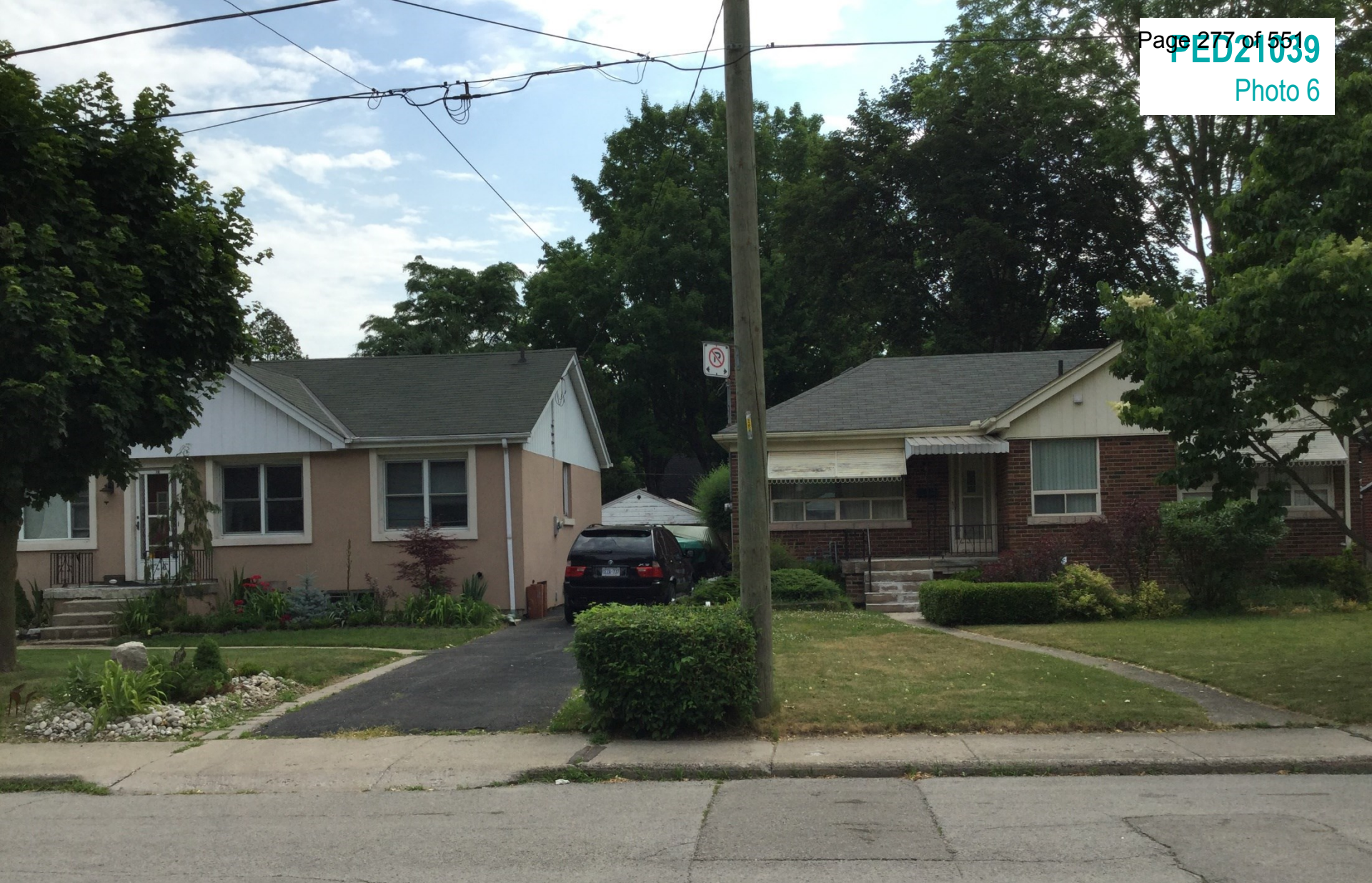
Properties at 8 and 10 Westbourne Road located across the street to the east of the subject property, as seen from Westbourne Road, looking east
