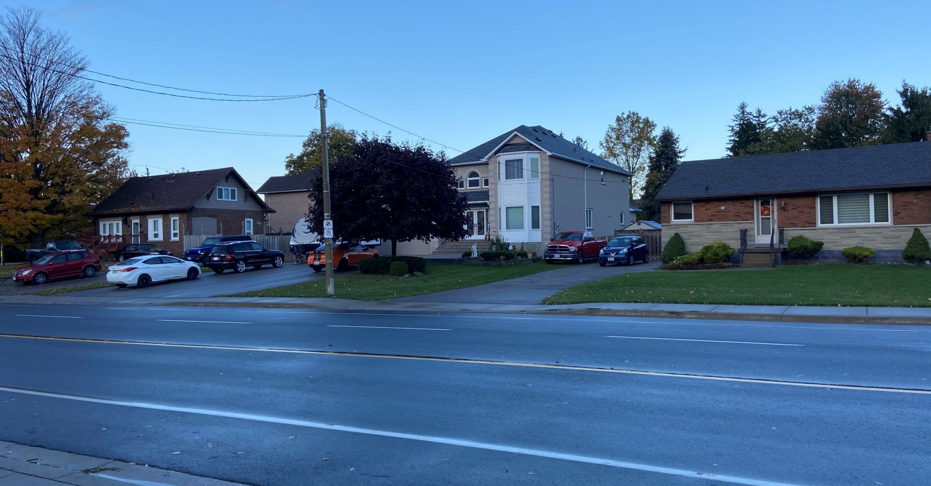
Single Detached Residential (north west of subject lands)
