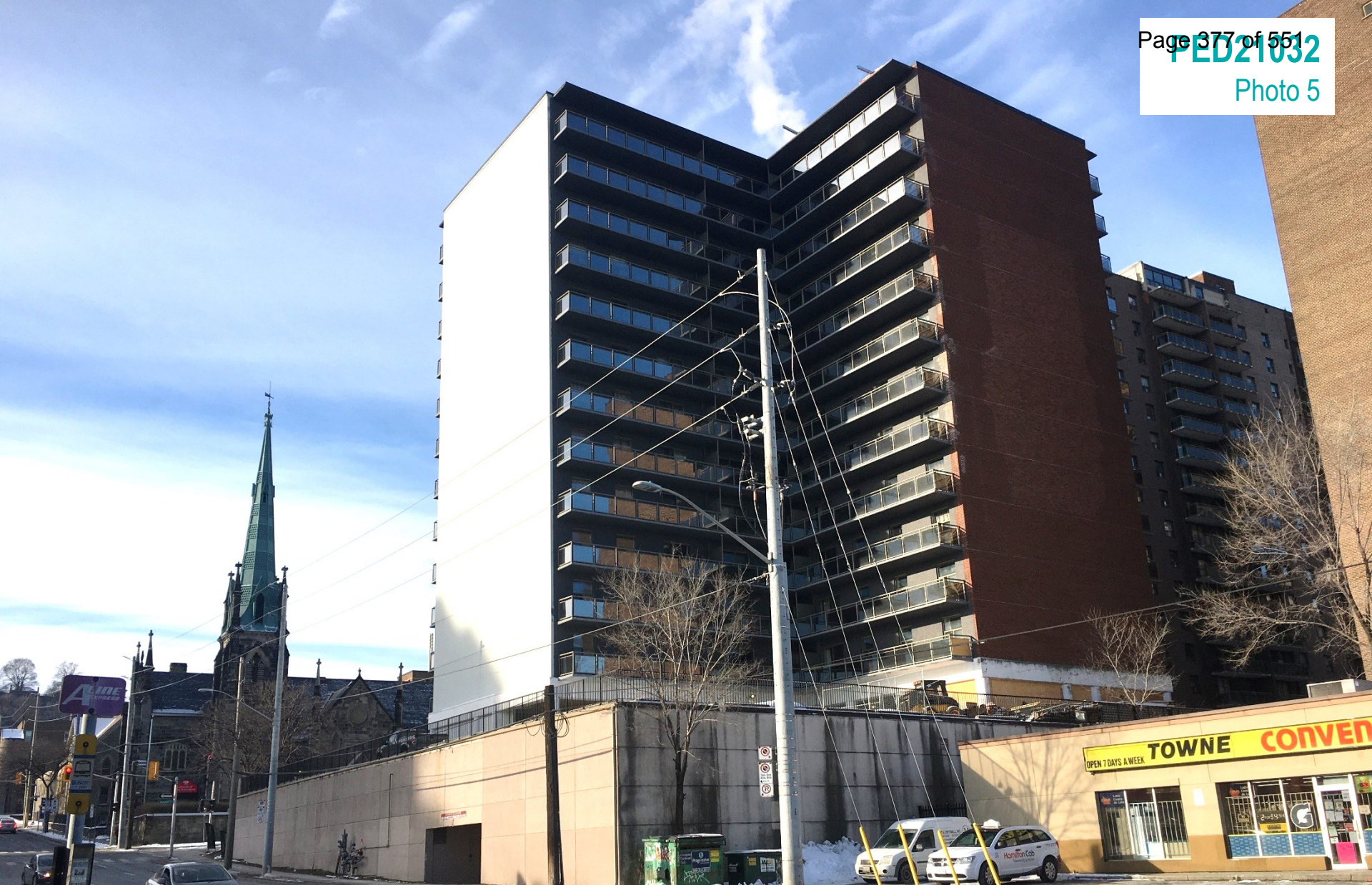
Existing development to the west and southwest as seen from John Street South
