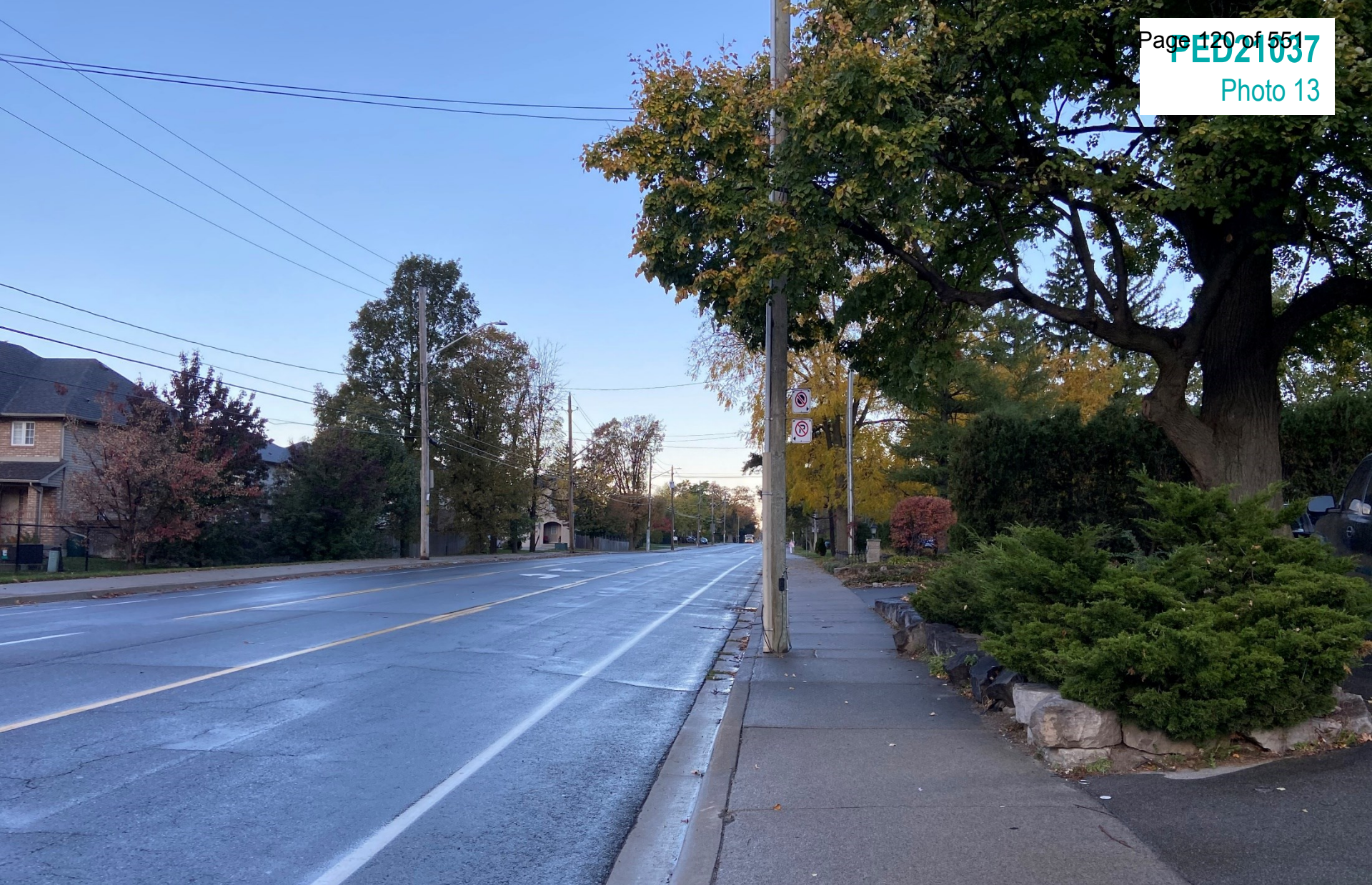
Stone Church Road West (looking west)
