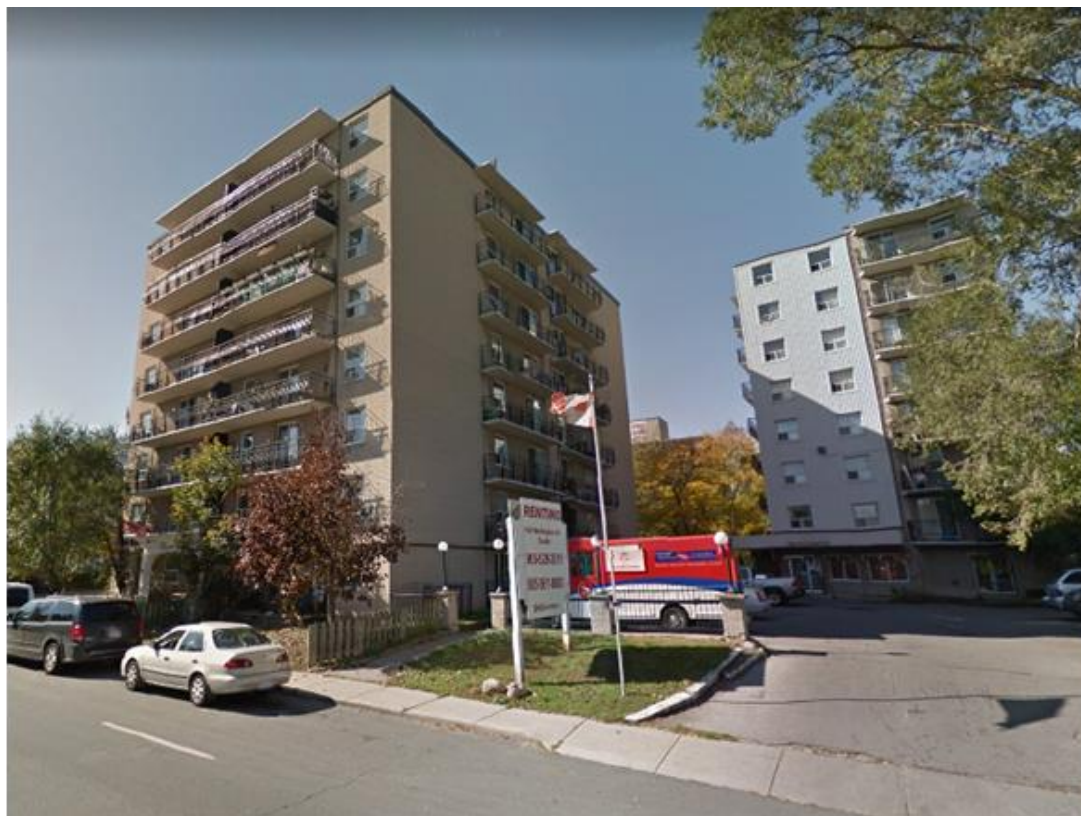
Existing Rental Buildings to South of Subject Property
