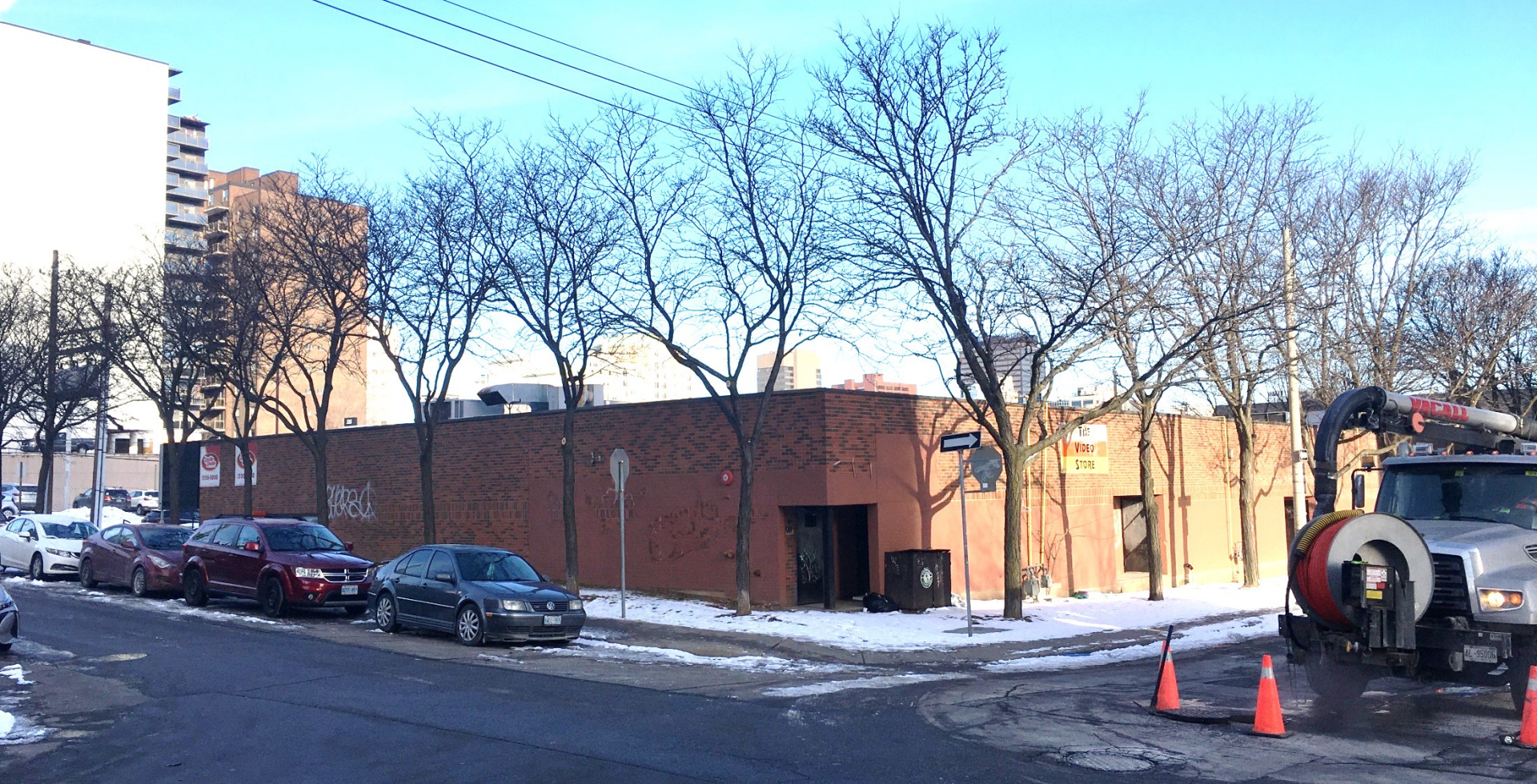
Subject property, as seen from the intersection of Catharine Street South and Forest Avenue looking northwest
