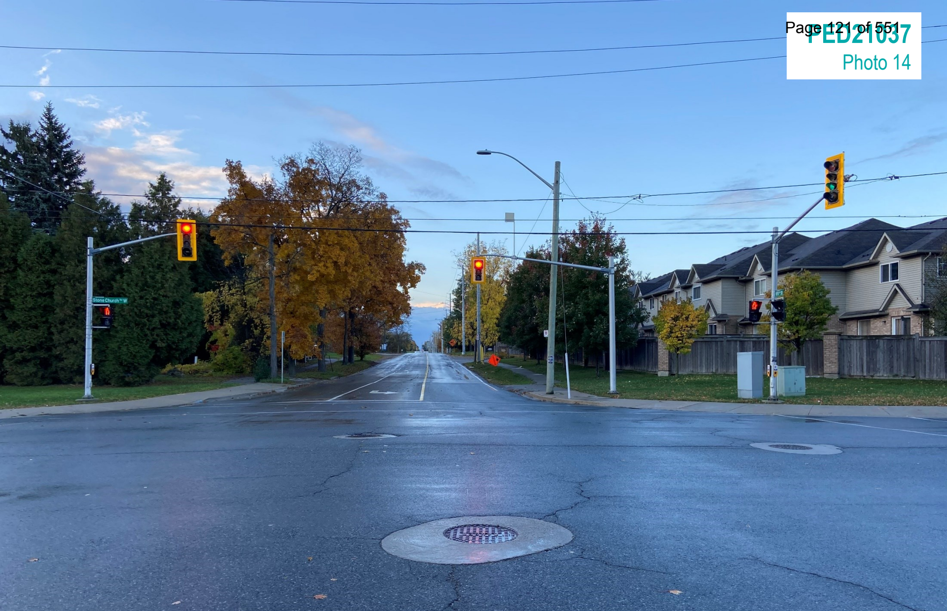
West 5 th Street (looking south)
