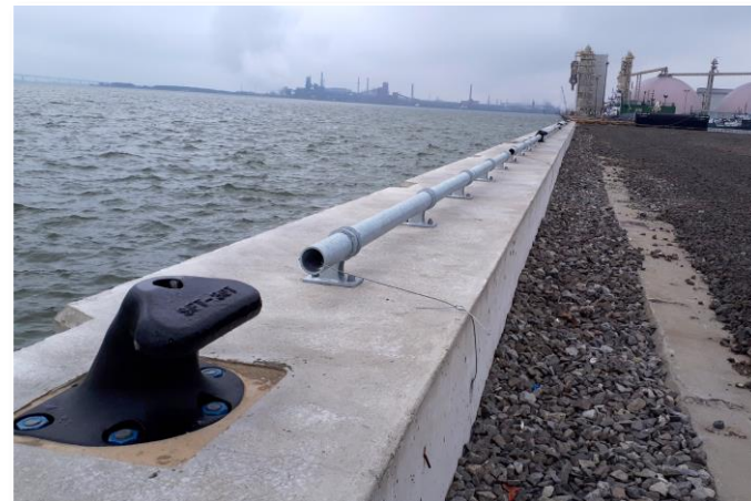
Waterfront Shore Wall Construction
