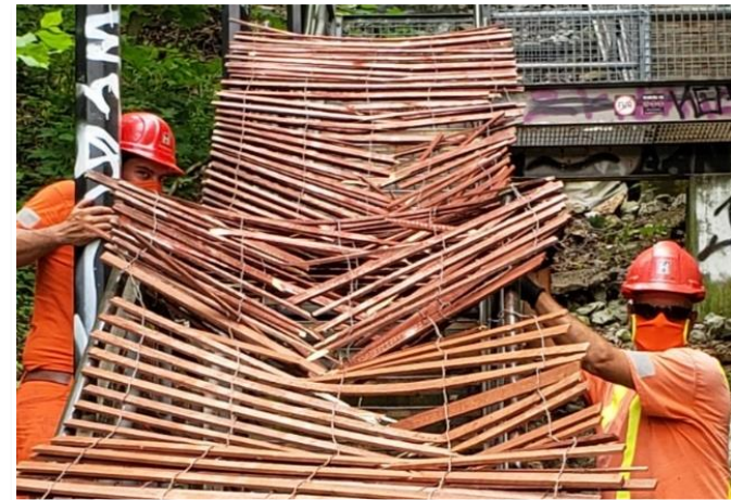
Barriers on the Escarpment Stairs
