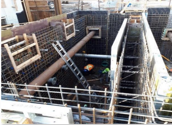
Pier 8 Wastewater Pumping Station
