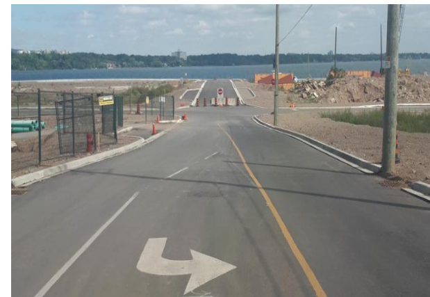
Pier 7 and 8 servicing
