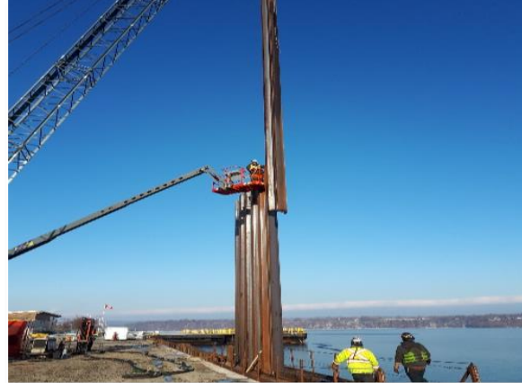
Pier 8 Shorewall Reconstruction
