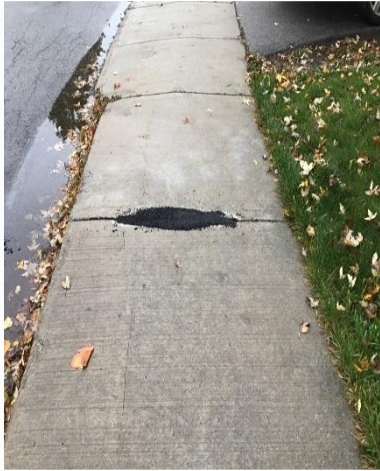
Asphalt Repair
