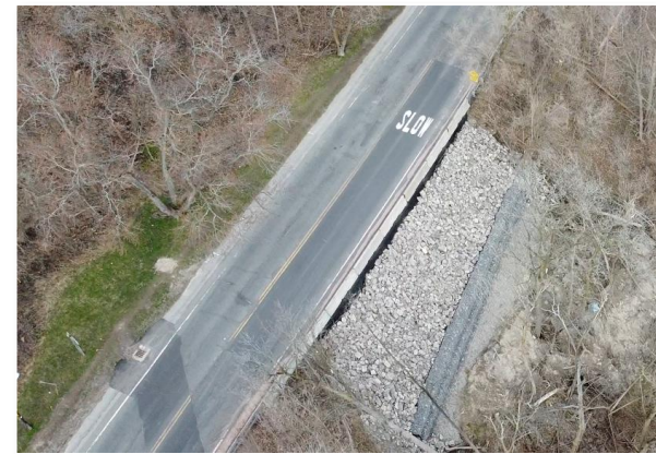
Hwy 8 Dundas Escarpment Repair
