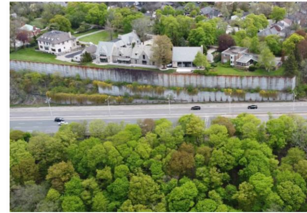
Claremont access bin walls
