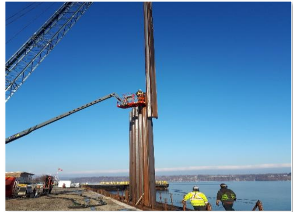
Pier 8 Shorewall Reconstruction
