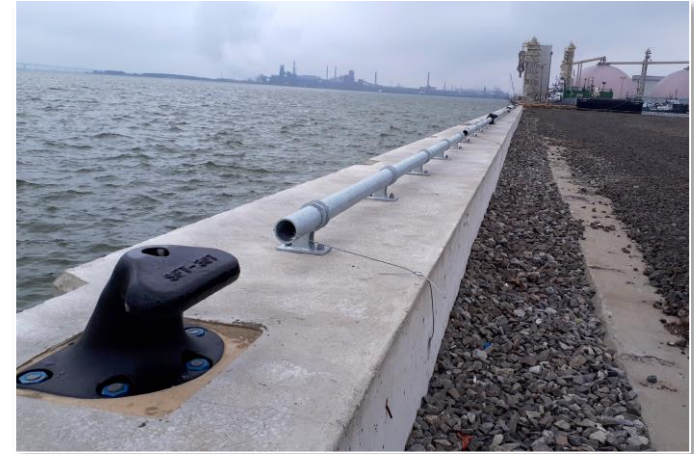
Waterfront Shore Wall Construction
