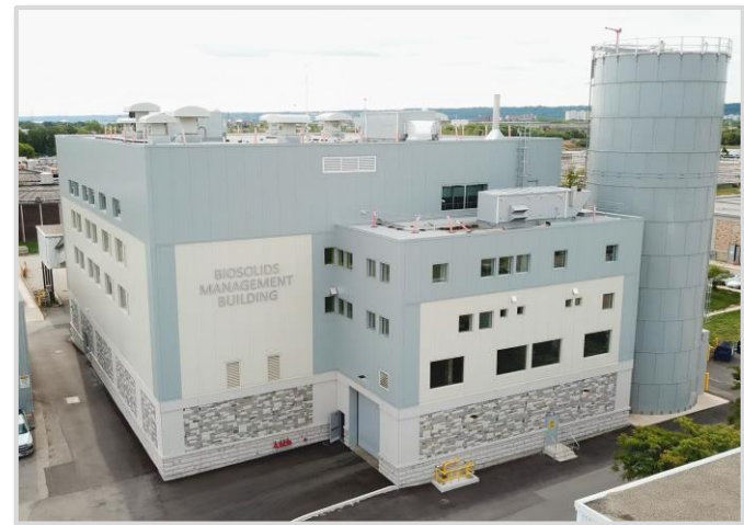
Biosolids Management Facility 16
