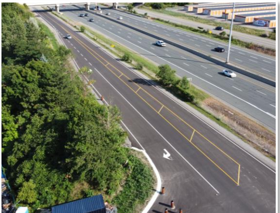
North Service Road
