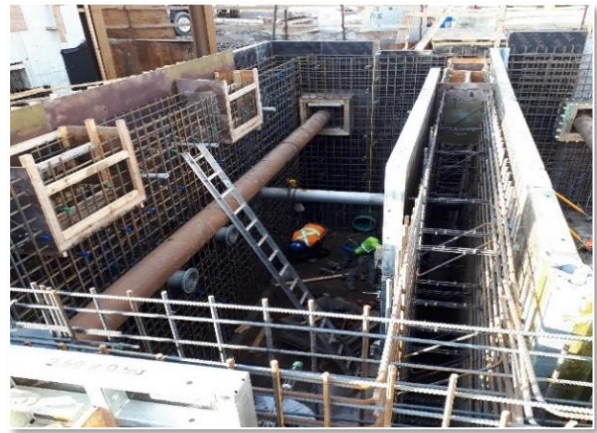
Pier 8 Wastewater Pumping Station
