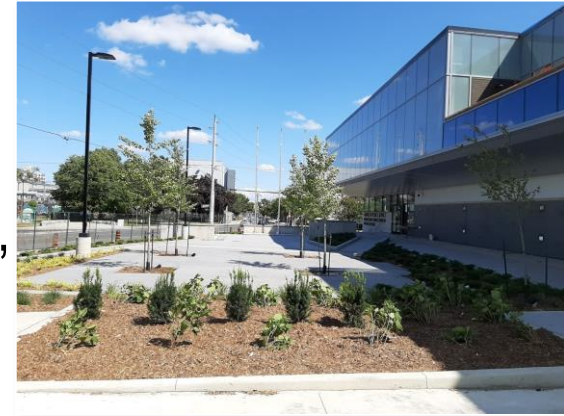
Police Forensics Building
