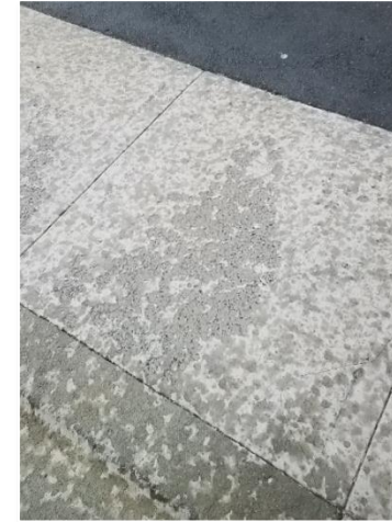
Concrete Spalling
