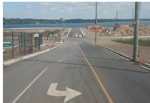
Pier 7 and 8 servicing
