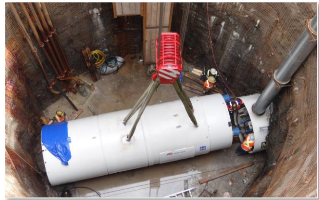
Upper Centennial Parkway Trunk Sewer Project
