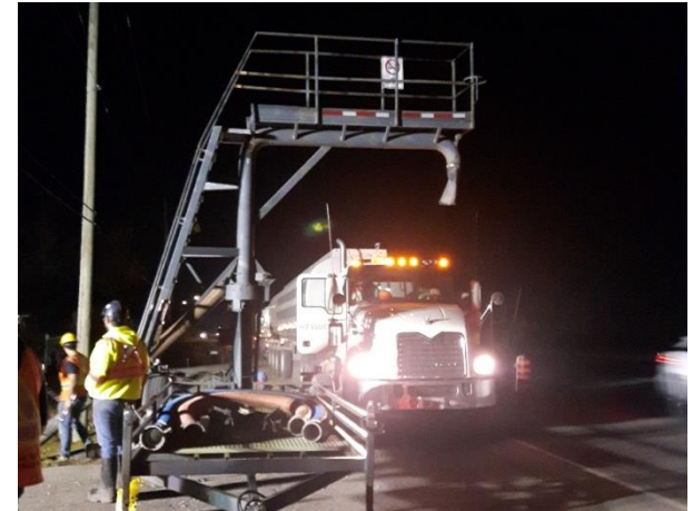
AEGD English church pumping station
