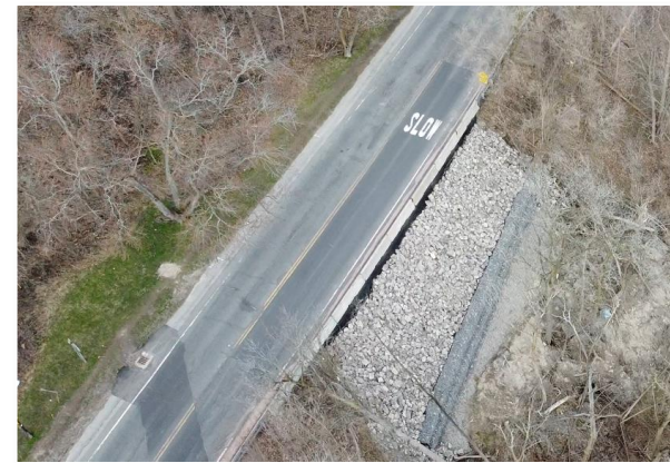
Hwy 8 Dundas Escarpment Repair
