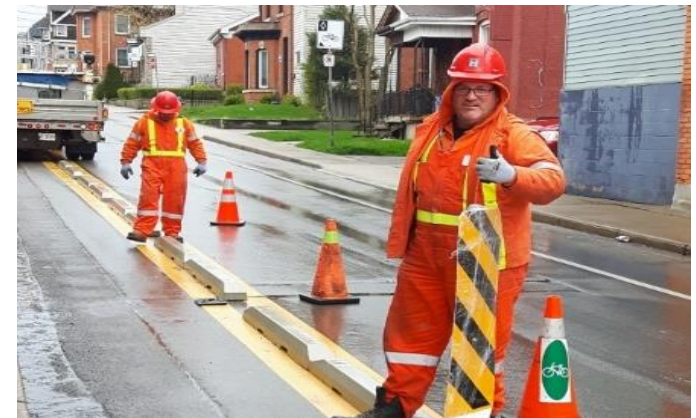
Concrete cycling curbs
