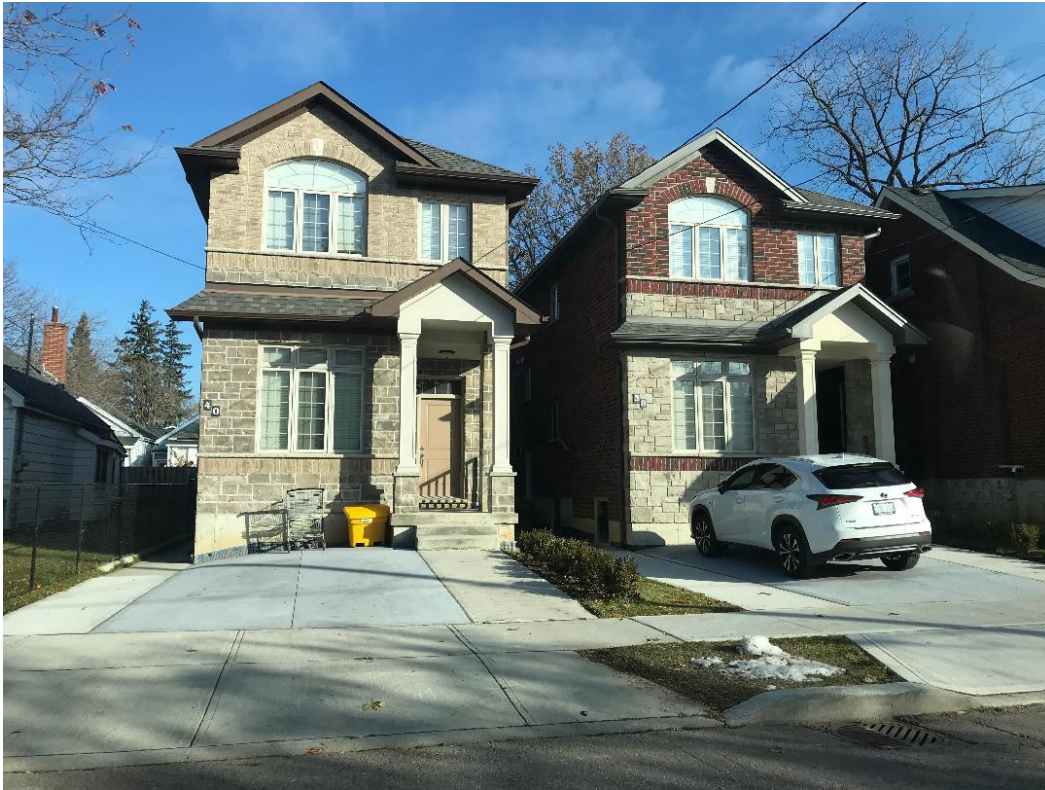
Figure 8 – New Dwellings Constructed at 38 and 40 Holmes Avenue
