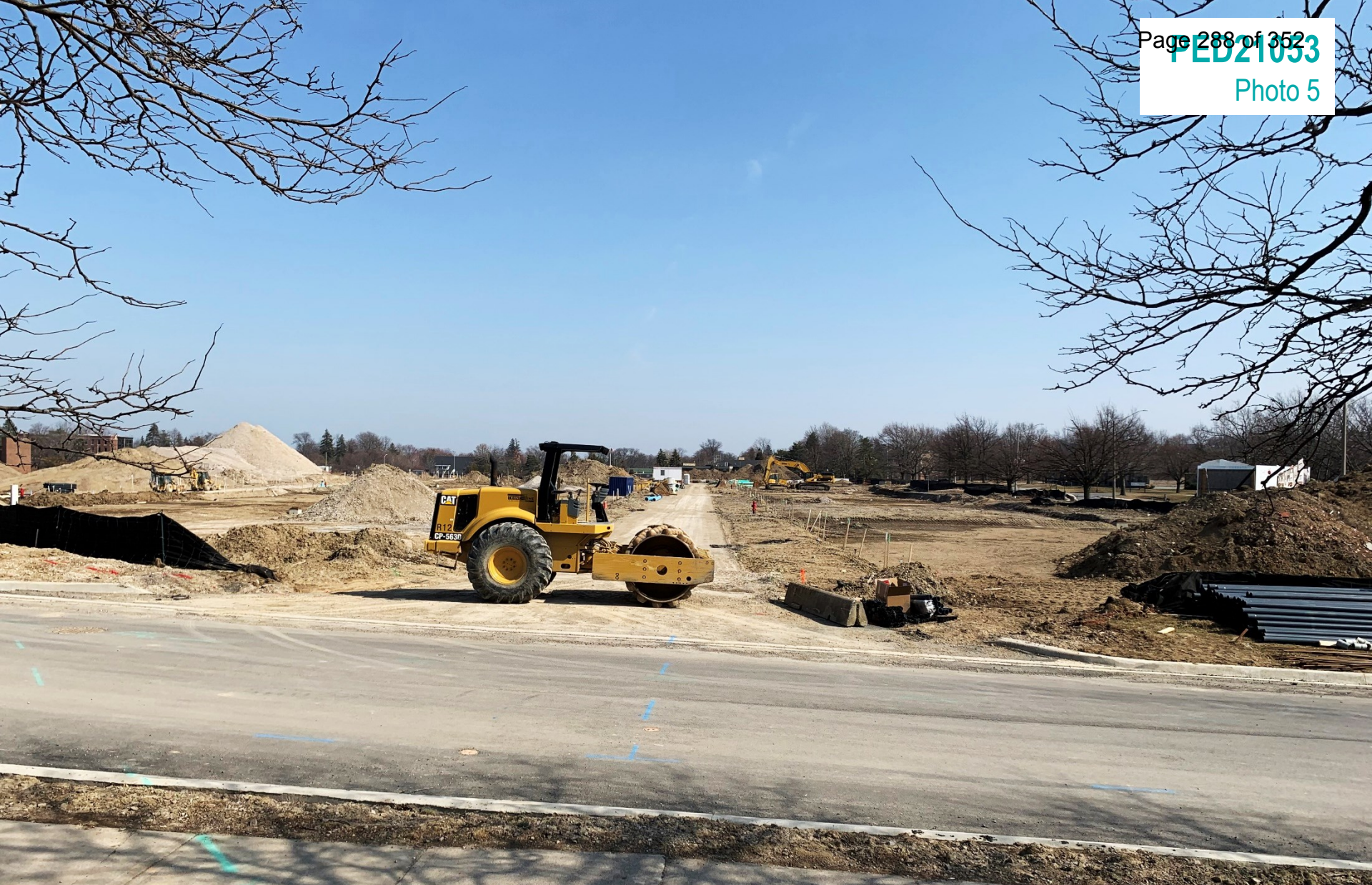
Phase 1 entrance to subject lands from the west
