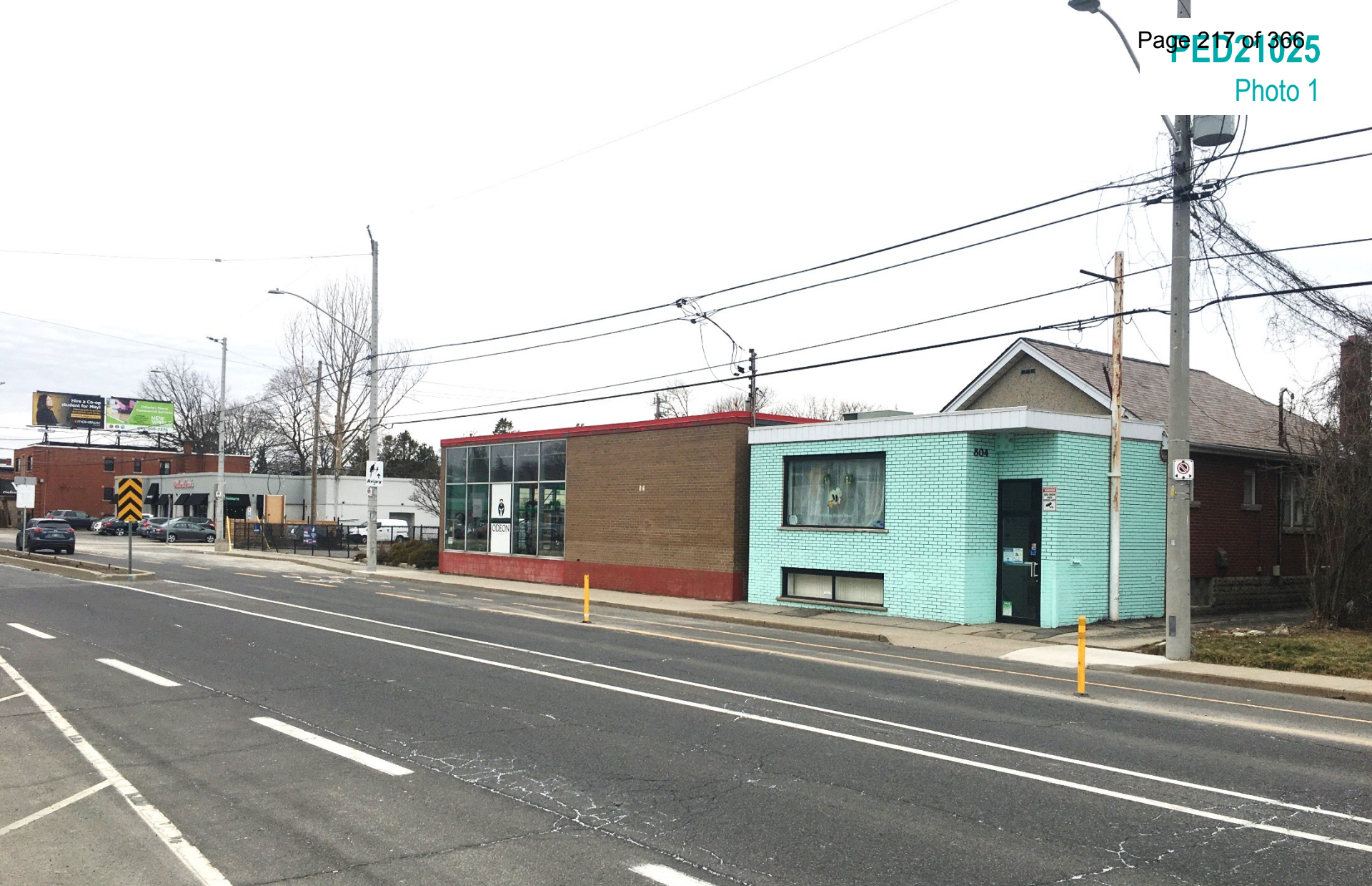
Subject property, as seen from King Street West looking northwest
