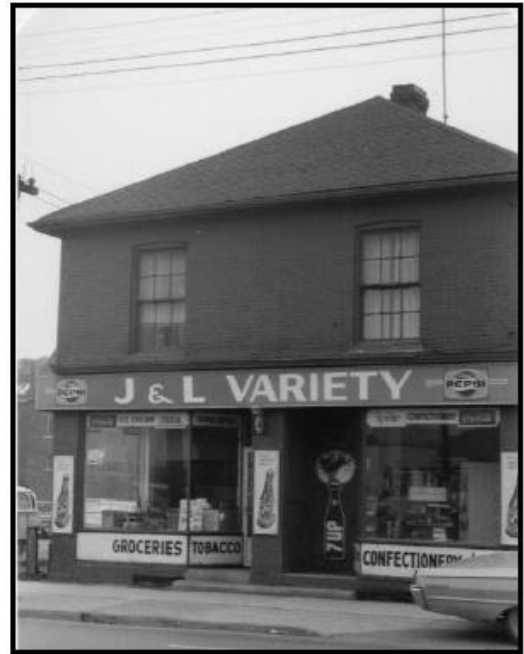
Figure 6: Intersection of Cannon and Cathcart Streets, showing front facade of 204 Cannon Street E; c.1973. (City of Hamilton Heritage Archives, ca. 1973).
