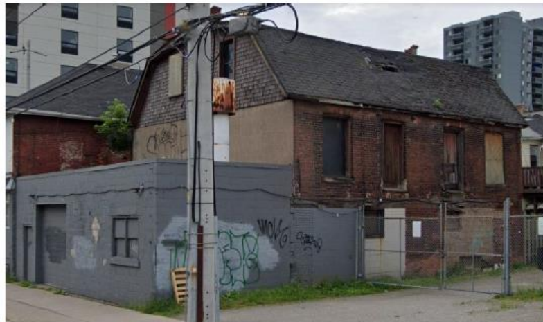
Figure 11: 202 Cannon Street; 19 th century; two floors and gambrel roof. One storey concrete block addition (c1960) in foreground. Source: Google Images
