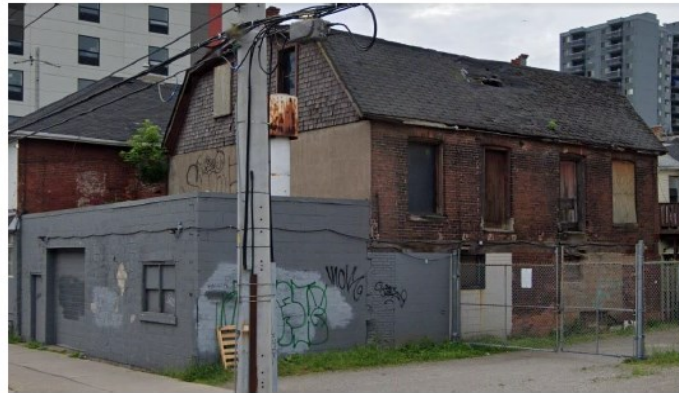
Figure 11: 202 Cannon Street; 19 th century; two floors and gambrel roof. One storey concrete block addition (c1960) in foreground. Source: Google Images
