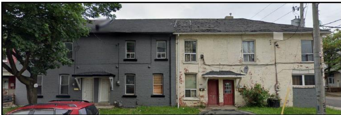
Figure 13: Facades of 79/81 Cathcart Street showing fire wall protruding above roof level between the units. The building at 202 Cannon Street (white building right) was originally 85 Cathcart Street. Source: Google Images.
