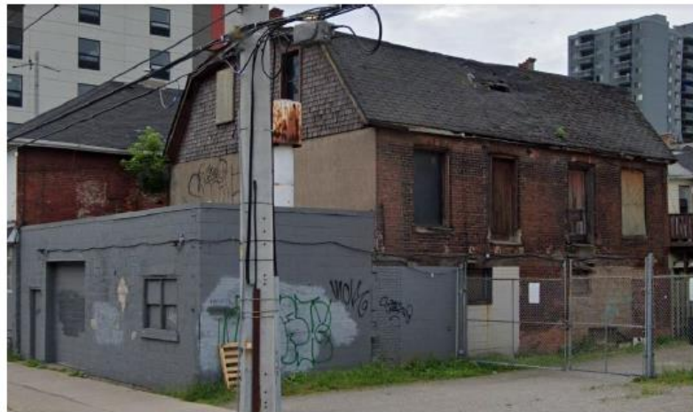
Figure 11: 202 Cannon Street; 19 th century; two floors and gambrel roof. One storey concrete block addition (c1960) in foreground. Source: Google Images
