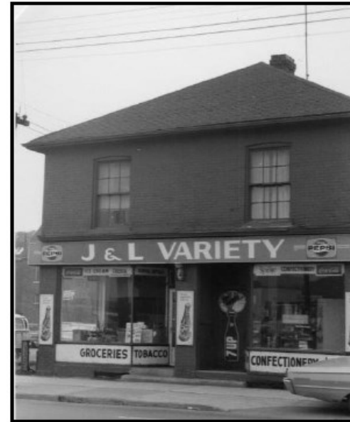
Figure 6: Intersection of Cannon and Cathcart Streets, showing front facade of 204 Cannon Street E; c.1973. (City of Hamilton Heritage Archives, ca. 1973).
