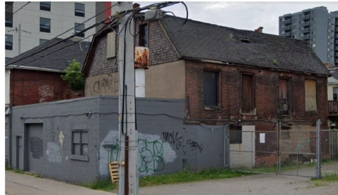
Figure 11: 202 Cannon Street; 19 th century; two floors and gambrel roof. One storey concrete block addition (c1960) in foreground. Source: Google Images
