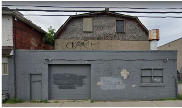
Figure 10: The foreground is a c.1960s one-storey concrete block entrance at 202 (formerly 200) Cannon Street. In the background is a 19 th century, two storey, gambrel roof abandoned "industrial" building. Source: Google Images.
