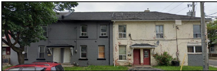
Figure 13: Facades of 79/81 Cathcart Street showing fire wall protruding above roof level between the units. The building at 202 Cannon Street (white building right) was originally 85 Cathcart Street. Source: Google Images.
