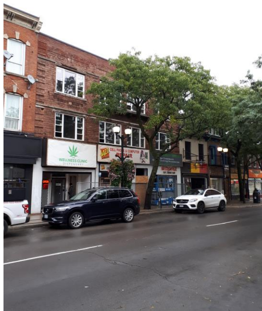
233-237 King Street East (Before Renovation) Source: City of Hamilton Building Division
