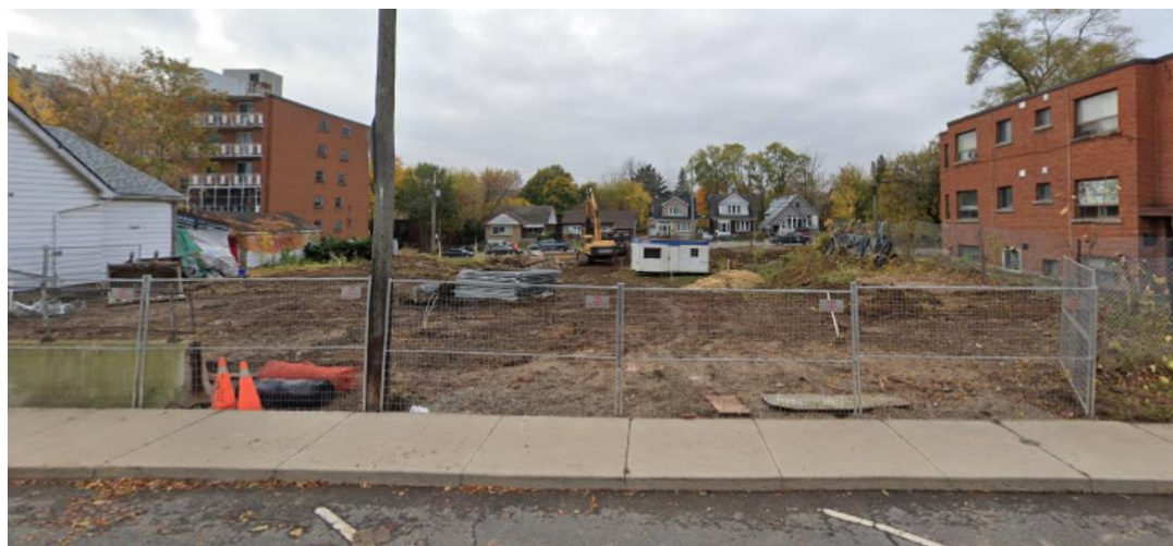
Existing Conditions – 801 and 803 King Street West and 80, 86 and 90 Carling Street, Hamilton (Source: maps.google.ca – Oct. 2020)
