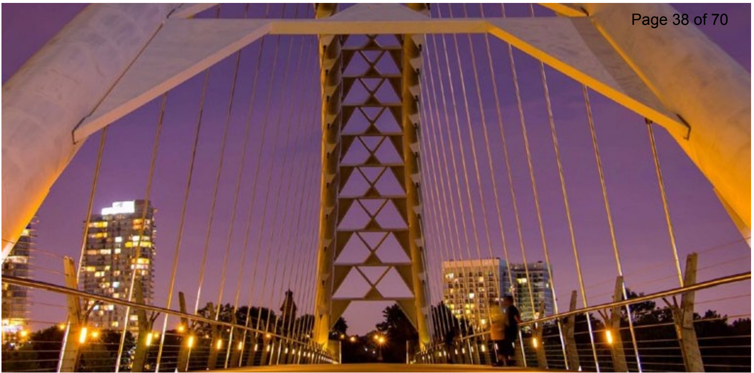
Humber Bay Arch Bridge, Etobicoke | Photo Credit: alyssablack, Flickr
