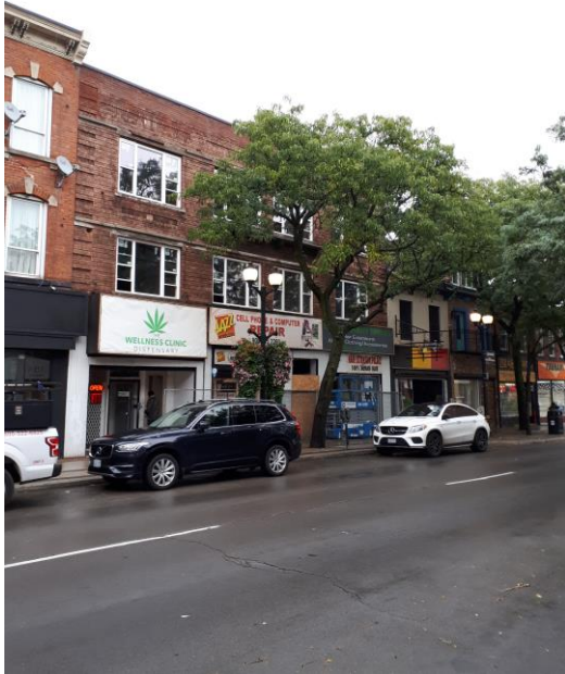
233-237 King Street East (Before Renovation) Source: City of Hamilton Building Division
