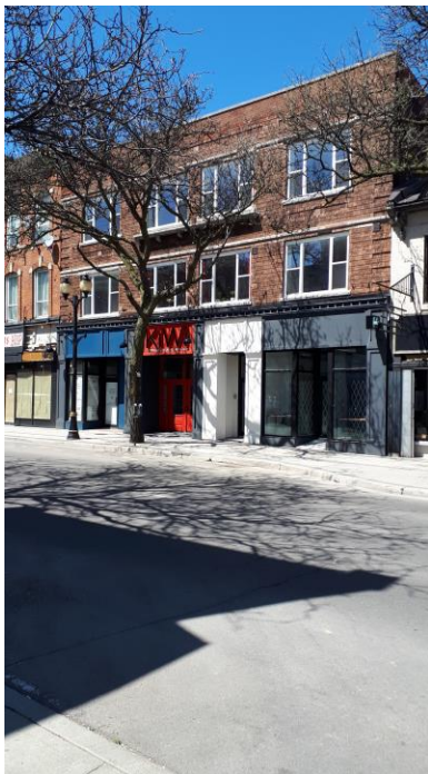
233-237 King Street East (Post Renovation) Source: City of Hamilton Building Division
