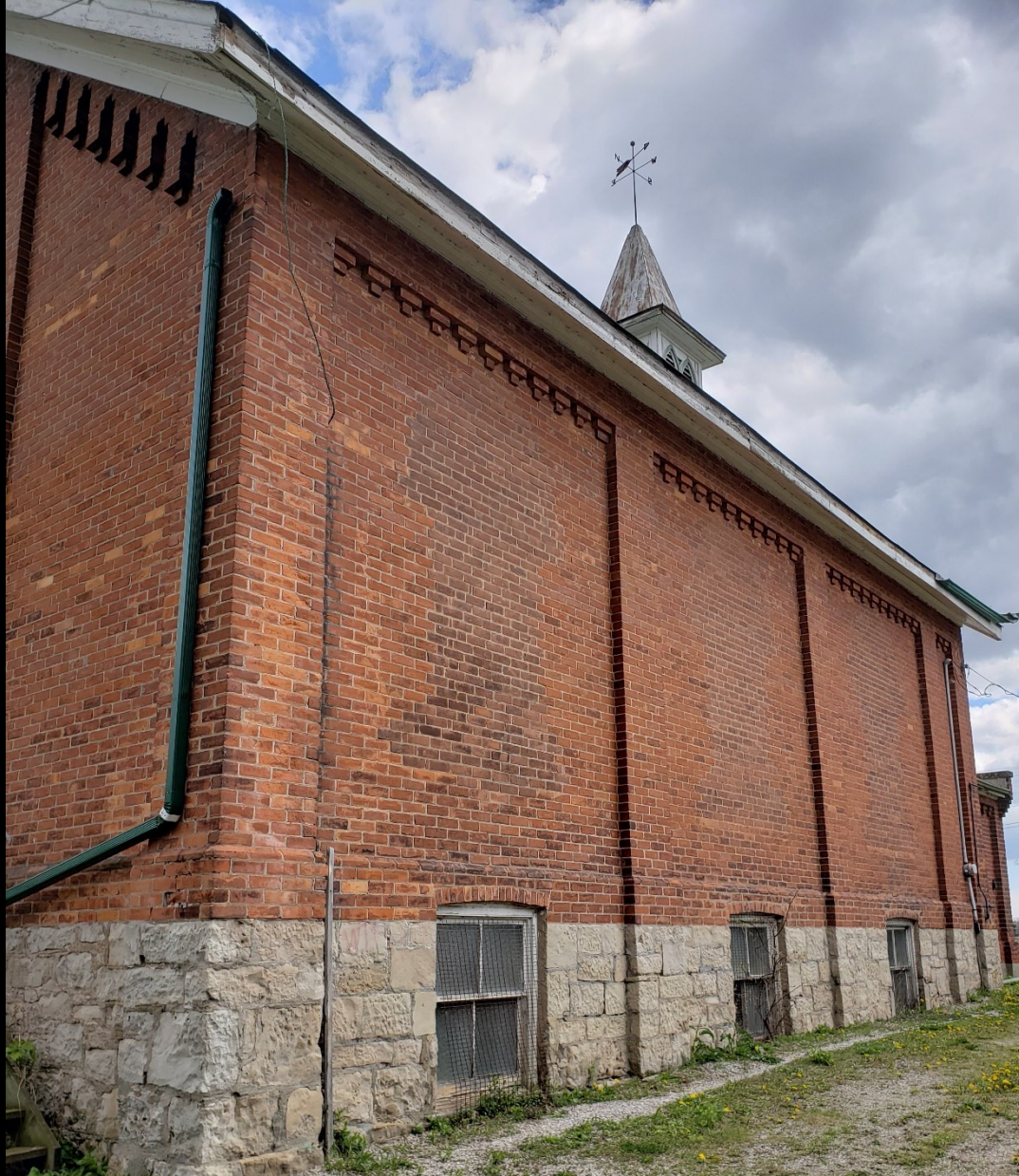
Corner of Market Street and Queen Street North looking east
