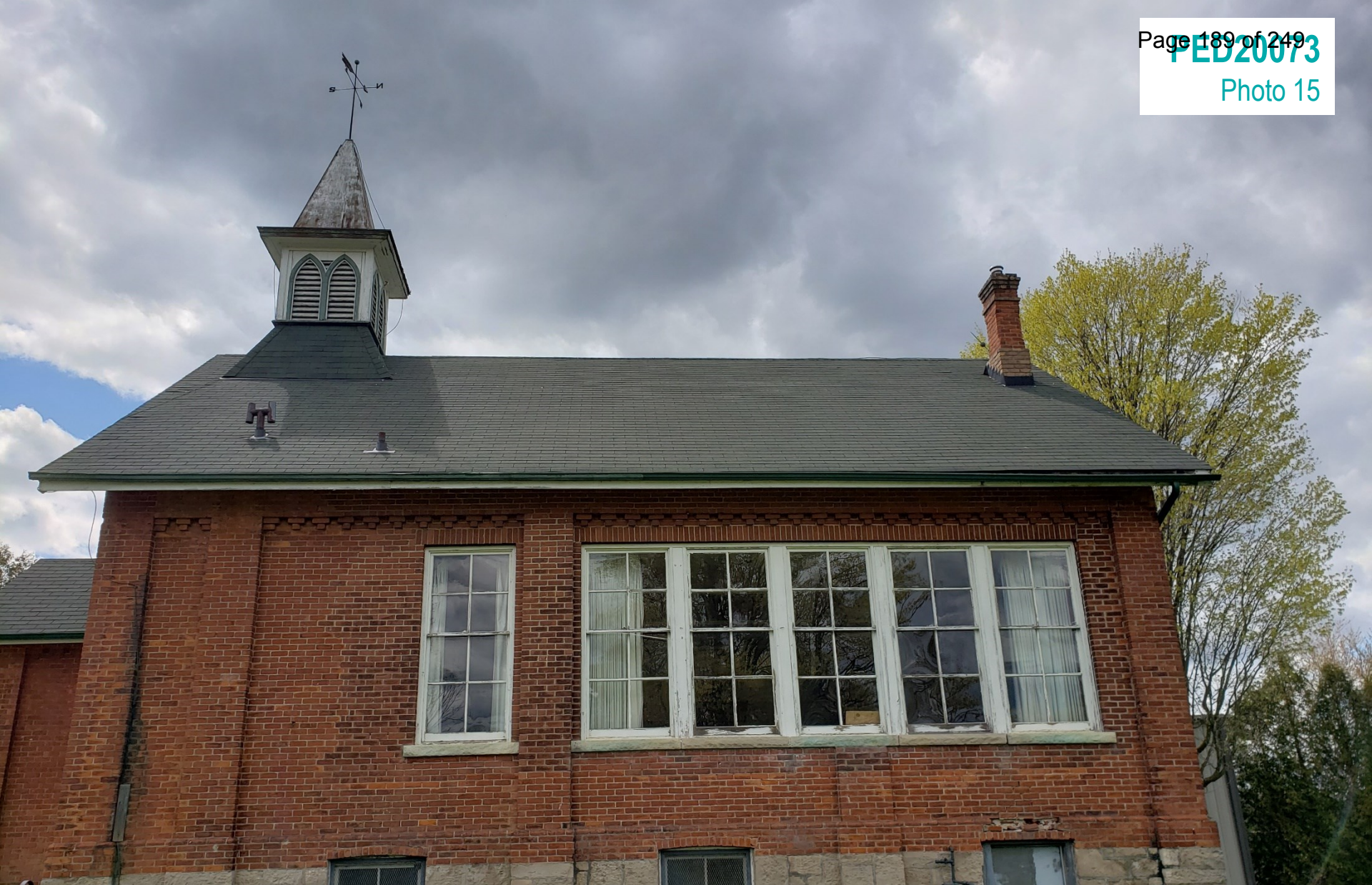
Roof, Chimney, Belfry and east windows
