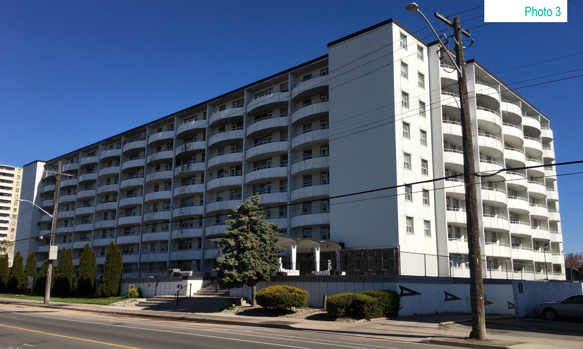
Existing development to the north, as seen from Melvin Avenue looking north
