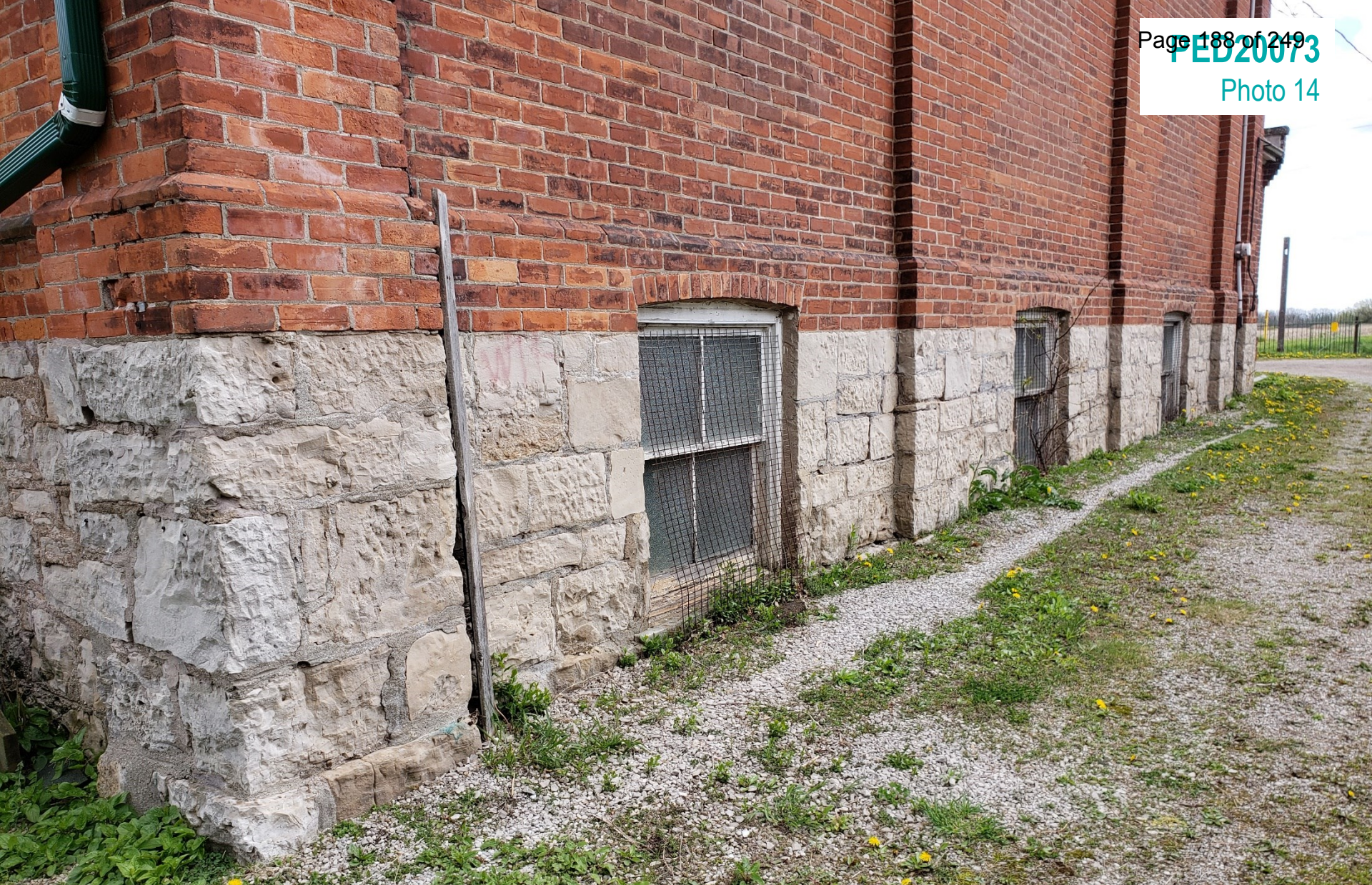
Stone Foundation and west windows
