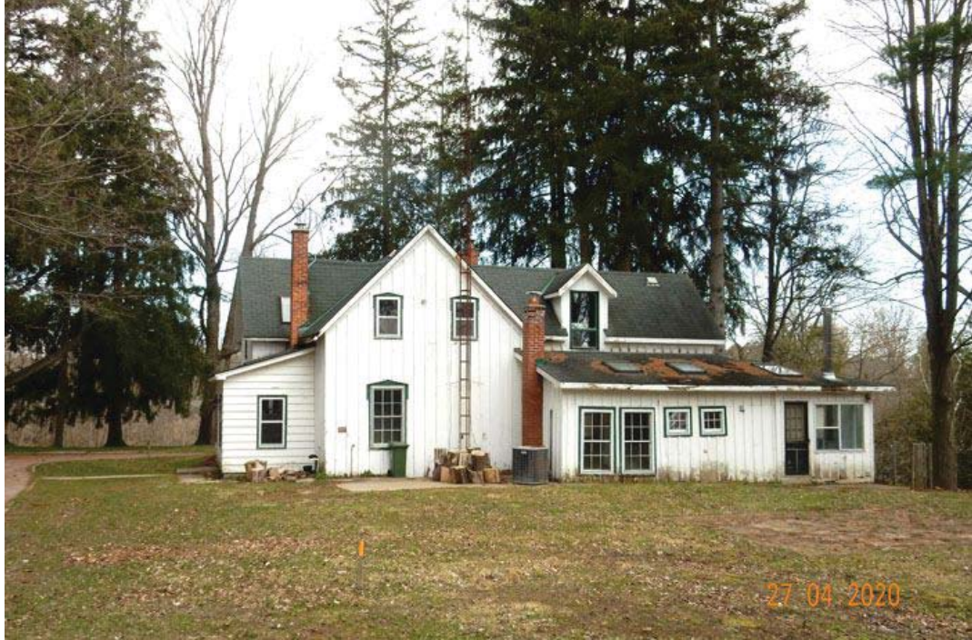
Figure 2: Rear Elevation, 1389 Progreston Road
