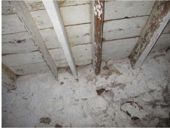
Randomly sized and spaced circular-sawn floor joists
