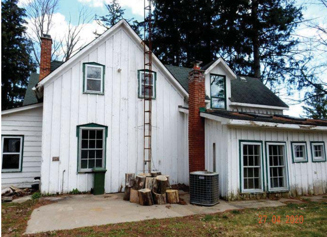
Figure 4: Rear Elevation, 1389 Progreston Road
