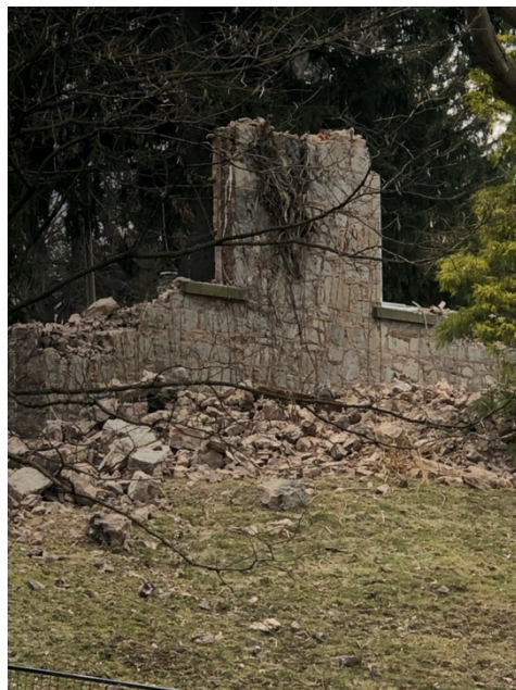
THE CITY DEMOLITION PERMIT WAS ACTED UPON IMMEDIATELY
