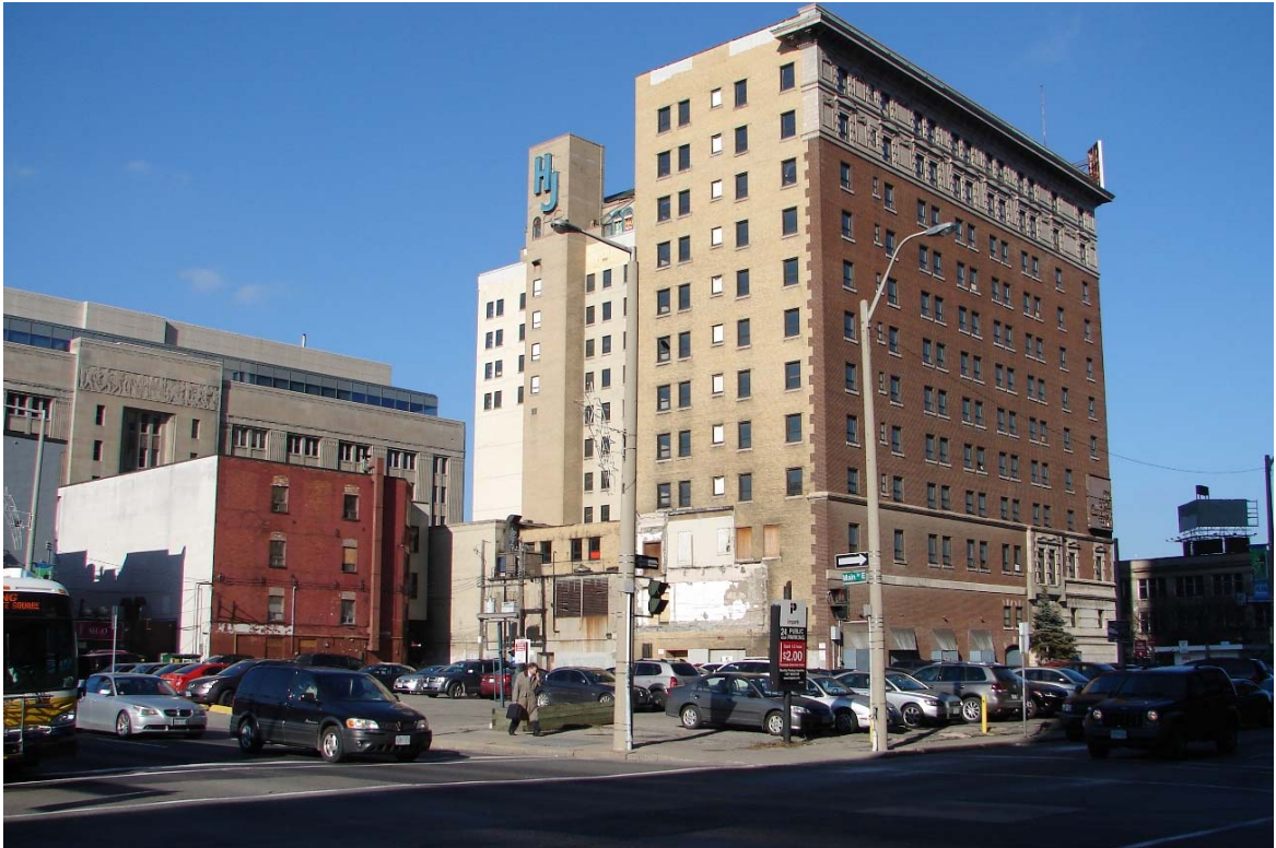
Fig. 37 Corner view of the south (rear) and east elevations from the east side of Catharine Street South (note Dominion Public Building on west side of John Street South)
