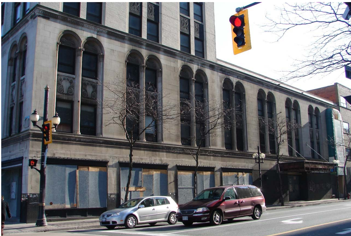
Fig. 69 Top: West elevation's tower shaft; Bottom: West elevation's base
