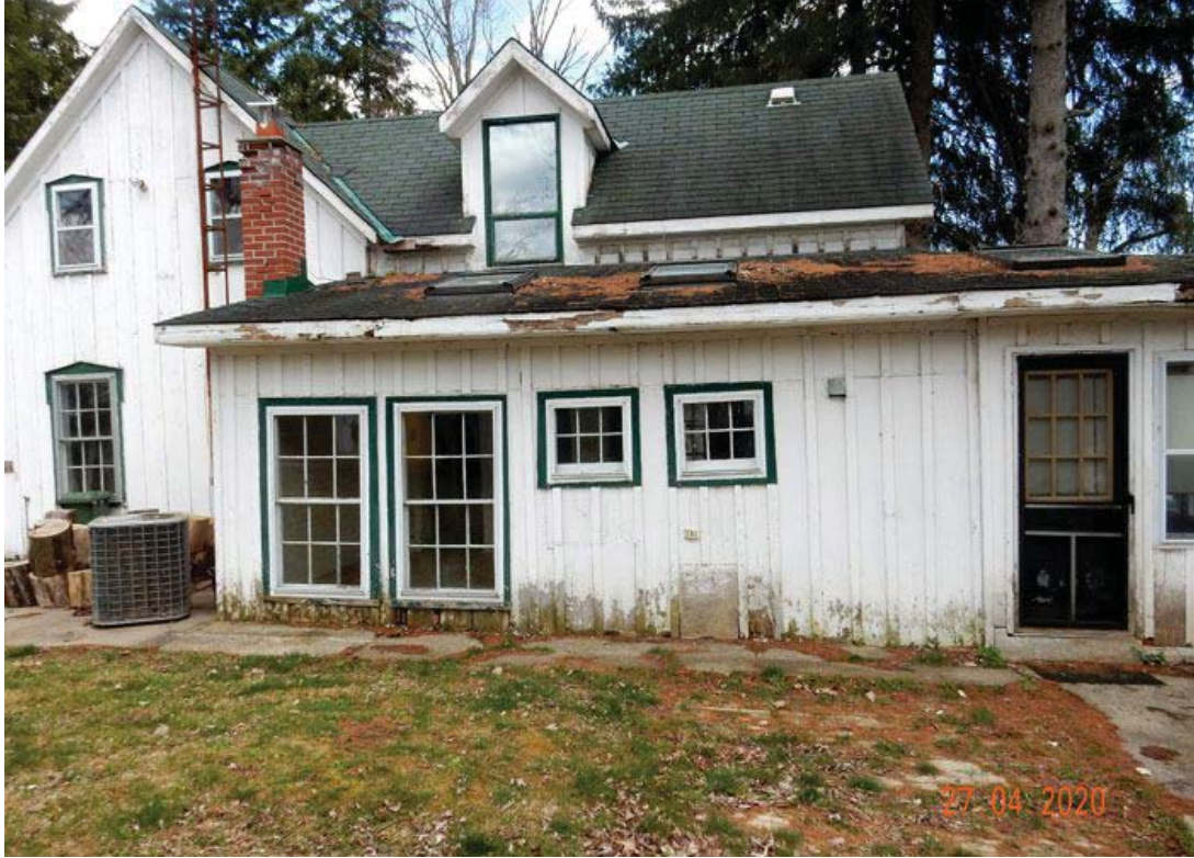
Figure 6: Rear Elevation, 1389 Progreston Road
