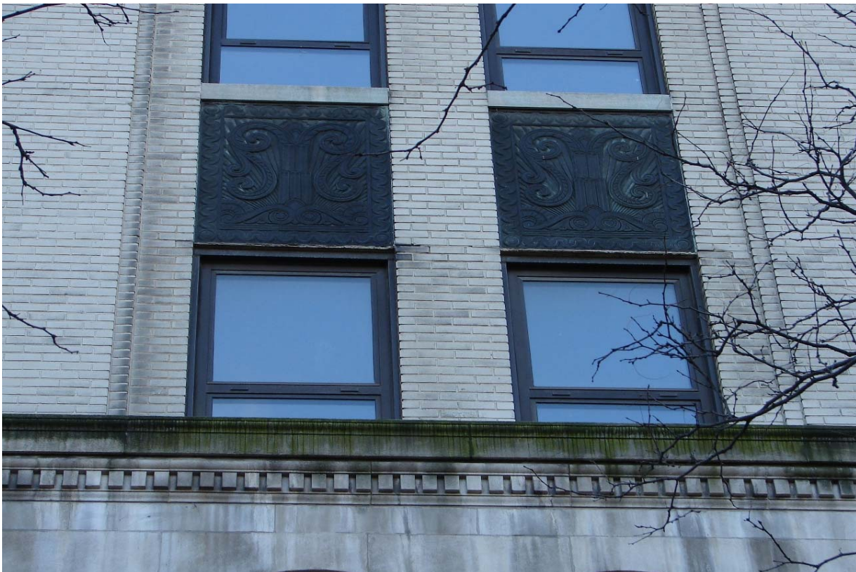
Fig. 57 Windows in shaft
