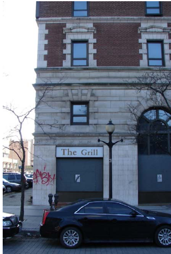
Fig. 43 East end of front facade's base
