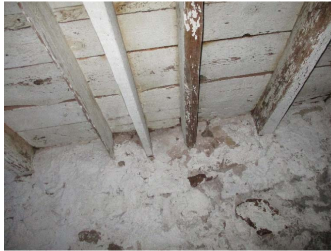
Randomly sized and spaced circular-sawn floor joists
