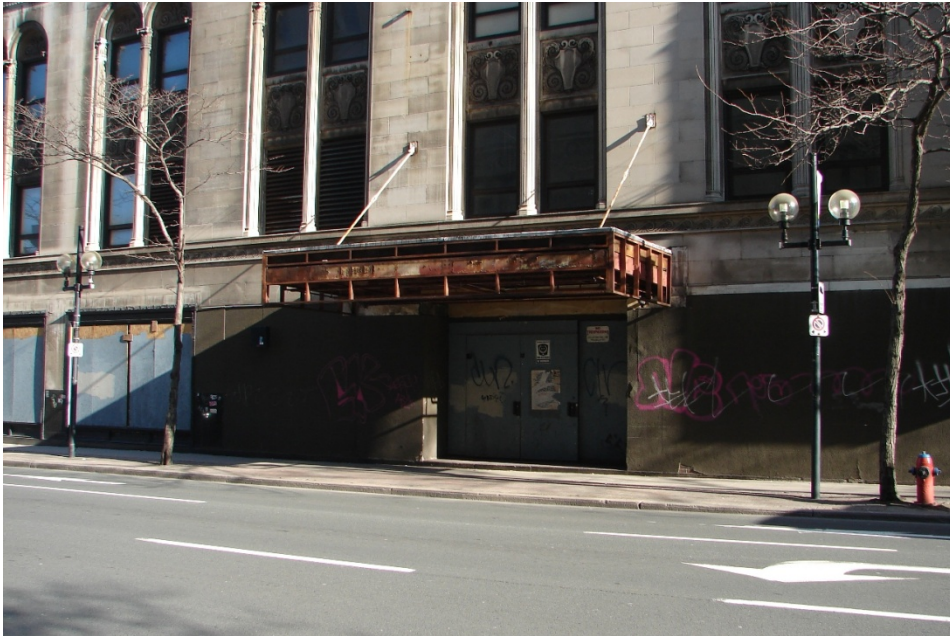
Fig. 70 Marquee frame over John Street South entrance
