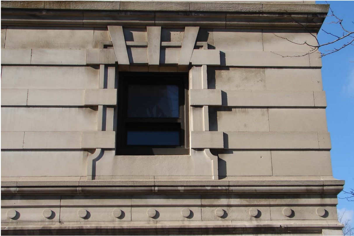
Fig. 63 Stone window surrounds
