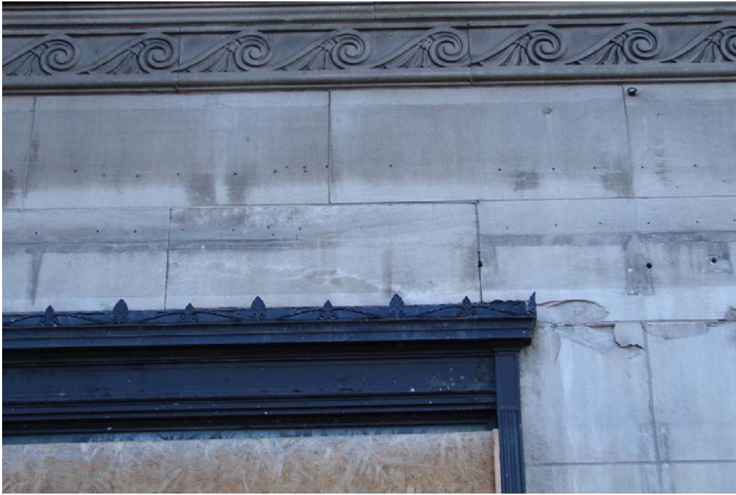
Fig. 54 Detail of ground-floor stringcourse in Art Deco wave pattern
