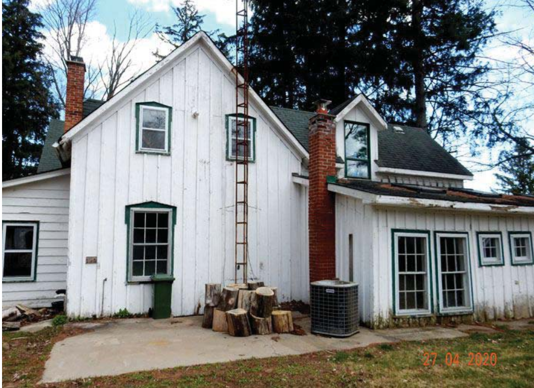
Figure 4: Rear Elevation, 1389 Progreston Road
