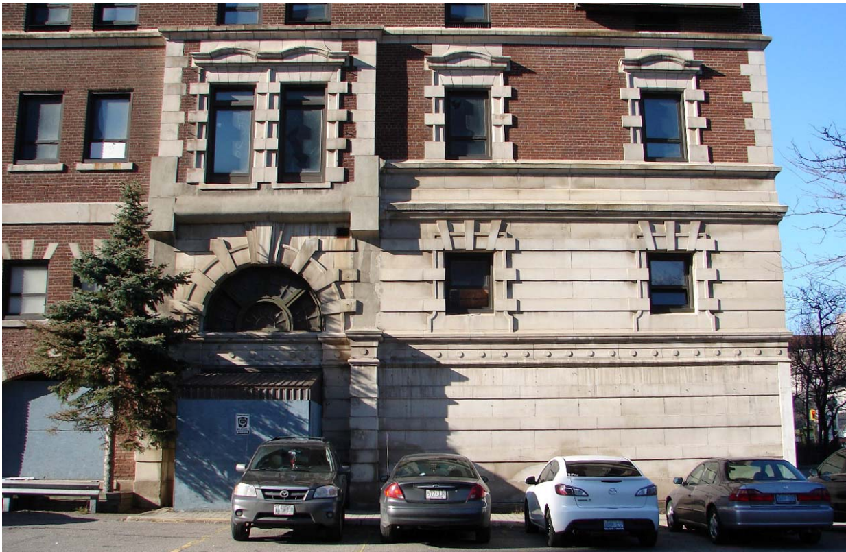
Fig. 61 Northernmost three bays of the east elevation's base
