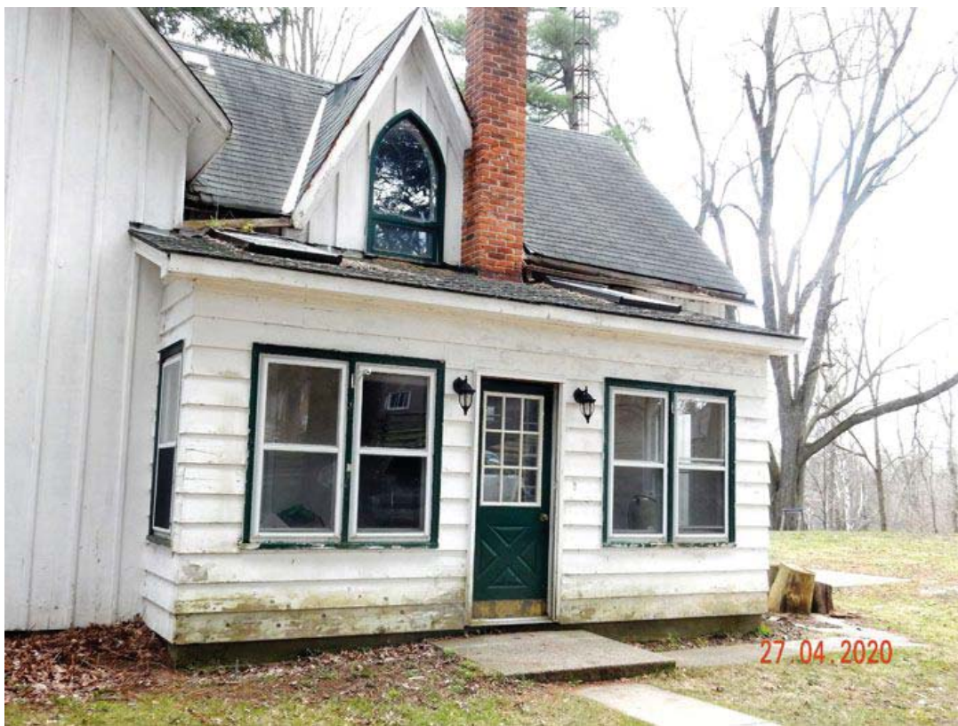
Figure 5: North Elevation, 1389 Progreston Road
