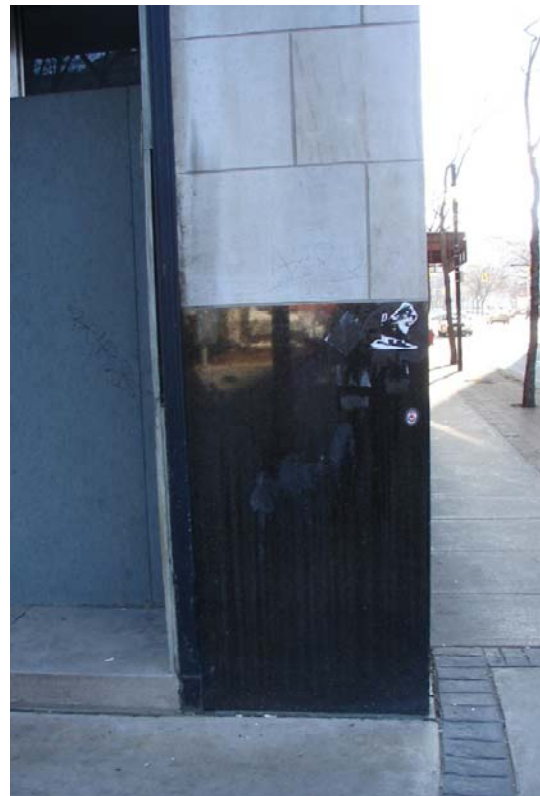
Fig. 51 Brown polished granite foundation veneer
