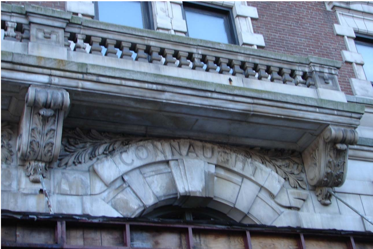
Fig. 41 Detail of stone balustrade of balcony above the main entrance
