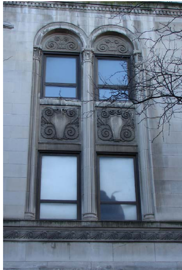
Fig. 55 Pair of round-arched windows lighting mezzanine and second floors
