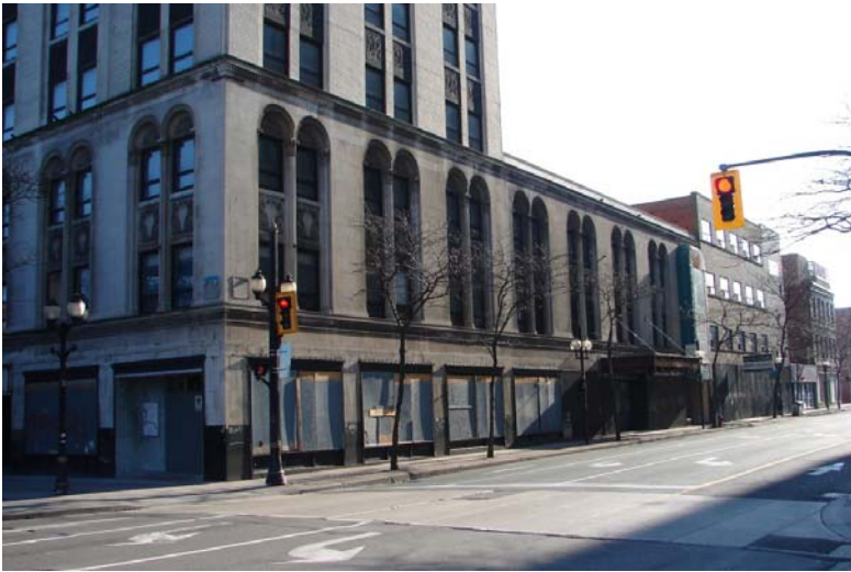
Fig. 34 East side of John Street South, looking south
