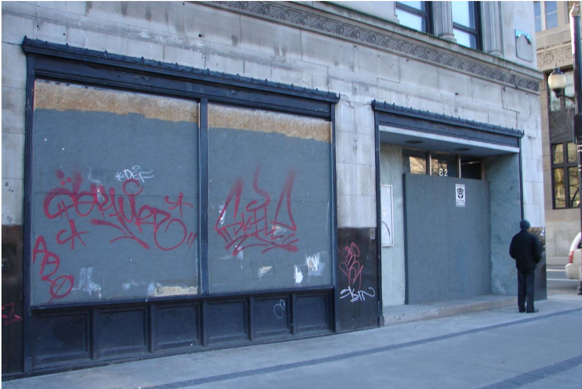
Fig. 50 Detail of ground floor in Art Deco addition
