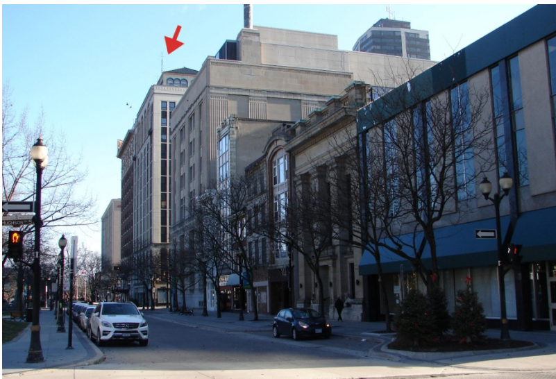
Fig. 32 South side of King Street East, looking east from Hughson Street (arrow points to rooftop pavilion)
