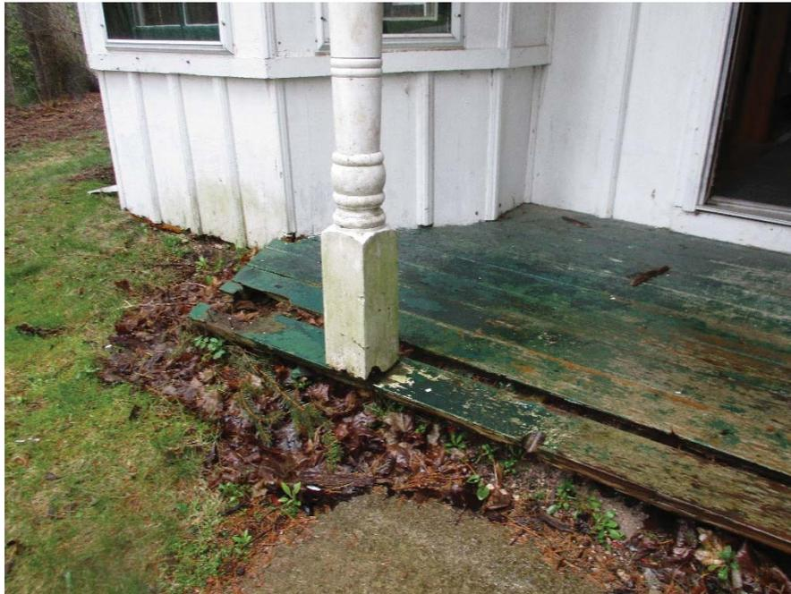
Front porch with rotting modern post and failing floor structure
