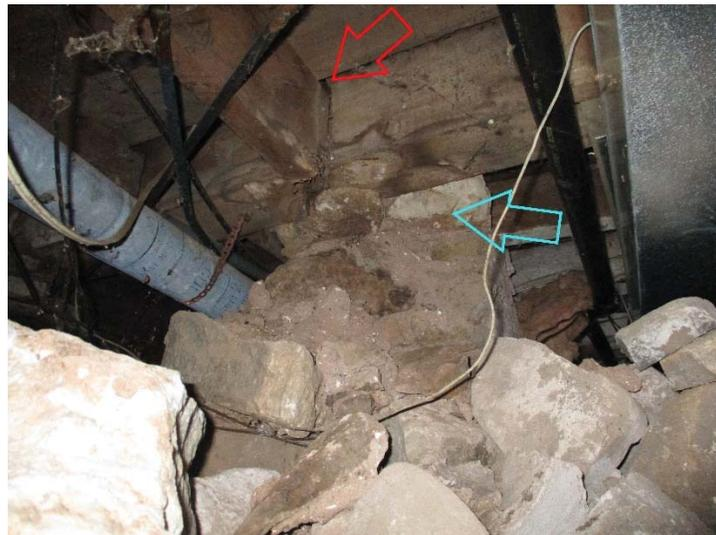
Dropped joist, sawn timber sill plate, altered foundation, missing support
