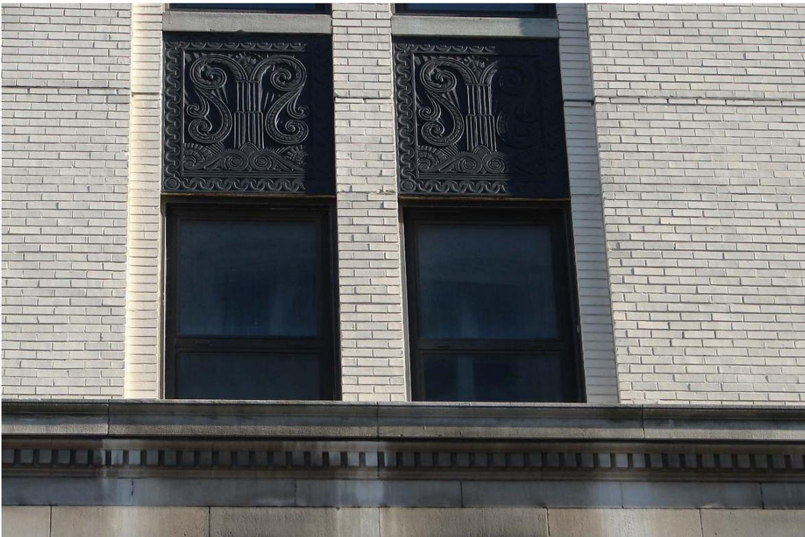
Fig. 75 Windows in west elevation's tower shaft (note bronze spandrels in the Art Deco style)
