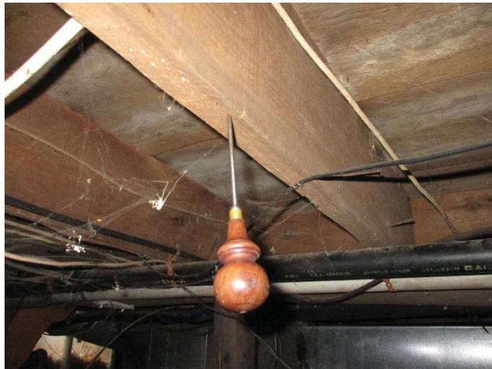
Deteriorated floor joist, awl inserted >2"
