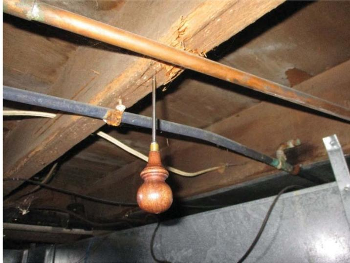
Deteriorated floor joist, awl inserted >2"
