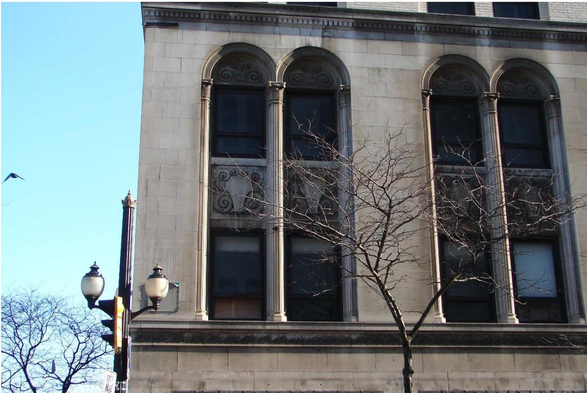
Fig. 74 Window pairs on mezzanine and second floors of west elevation's base (note also dentils in cornice above)
