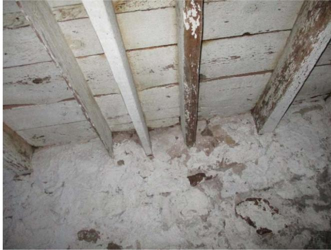
Randomly sized and spaced circular-sawn floor joists
