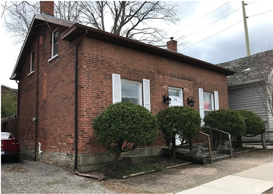
A 1½ storey brick cottage at 198 Hatt Street, with a symmetrical façade, Flemish bond brickwork and returned roof eaves.
