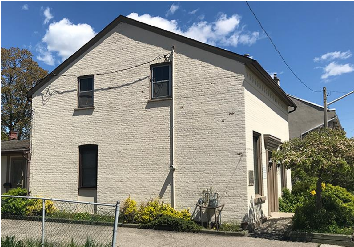
West façade showing the upper storey windows for second floor bedrooms, the converted doorway and the common bond brickwork of the side and rear walls, with one row of headers for every five rows of stretchers. Photo credit: Ann Gillespie, May 2021
