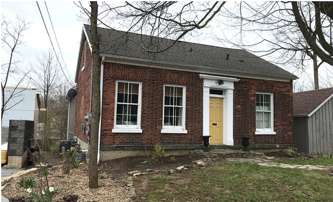
1½ storey brick masonry cottage at 320 MacNab Street. Features an asymmetrical façade with three windows and a more elaborate classical doorway with pillars and an entablature. Similarly to 215 King Street West, the bricks are laid with a Flemish bond.
