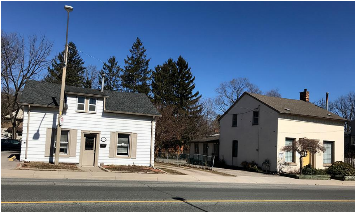
1½ storey cottages at 219 and 215 King Street West, just west of Market Street. Photo credit: Ann Gillespie, March 2021
