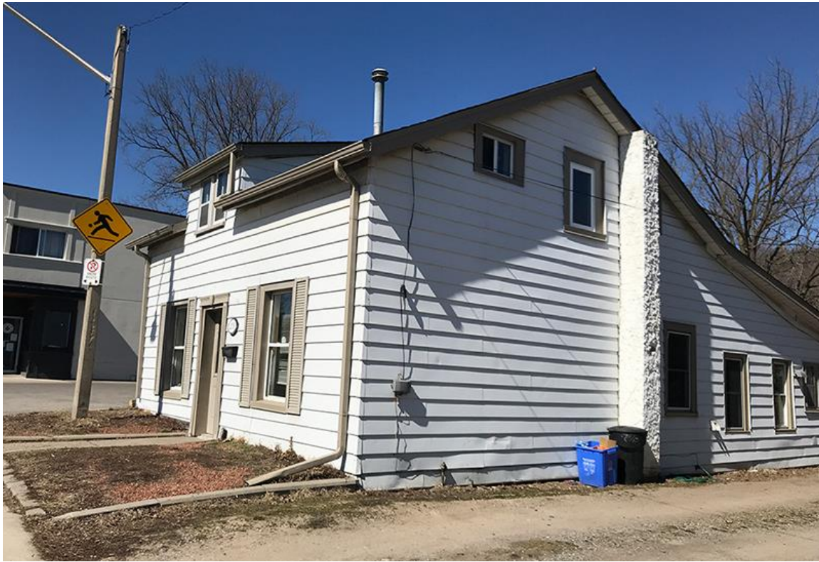
Shows the rear addition on the east side, the lowered brick chimney covered with rough stucco and an added horizontal sliding window on the second floor. March 2021
