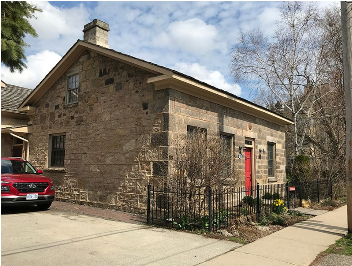
Front (south) and west facades showing the end chimney against the west wall. Also shows the large corner quoin blocks and medium-pitched side-gabled roof with returned eaves. All window and door sills and lintels are cut stone. The reproduction windows feature the original configuration of six-over-six paned sashes.
