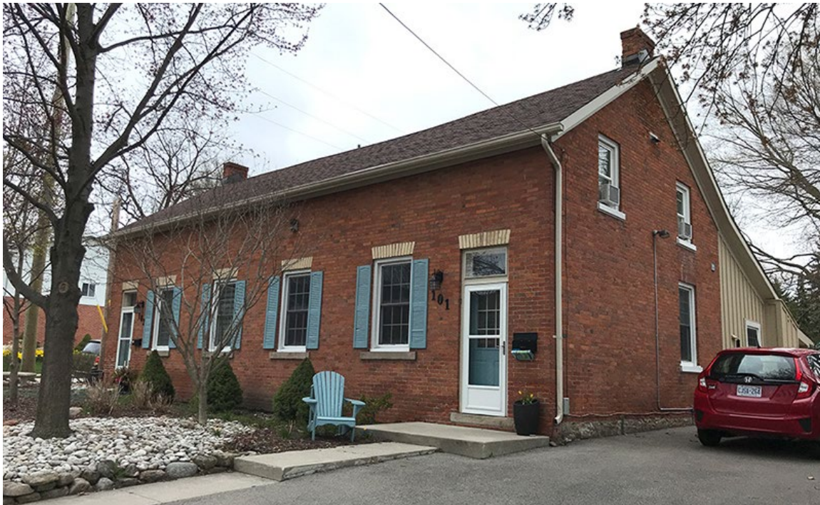
A more unusual semi-detached 1½ brick masonry storey cottage at 101 to 103 Park Street with a tall symmetrical façade and end doorways. Features flat voussoir arch window and doorway lintels in a contrasting yellow brick and stone sills. I have two more semi-detached examples to add here.
