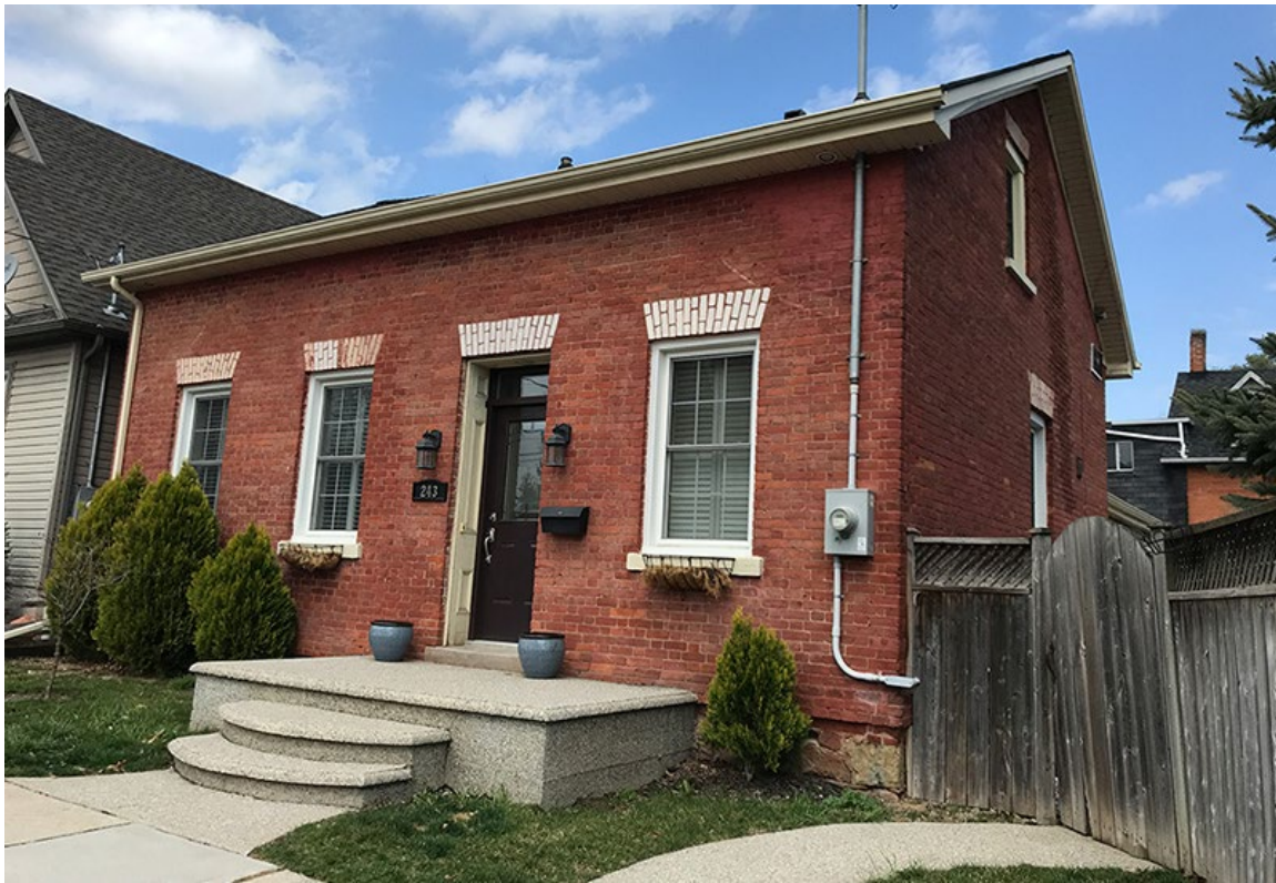
1½ brick masonry cottage at 243 Hatt Street, which features an asymmetrical façade with three windows and a recessed doorway. Window and door sills are made of cut stone; lintels are flat voussoir arches in a contrasting yellow brick. Another example of bricks laid with a Flemish bond.
