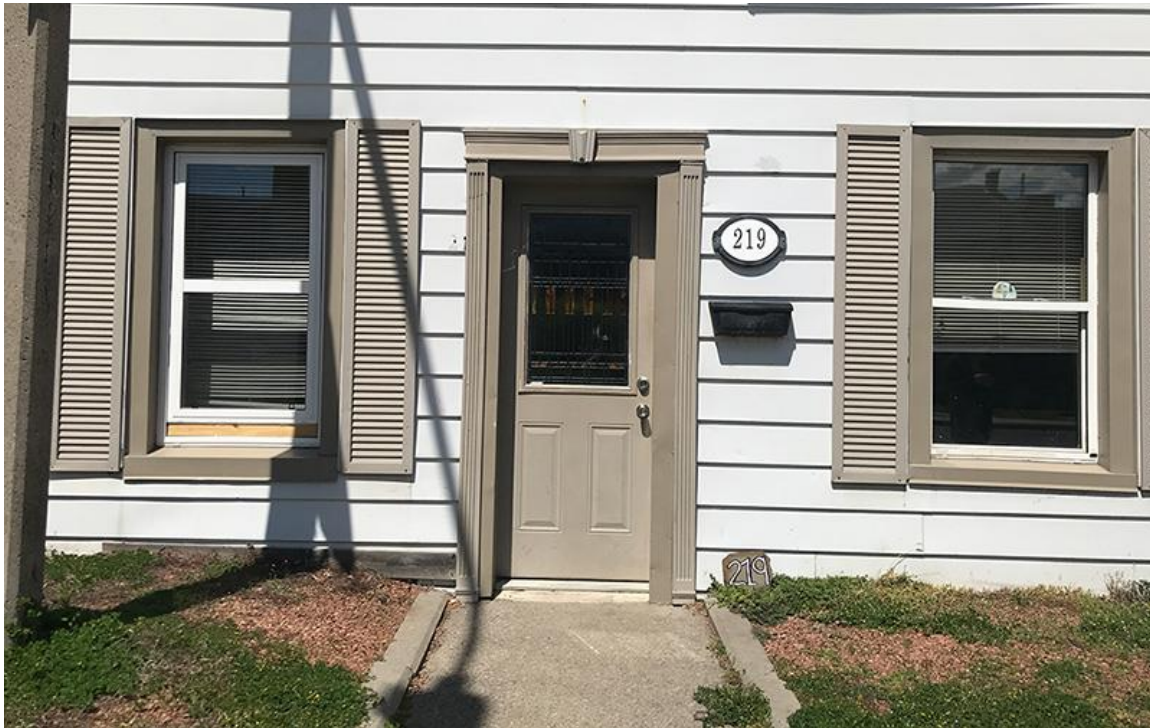
Close-up view of the front doorway and two first storey windows showing the aluminum cladding of the original wood door and window surrounds and a replacement metal door. May 2021
