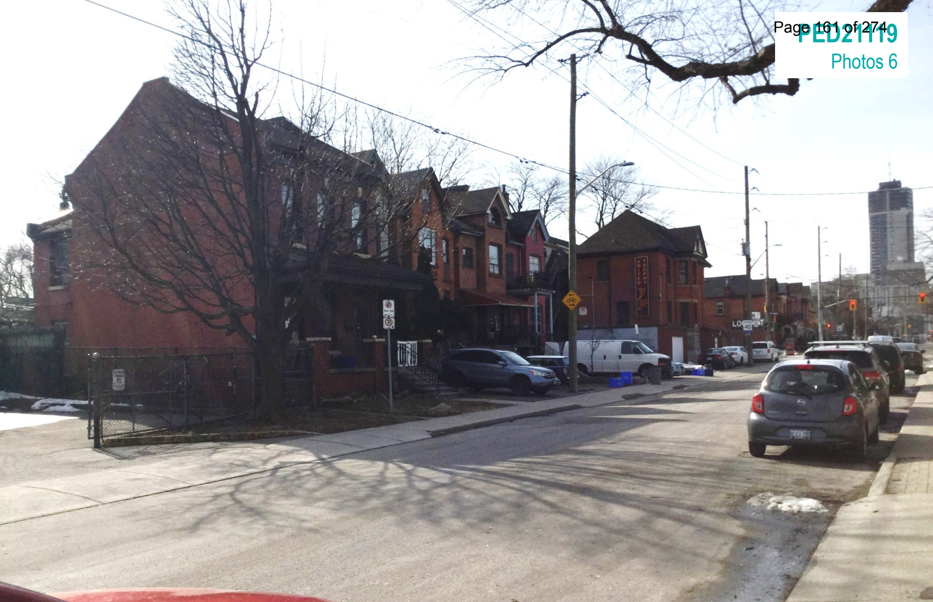
164-172 Catharine Street North located to the south east of the subject lands, as seen from Catharine Street North looking south east
