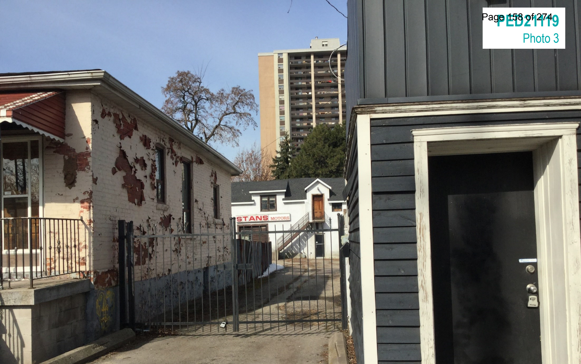
Between 181 and 183 Catharine Street North showing the existing repair garage located at the rear of the subject property, as seen from Catharine Street North looking west
