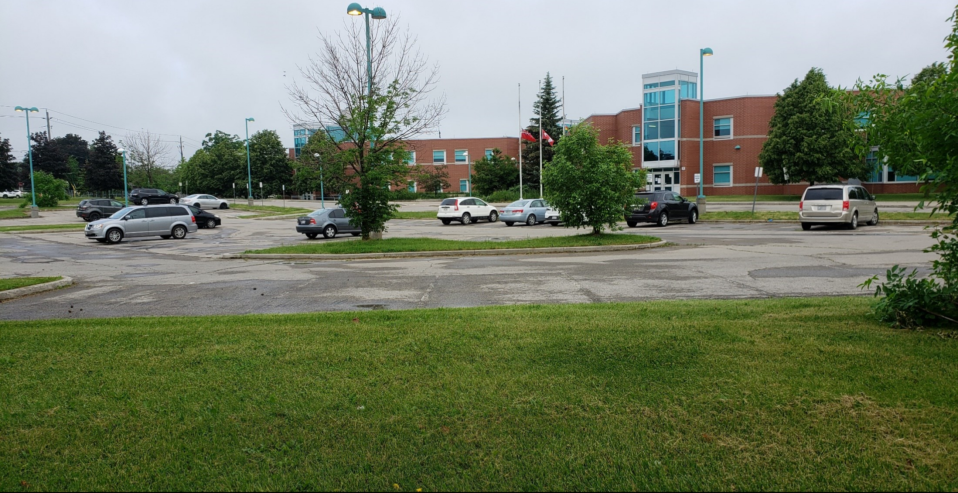
Saltfleet District High School
