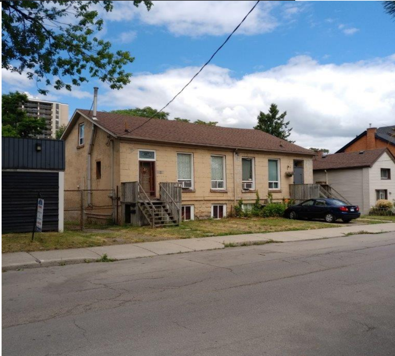
Retained Pre-Confederation Heritage Dwelling
