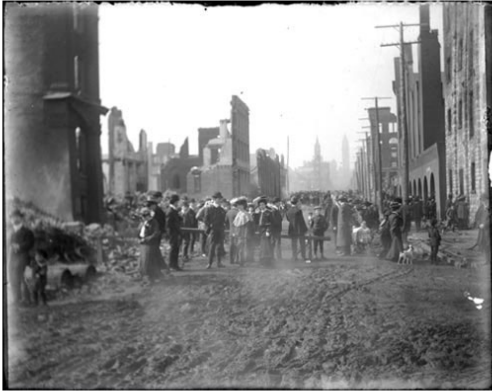
Figure 8. Toronto Fire 1904 (Image courtesy of Archives of Ontario).
