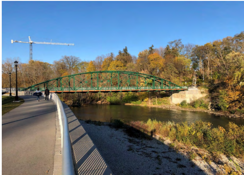
Figure 35. Blackfriars Bridge - 1875 wrought iron bowstring arch bridge underwent a major rehabilitation in 2017-2018 (Image courtesy of the City of London).
