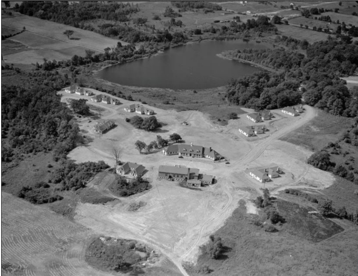
Figure 3. The Western Counties Health and Occupation Centre is a listed on the City of London's Register of Cultural Heritage Resources (Image courtesy of the City of London).
