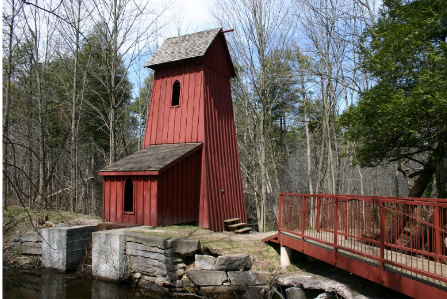
Figure 20. Sheave Tower (MHSTCI)
