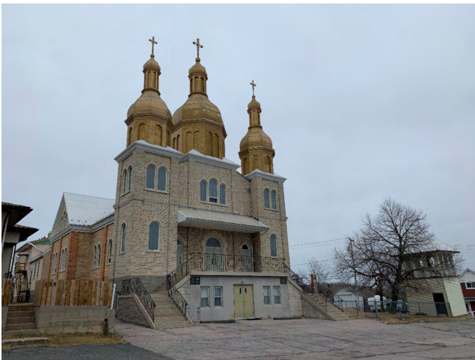
Figure 3. St. Nicholas Ukrainian Catholic Church in Kenora is listed on the municipal register of heritage properties (Image courtesy of the City of Kenora).
