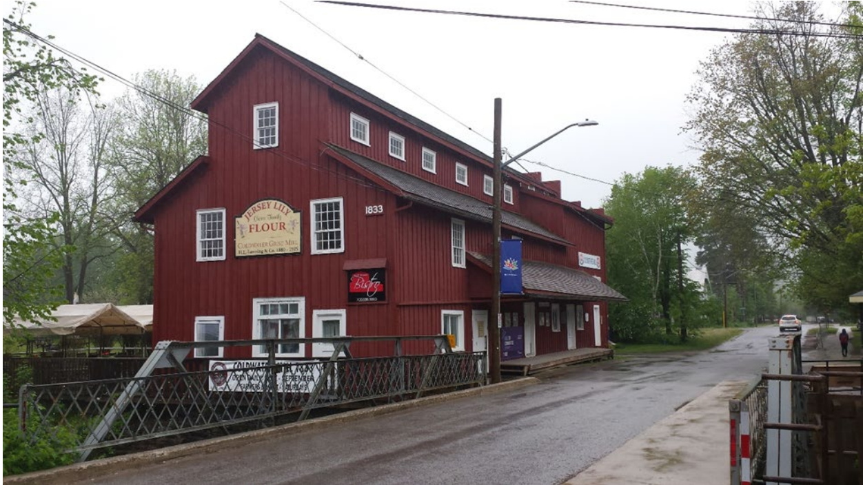
Figure 18. Cold Water Mill - A two-storey addition was added to the back of the Mill with barrier free entrance and washrooms. A cultural centre and Indigenous Gallery is planned for the second floor (Image courtesy of Coldwater Mill Heritage Foundation).
