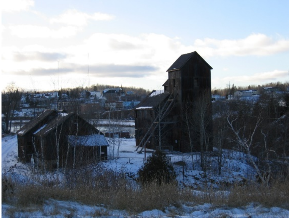
Figure 7. Townsite Shaft 1 Headframe in Cobalt (MHSTCI).
