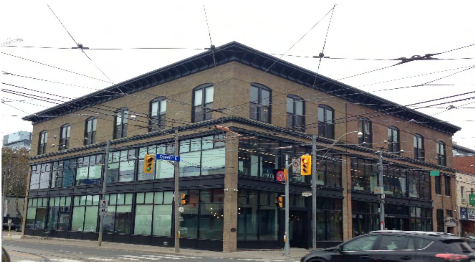
Figure 17. As can be seen in these photos depicting the restoration of 339 Queen Street East in Toronto, material changes to a property do not necessarily result in a loss of integrity. In this case, the building was restored by reinstating the features that contribute to its cultural heritage value (Image courtesy of the City of Toronto).
