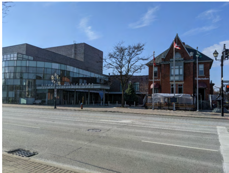
Figure 1. "10268 Yonge Street – Built in 1897, the original Richmond Hill High School was later used as the town hall and a library. It is now a well-loved coffee house. It was restored by the City of Richmond Hill and integrated into the newly built Richmond Hill Centre for the Performing Arts (Images courtesy of the City of Richmond Hill).
