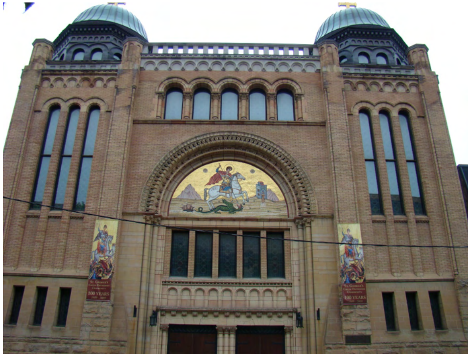
Figure 22. St. George's Greek Orthodox Church, Toronto. (Image courtesy of the Ontario Heritage Trust).
