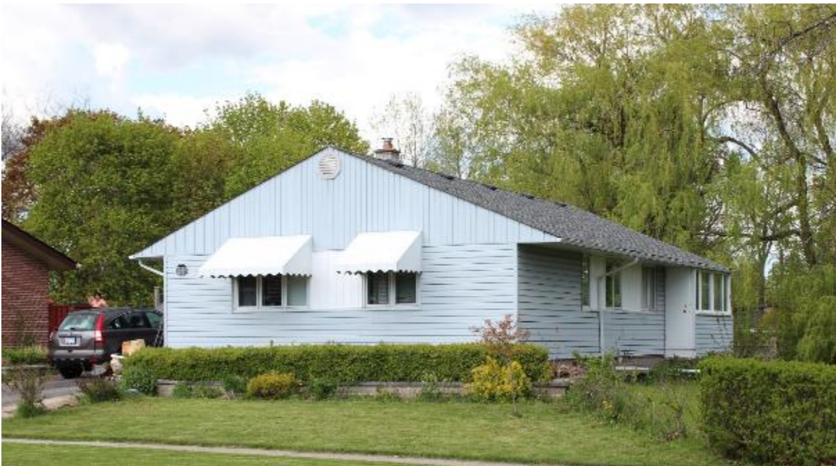
Figure 2: Typical postwar single-family dwelling (Image courtesy of the City of Ajax).
