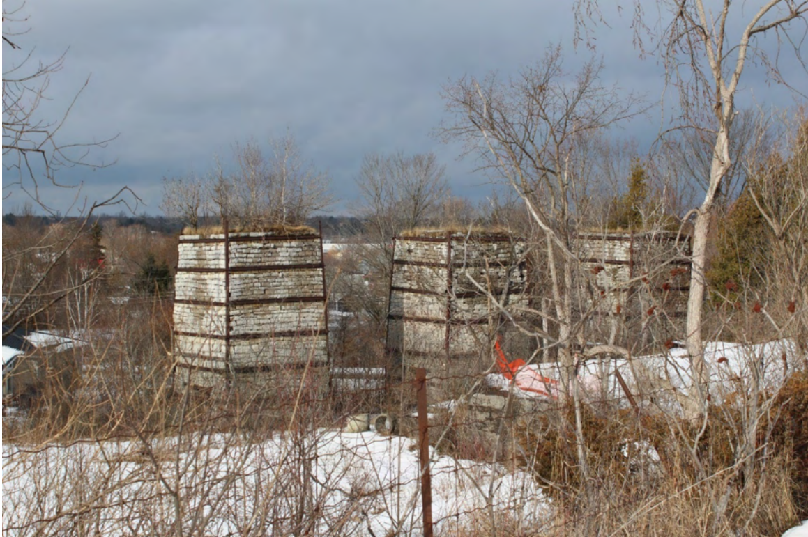
Figure 12. Coboconk Lime kilns - Limestone became an important part of the local economy as it was often refined and sold for range of use in construction, industry and agriculture (Image Courtesy of the City of Kawartha Lakes).
