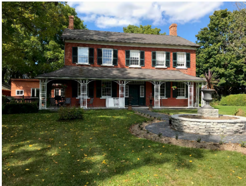
Figure 13. Brazel Chambers House – This home reflects the building technologies of upper Canada in the mid 19 th century. The designation includes its original doors windows and shutters (Image courtesy of Bradford West Gwillimbury).
