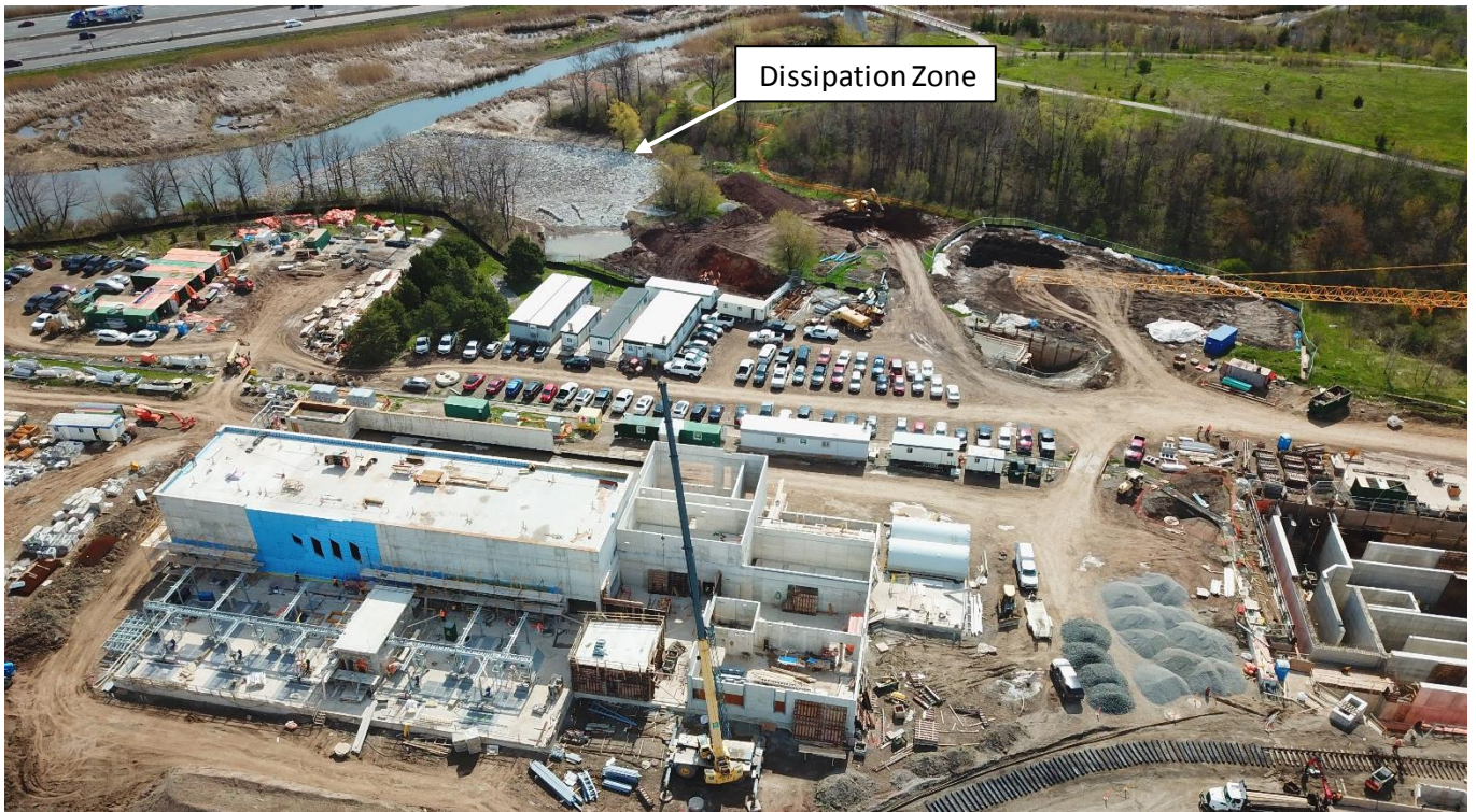
Figure 8: New Tertiary Treatment Facility Construction with Effluent Dissipation Zone
