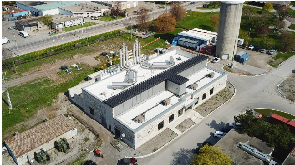
Figure 4: New Electrical Power Centre
