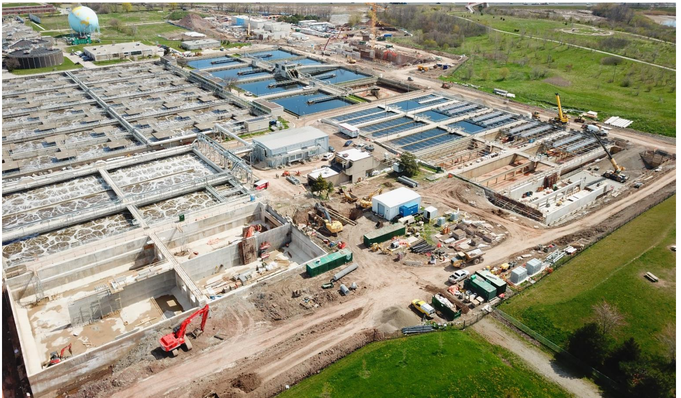
Figure 9: South Secondary Treatment Plant Upgrades Construction
