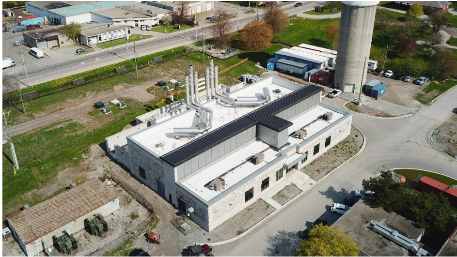
Figure 4: New Electrical Power Centre
