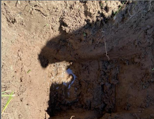
11. Leaching field saturated – water above distribution pipes
