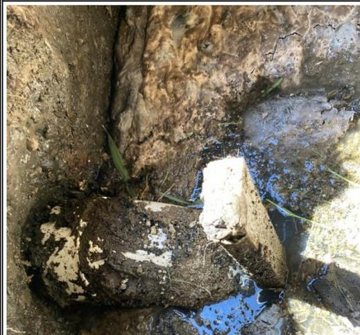
5. 90 degree elbow baffle installed 4 years prior – air locking system causing high levels
