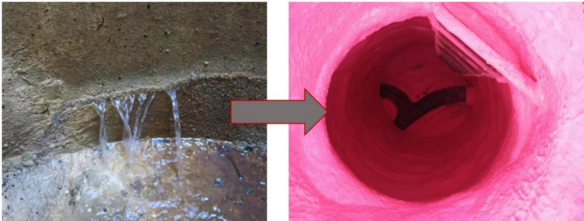
**Figure 1.2: Infiltration in Manhole (left) and SpectraShield® Sealant in Manhole to Mitigate Infiltration (Right)**
