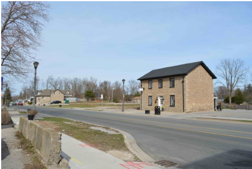
A view from the west side of Wilson Street East looking towards the property at 392 - 406 Wilson Street East looking south. The Marr House is visible here, and is adjacent to a surface level parking lot to the south. This is the location of the former gas station.
