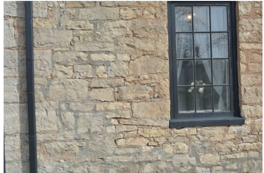
West elevation: ground level showing cementitious parging applied at the northern edge of the building.
