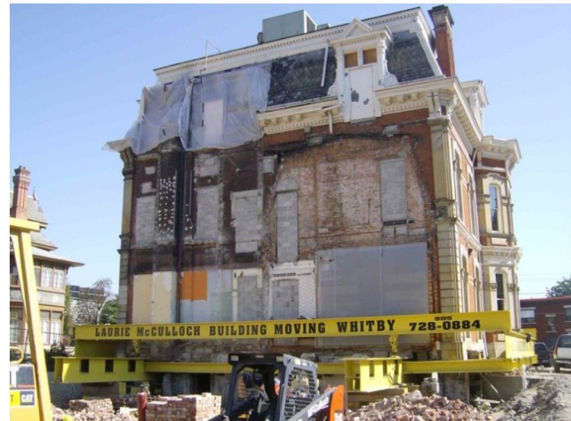
James Cooper Mansion relocation in Toronto (2008)
