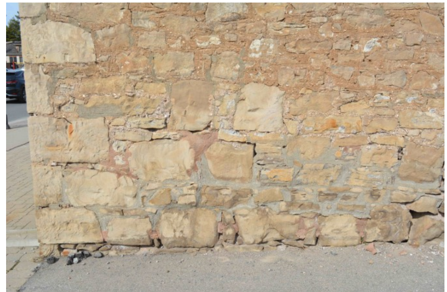
South elevation: ground level showing open joints, and repair work.
