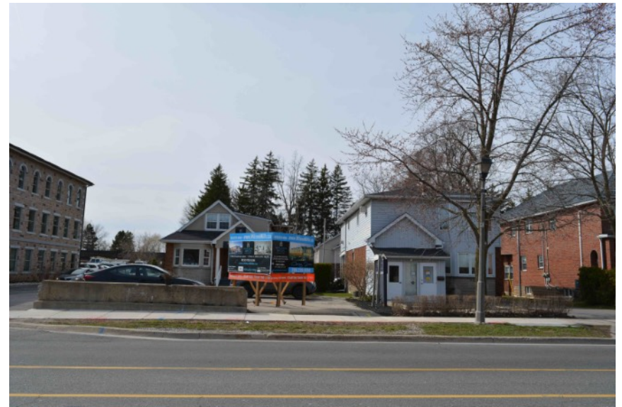
View from the subject site directly north across Wilson Street East.
