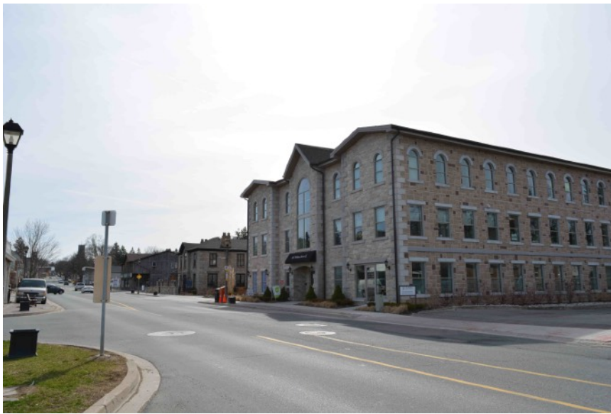
Looking south from the corner of the subject site towards 385 Wilson St. East, a professional/commercial building with pre-cast moulded concrete blocks that appears to be a scaled version of a Italianate style house. To the south of this is 375 Wilson Street East - the Rousseau house (1848).
