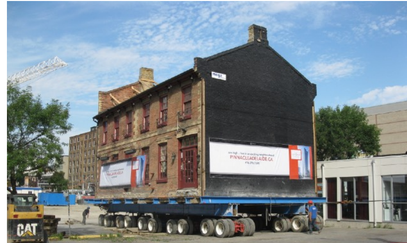
Richard West House relocation in downtown Toronto (2009)
