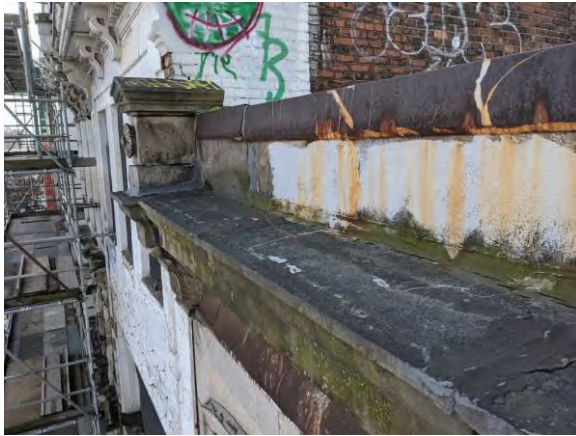
Fig 12: Cornice and stones above, at 22 King
