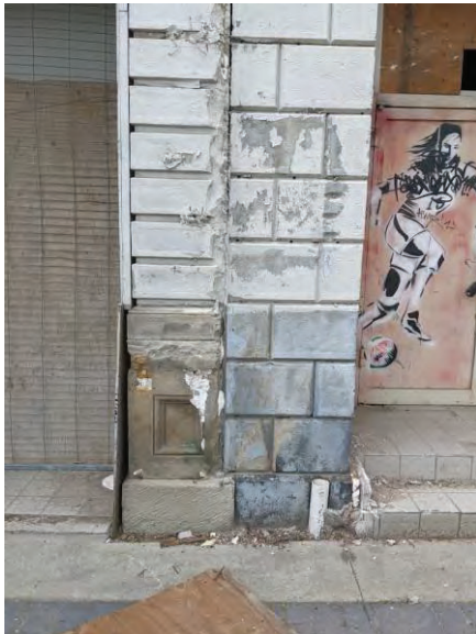
Fig 7: 18-20 & 22, example of ground level masonry
