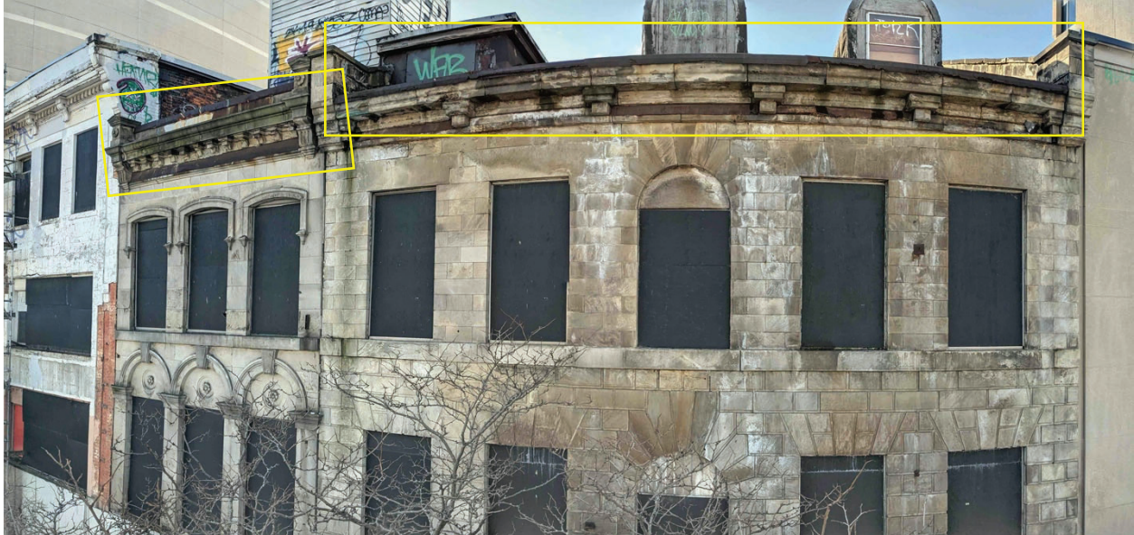
18-22 KING E (KERR BUILDINGS) – significant deterioration of stone cornice due to failure of the roof and gutters
