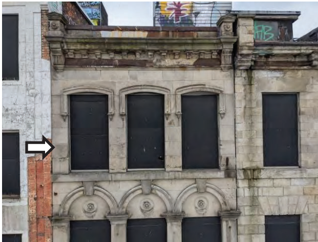
Fig 8: 22, cornice and bands of stone below. Sliding indicated. Fig 9: 22, sliding at base of 3 rd flr pier, E side.
