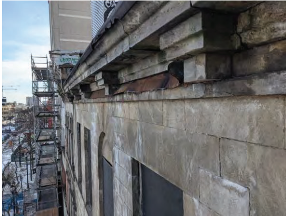
Fig 5: 18-20, cornice and bands of stone below.
