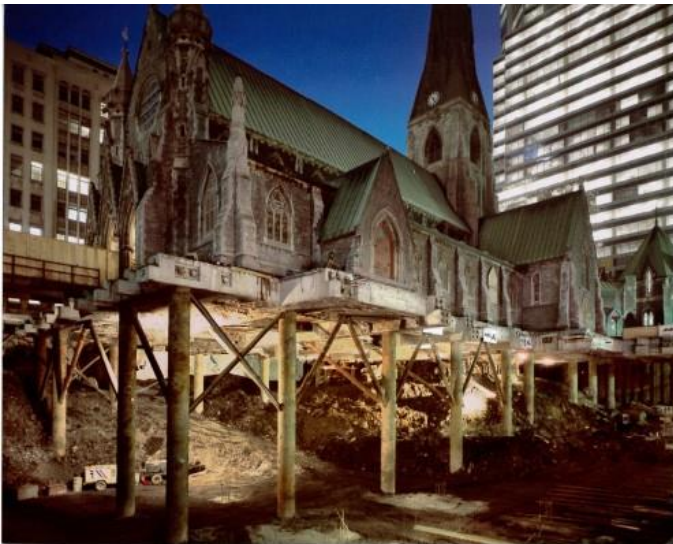
Caissons and pre-stressed beams support the Cathedral
