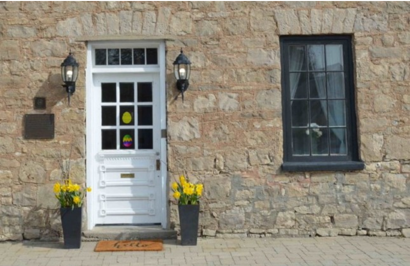
West elevation: Central door with with 12-over-12 sash and five-pane toplight is in good repair.
