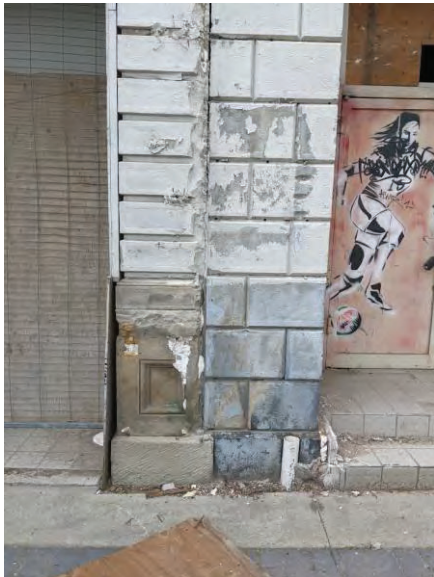
Fig 7: 18-20 & 22, example of ground level masonry
