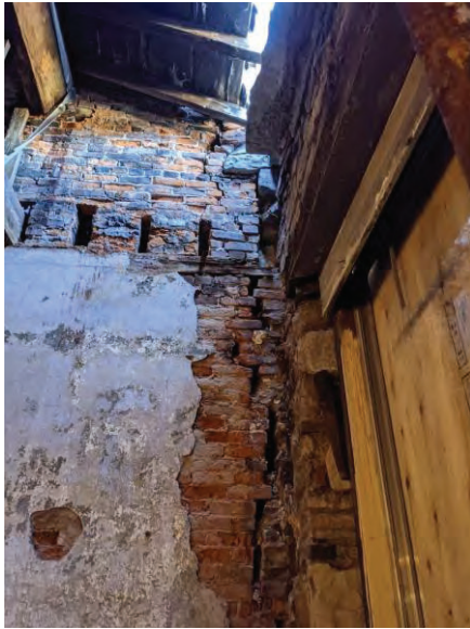
Fig 1: 18-20, 3 rd floor, West return wall separation
