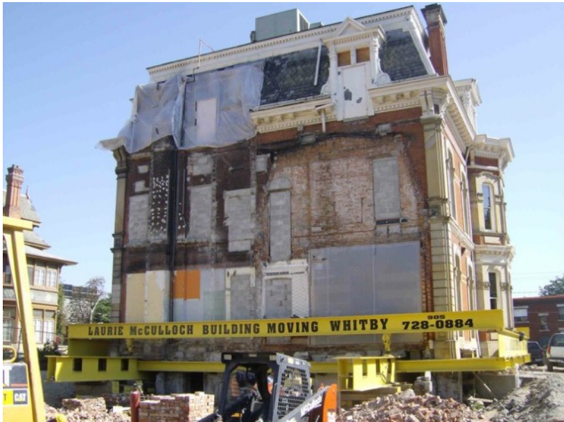
James Cooper Mansion relocation in Toronto (2008)
