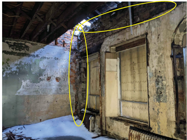
18-22 KING E (KERR BUILDINGS) – significant deterioration of stone cornice due to failure of the roof and gutters
