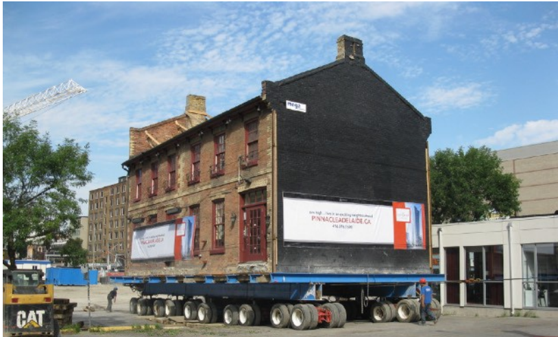
Richard West House relocation in downtown Toronto (2009)
