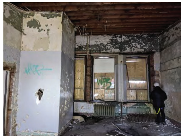
Fig 11: 22, roof framing, connected to adjacent bldg's.
