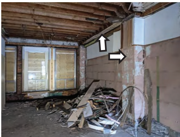
Fig 10: 22, beam and piers underside 3 rd floor framing
