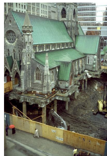
Caissons and pre-stressed beams support the Cathedral
