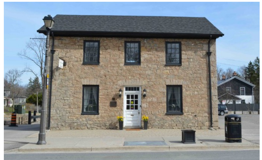
Marr House, 2021 (GBCA). West Elevation 2.4 meters from Wilson Street East. Although the designation by-law notes that chimneys are a contributing heritage attribute, in its current state these are no longer present.
