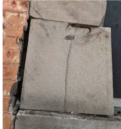
Fig 8: 22, cornice and bands of stone below. Sliding indicated. Fig 9: 22, sliding at base of 3 rd flr pier, E side.
