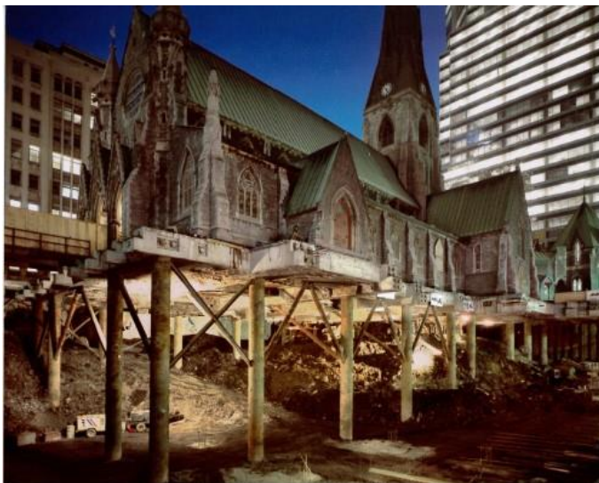
Caissons and pre-stressed beams support the Cathedral
