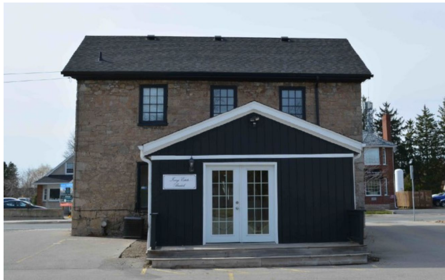
Marr House, 2021 (GBCA). East Elevation. Rear tail covers to ground level openings.
