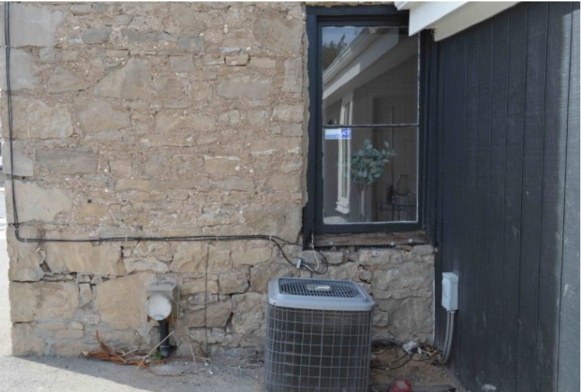
East elevation: Openings at rear elevation have been obscured by the later addition of a one-storey tail.
