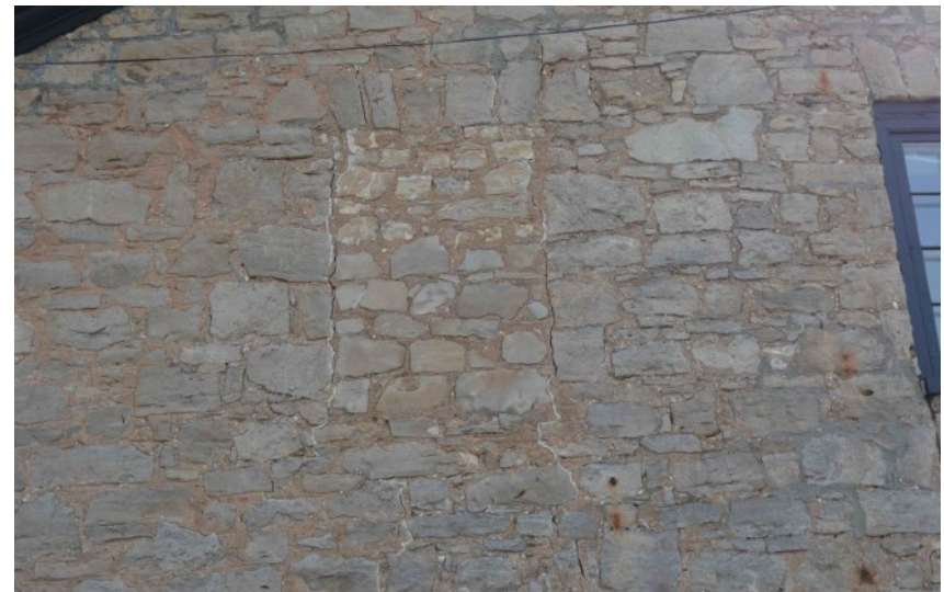
North elevation: eastern-most window opening on 2nd storey has been closed in.
