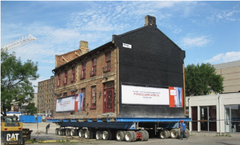
Richard West House relocation in downtown Toronto (2009)
