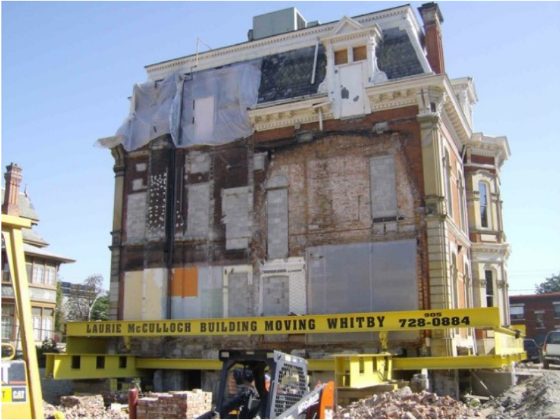
James Cooper Mansion relocation in Toronto (2008)
