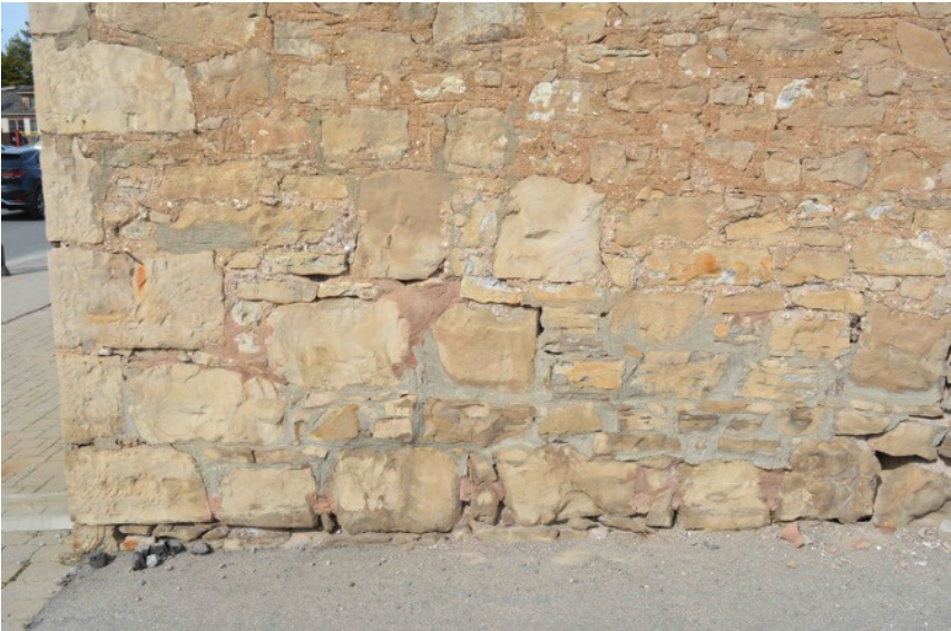
South elevation: ground level showing open joints, and repair work.
