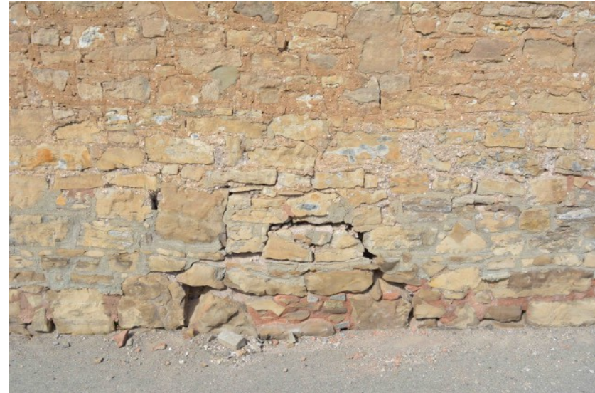
South elevation: ground level failed and open joints with previous repair work also visible.
