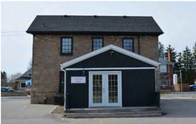
Marr House, 2021 (GBCA). East Elevation. Rear tail covers to ground level openings.
