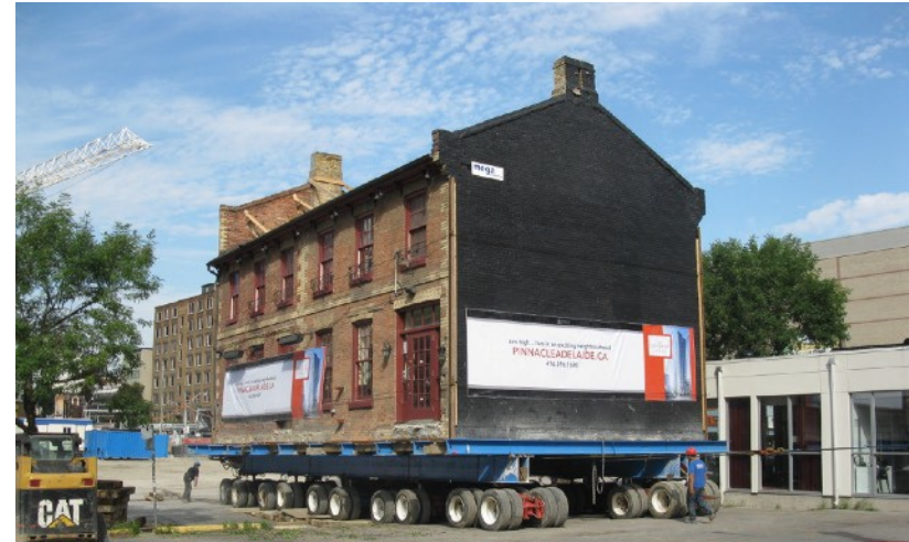
Richard West House relocation in downtown Toronto (2009)
