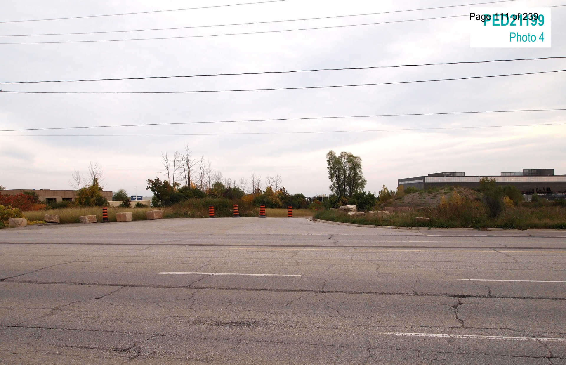
Future Road "Street C" from Hwy #5
