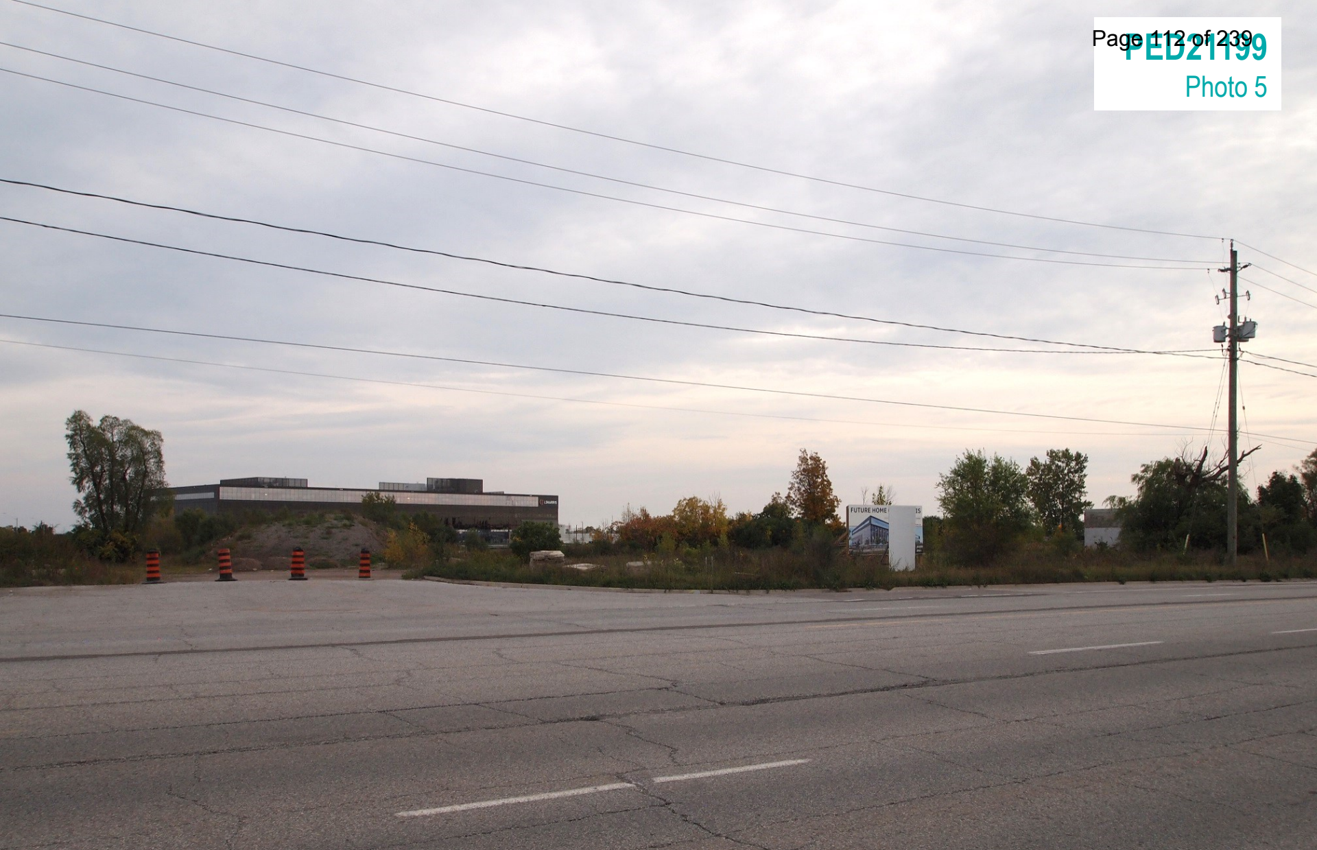
South Lands from Hwy #5, L3Harris in the background
