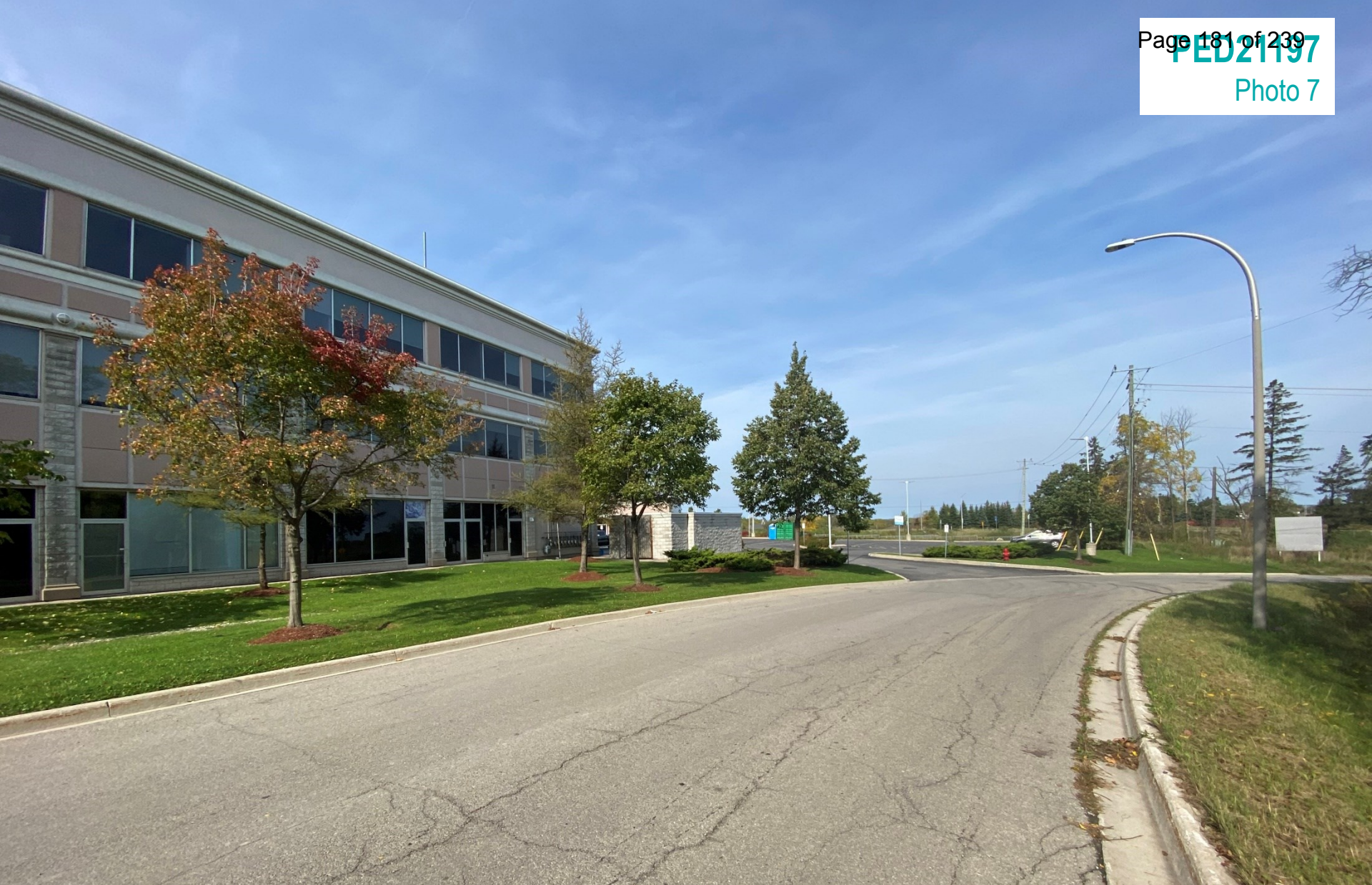
Urbanized streetscape of Old Golf Links Rd
