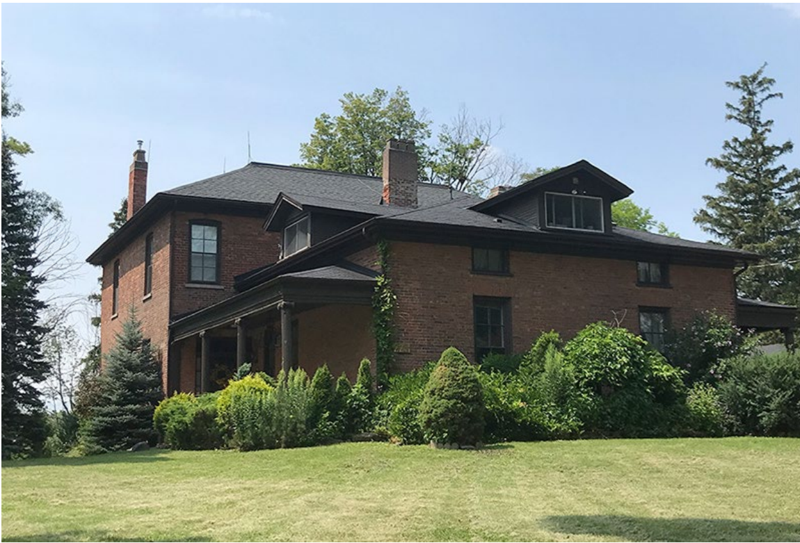
South and east façades of former Maw residence facing Governor's Road at #223.
