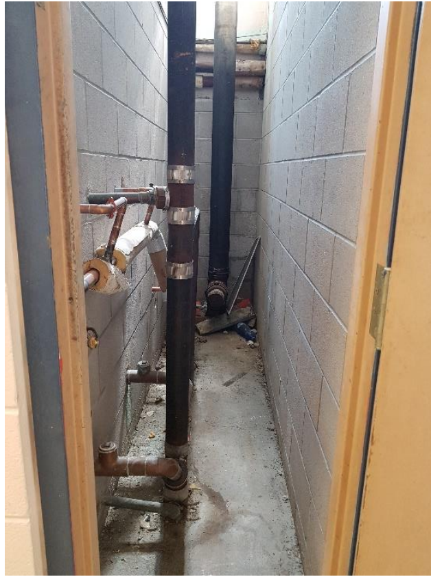
Figure 45: Utility room (1974/75) withing male change room, looking east.
