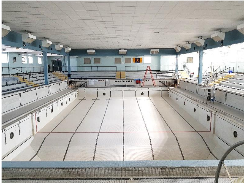
Figure 81: Pool floor, looking north. Stairs to the change rooms, gutters along the east and west limits of the pool, and drop ceiling covering the former skylights are visible.
