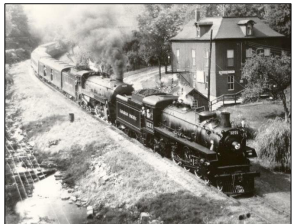
Figure 33: Passenger Train at Waterdown South Railway Station, circa 1920 (Flamborough Archives, BW 1095)
