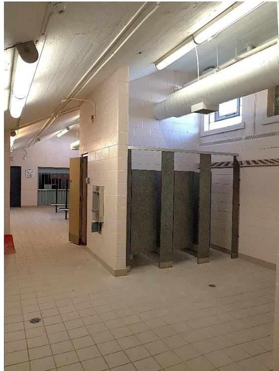
Figure 56: Female change room, looking south west. Air vents installed during 1974/75 updates.
