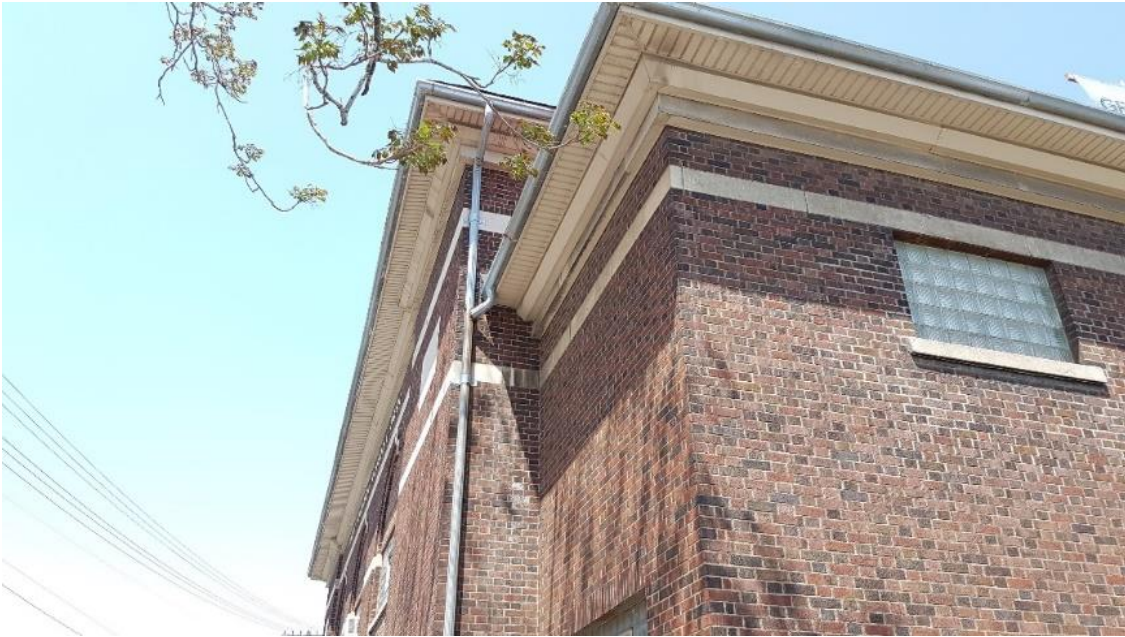
Figure 27: Projective eaves and verges, looking at the south east corner of the frontispiece.
