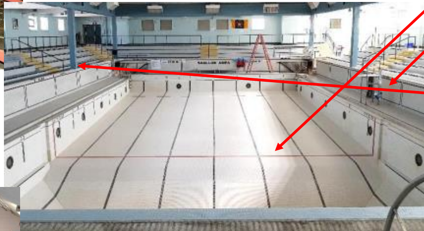
Tiled pool barrier wall
