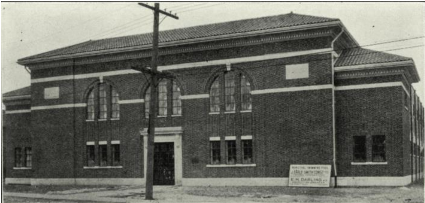
Front façade of the pool, presumed while the building was still under construction since there is a board leaning against the wall that names the J. Earle Smith Construction Company and E.H. Darling.
