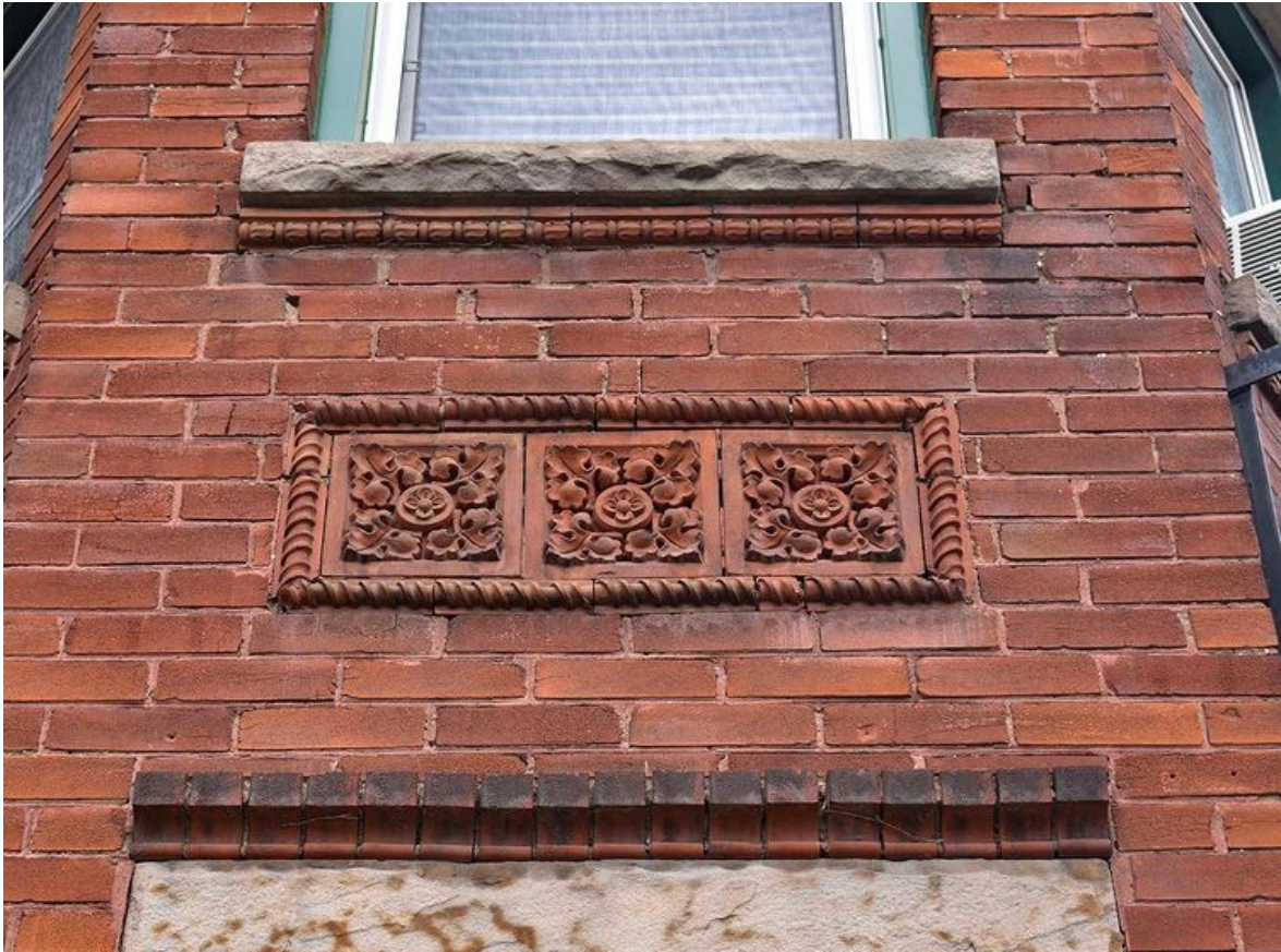
Terra Cotta on east facade
