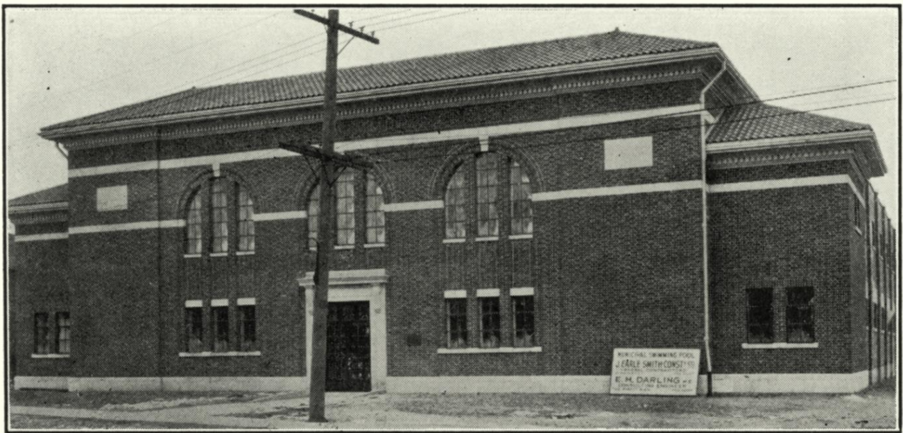
Figure 11: Front façade of the pool, presumed while the building was still under construction since there is a board leaning against the wall that names the J. Earle Smith Construction Company and E.H. Darling. This photo also appears to pre-date December 1929 as the "Municipal Swimming Pool" sign below the cornice had yet to be added (see Figure 10, from Darling 1933:423)
