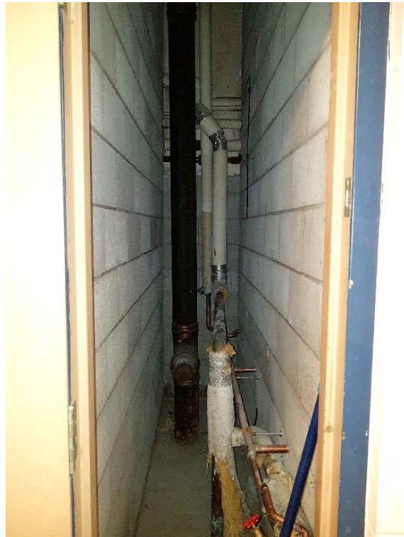
Figure 54: Utility room (1974/75) within female change room, looking west.
