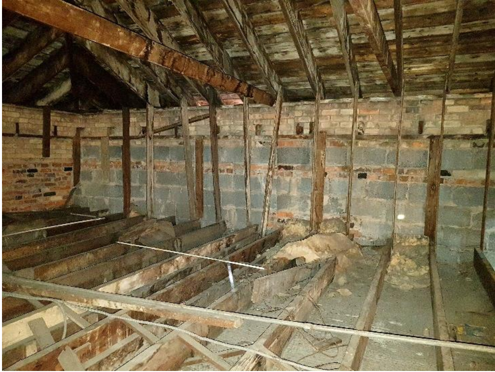
Figure 84: Looking south east within the attic space of the frontispiece.
