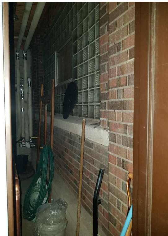
Figure 26: Sill and glass block of the west window as seen from inside the 1974/75 addition.
