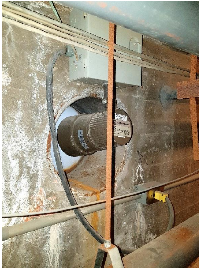
Figure 73: Updated under water pool light.
