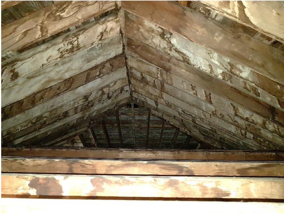
Figure 86: Timber-framed hipped roof of the frontispiece.
