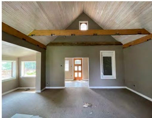
Fig. 5.16. Fully renovated interiors
