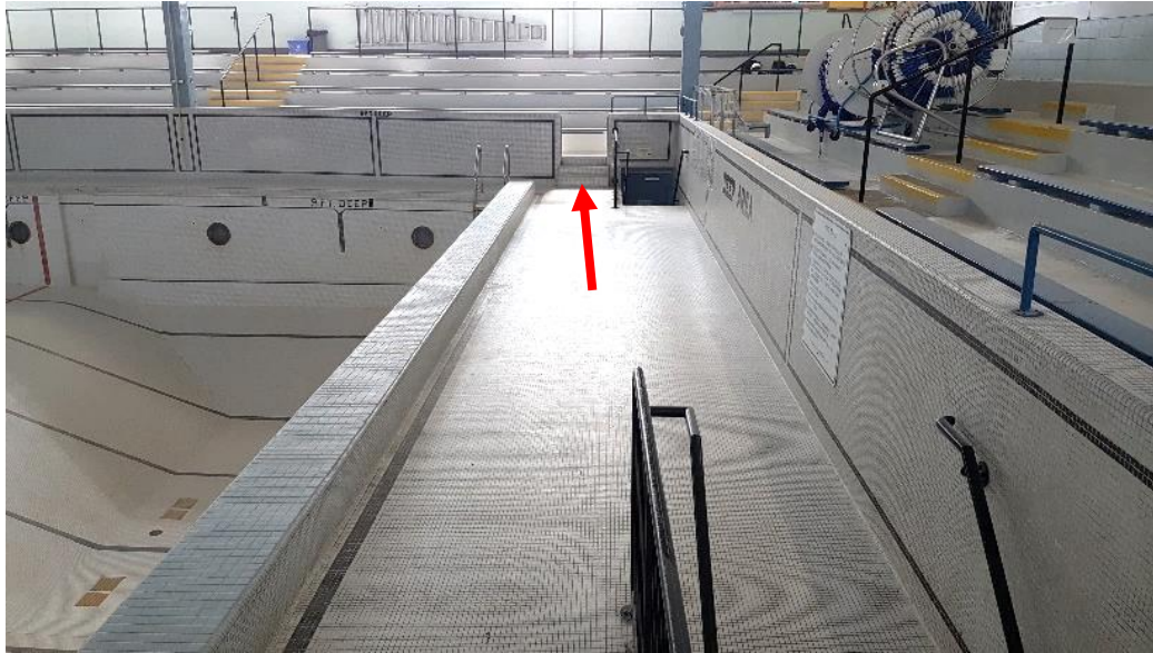
Figure 79: Entrance to the pool deck from the bleachers, looking east.
