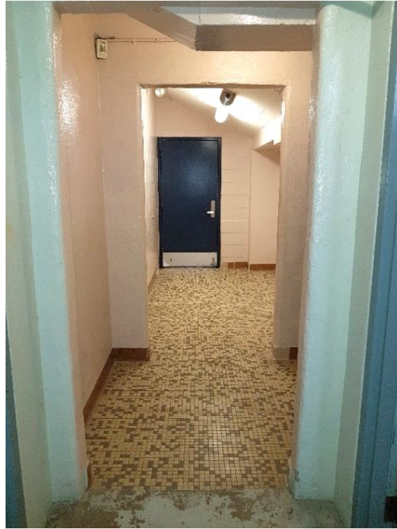
Figure 49: Corridor north of male change room, looking north. Reconfigured in 1974/75.
