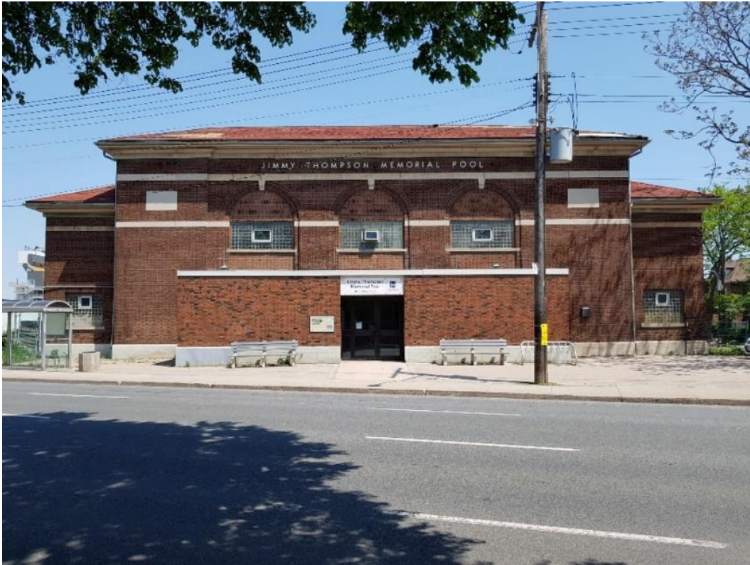
Figure 25: Looking north at the south facade of the Jimmy Thompson Memorial Pool and the 1974/75 addition.
