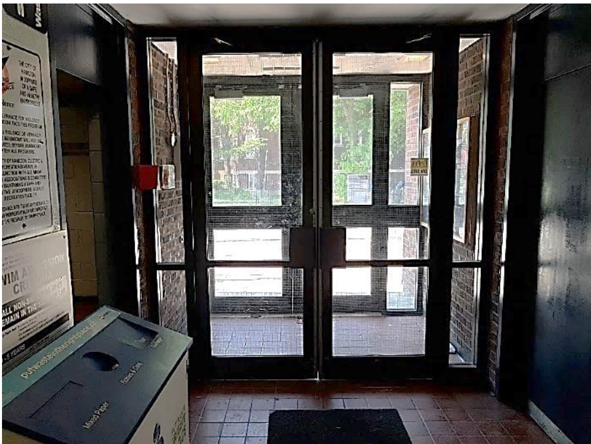
Figure 34: Looking south at the main entrance and vestibule associated with the 1974/75 addition.
