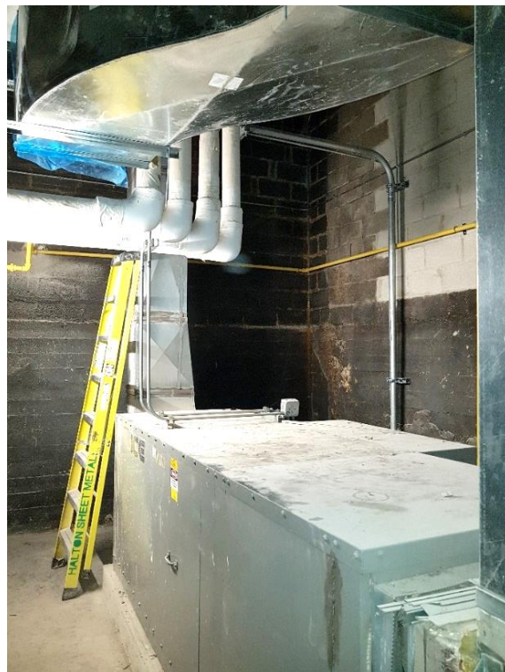
Figure 66: Air conditioning room, formerly employed as a storage room.
