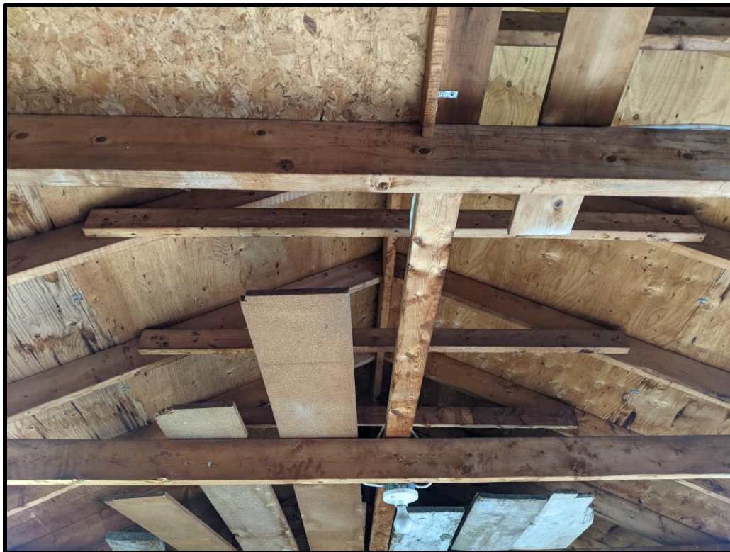
Interior of Garage (Roof), 19 Mill Street South, Waterdown City of Hamilton 2021
