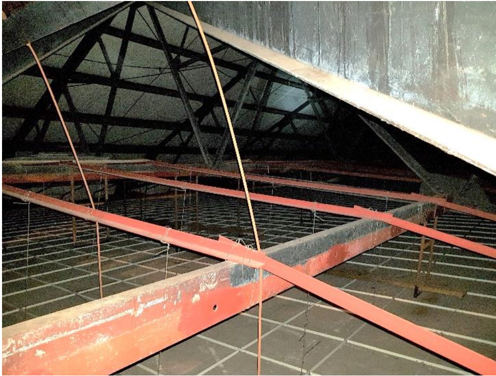
Figure 88: Original metal trusses of the skylight, looking northwest.
