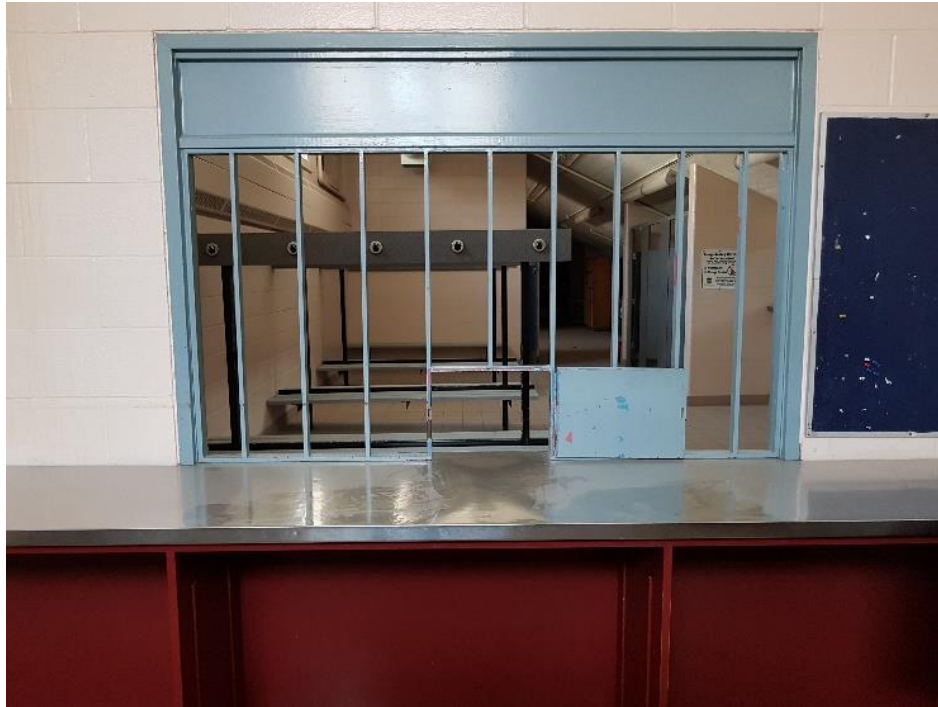
Figure 41: Female check room, looking north into female change room. Room was reconfigured in 1974/75.
