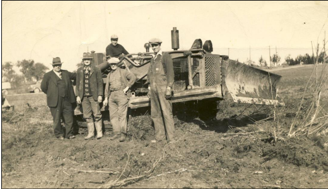
Figure 43: Work starting on Memorial Park, circa 1946 (Flamborough Archives, BW 2405)
