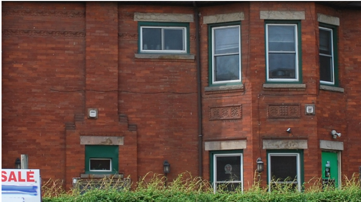
Terra Cotta Panel on south side of tower
