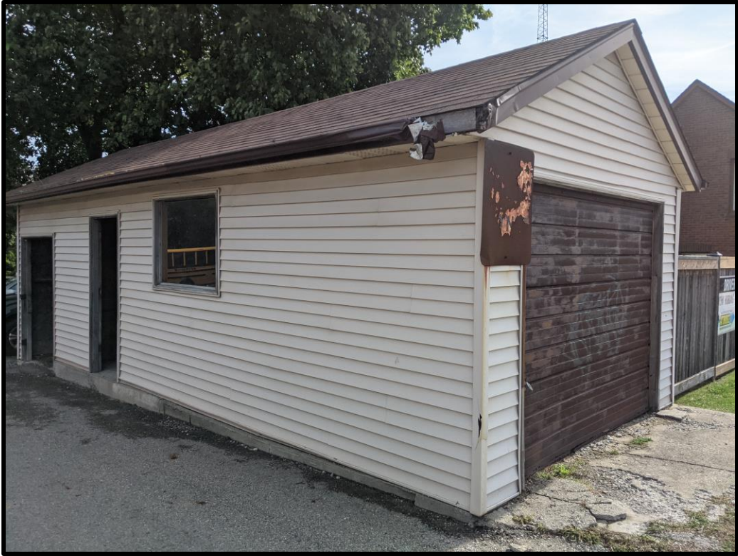
Exterior of Garage, 19 Mill Street South, Waterdown City of Hamilton 2021
