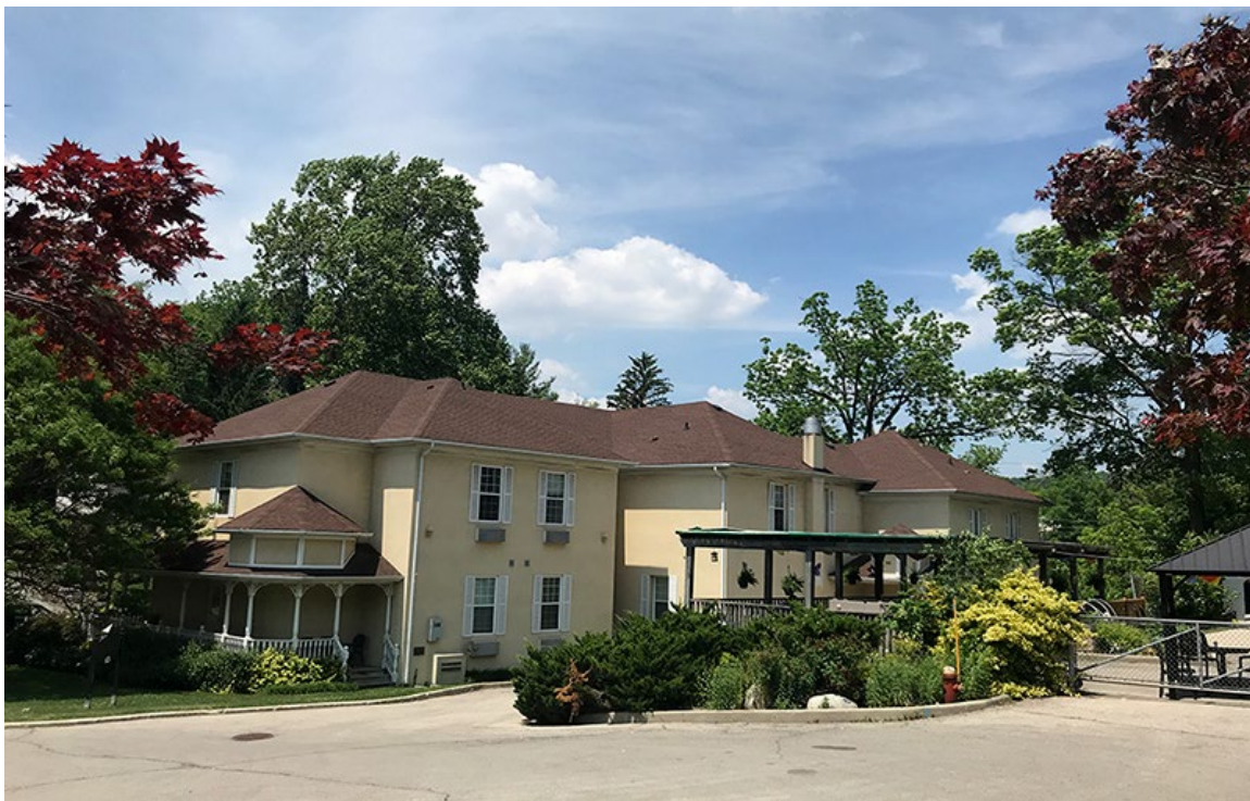
East (rear) façade with three wings that were likely a later addition to the factory building. There are two entrances at each end of the building.
