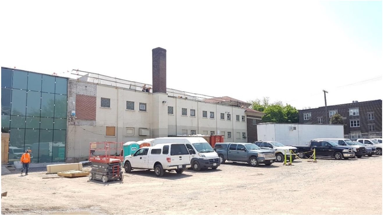
Figure 29: Looking southeast at the west facade of the Jimmy Thompson Memorial Pool.
