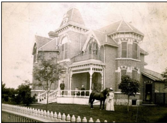
Figure 25: 288 Dundas Street East (Carson House) in the late-nineteenth century (Facebook, Posted by J. Vance, Oct 21, 2018)
