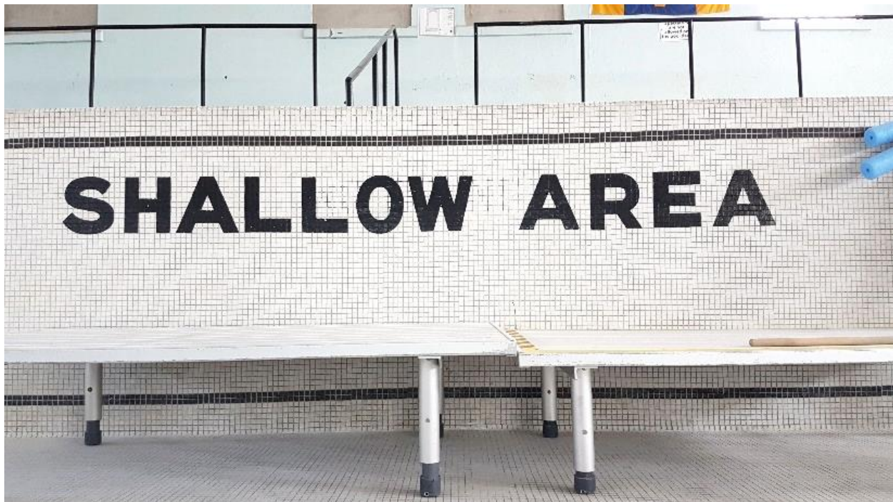
Figure 78: Letters are ascribed by hand; a later addition likely to meet health and safety requirements.
