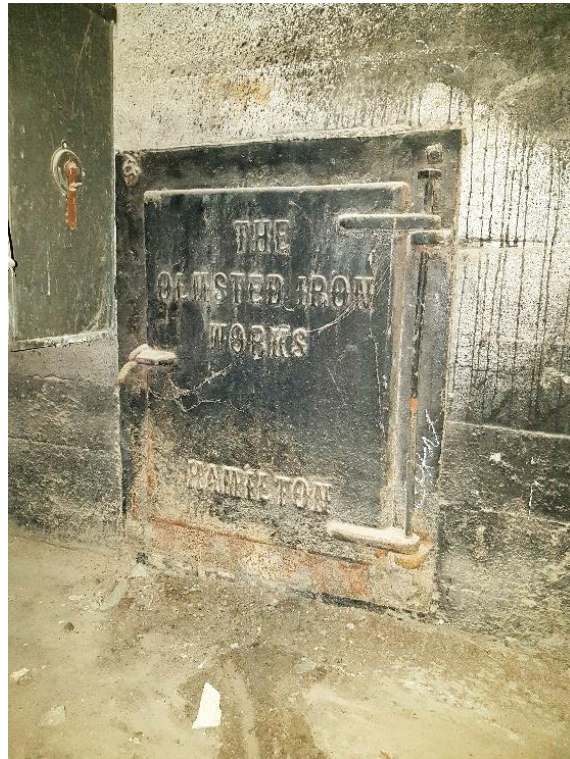
Figure 65: Chute to the original coal furnace.
