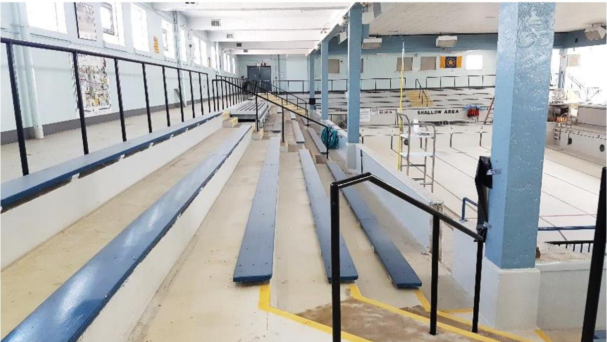
**Figure 74: Bleacher rows along the west side of the pool, looking north. Note, the absence of the Corinthian capitals and decorative base on the columns. Roof columns are evident. The drop ceiling over the former skylight is visible.**
