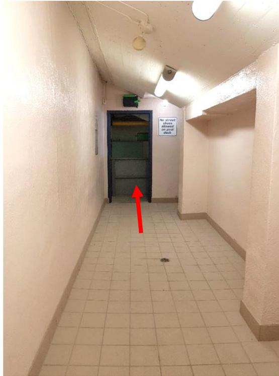
Figure 59: Corridor north of female change room, looking north. Wall at north end was opened and a door installed in 1974/75 for access to an emergency exit.
