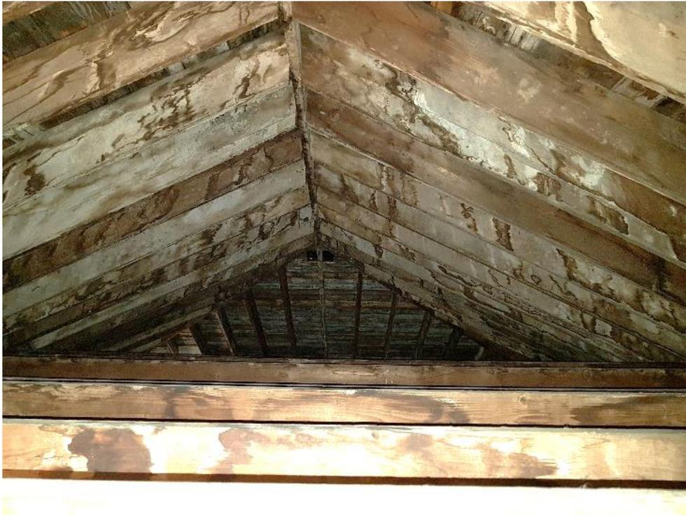
Figure 86: Timber-framed hipped roof of the frontispiece.
