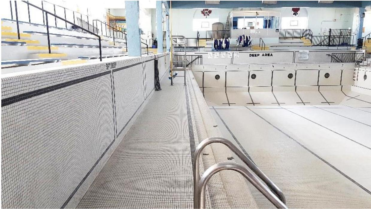
Figure 77: Wall separating bleachers from the deck level, looking south. Gutters are visible between the deck and pool.
