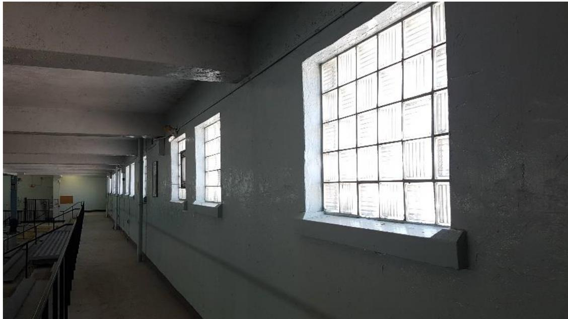
Figure 76: Updated glass-block windows along west side of pool. Note, some of the windows are fitted with a centre single-hung opening.
