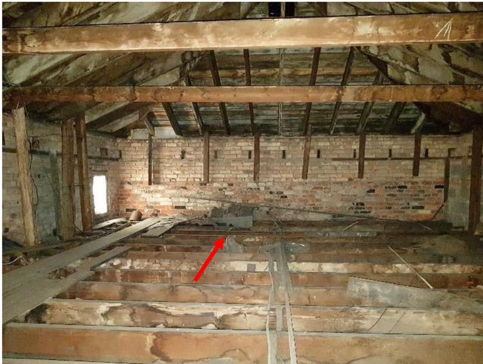
Figure 83: Looking east within the attic space of the frontispiece. The arrow points to red roof tiles, which may be the original to the frontispiece.
