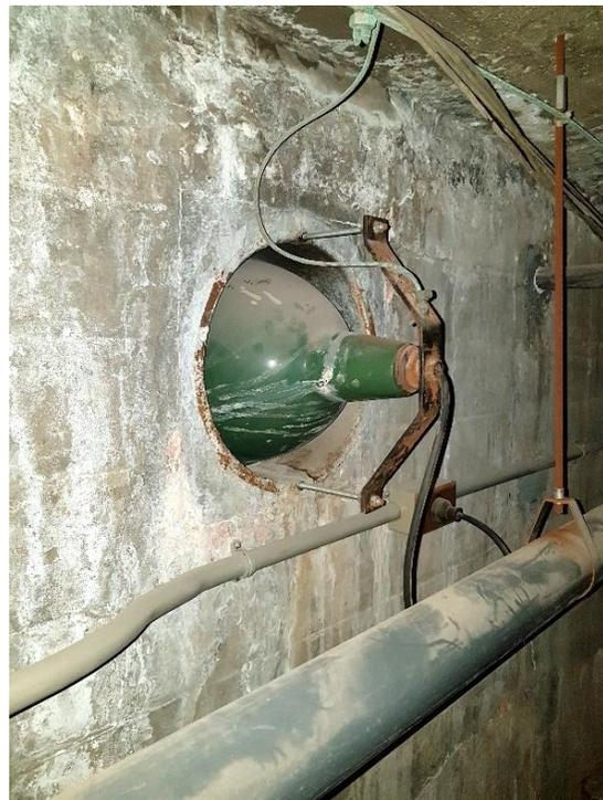
Figure 72: Under water pool light; this light appears to be original. Note, marks of the board forms are visible on the cement.
