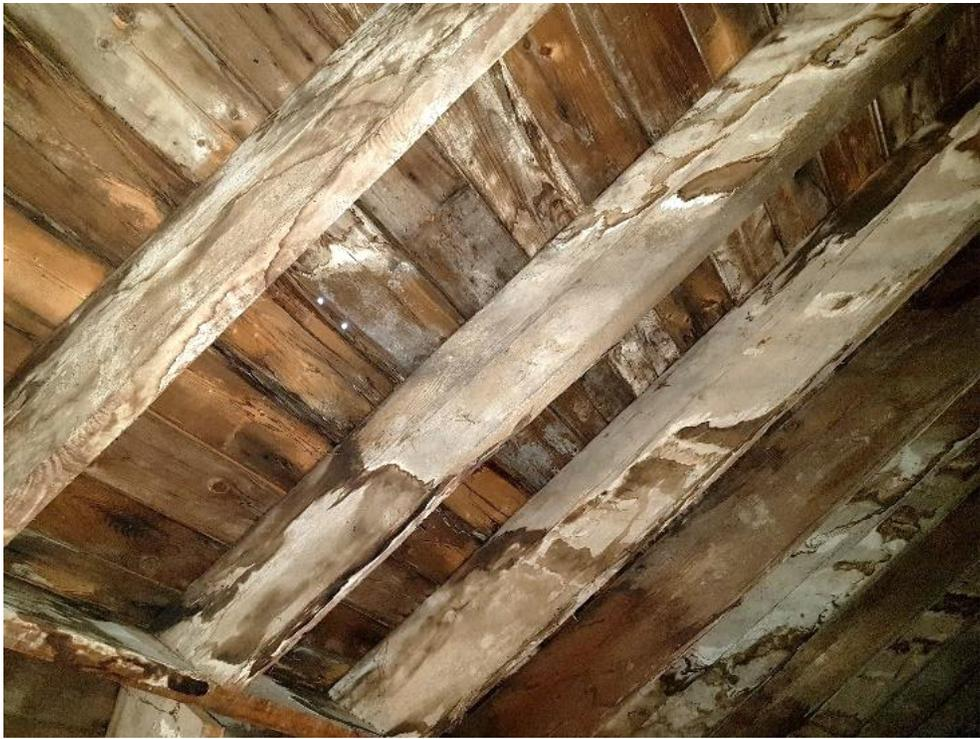
Figure 87: Roof deck on the frontispiece appears to be constructed in tongue and groove method.
