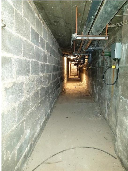
Figure 71: Pipe tunnel that runs around the perimeter of the pool. Note, electrical and pipes within pipe tunnel has been updated.
