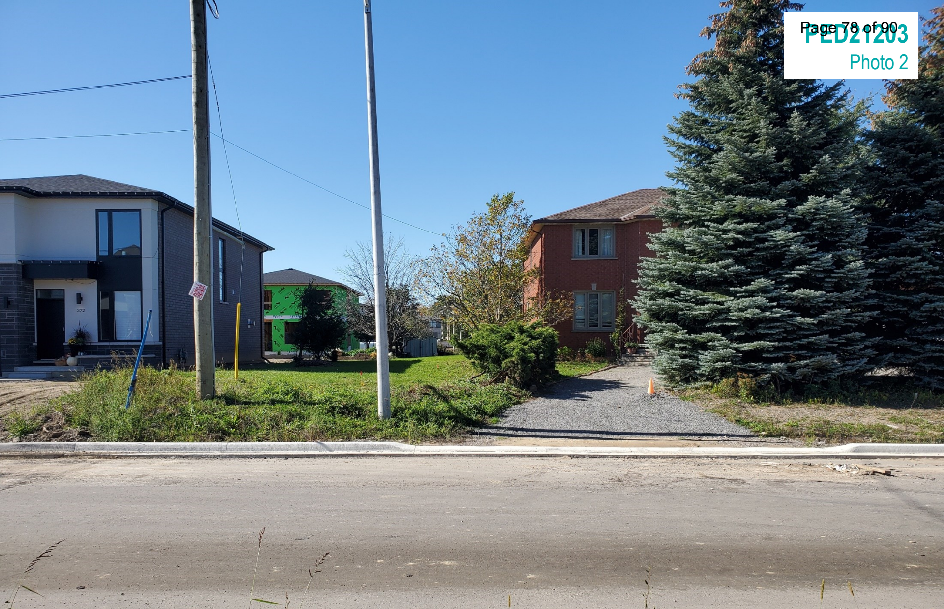
Looking Across the Street of Subject Property (West side of Springbrook Avenue)
