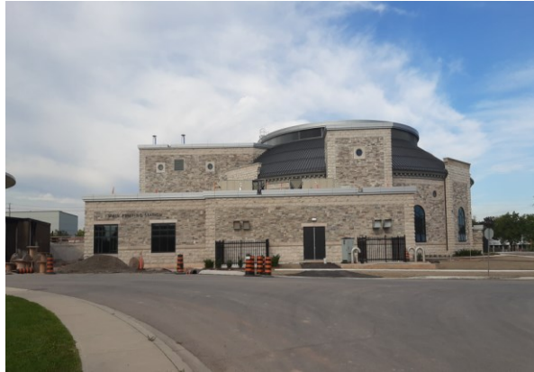
CONTRACT 1 Main Pumping Station
