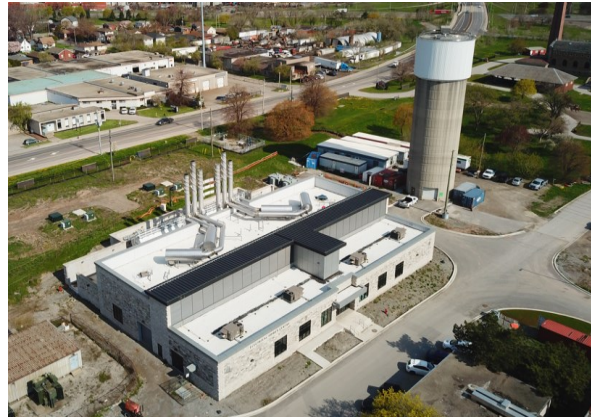
CONTRACT 2 Electrical Power Centre
