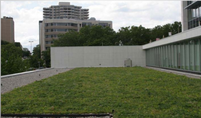
Hamilton City Hall Green Roof Lot Level Control
