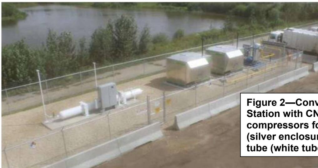
**Figure 2—Conventional CNG Station with CNG dryer (blue), two compressors for redundancy (silver enclosures), one storage tube (white tube with panel) (left).**
