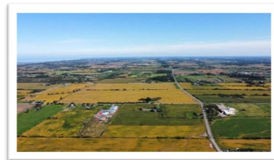
Rural roads - maintenance
