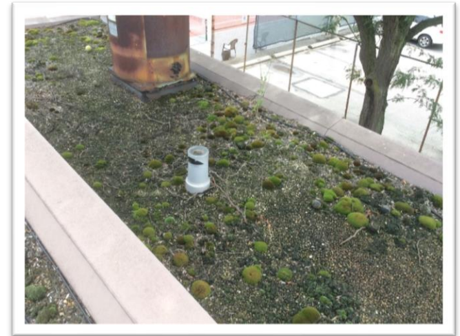
Rosedale tennis club roof
