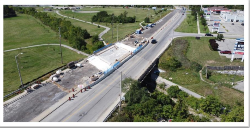
Mudd Street Bridge
