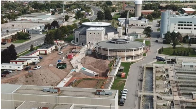
Wastewater pumping stations at the WWTP
