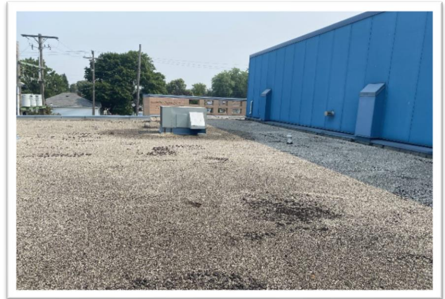
Inch Park arena roof
