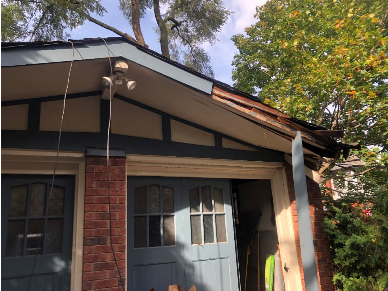
Photograph 2: Front Elevation - Original Brick (October 20, 2020)
