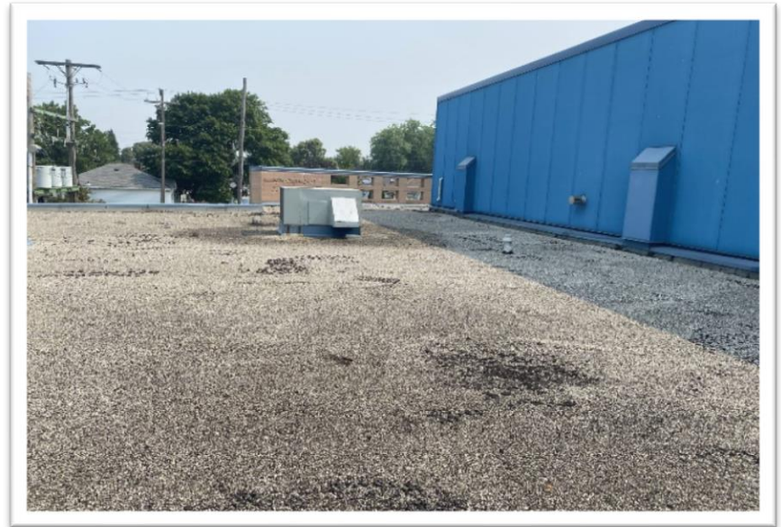
Inch Park arena roof
