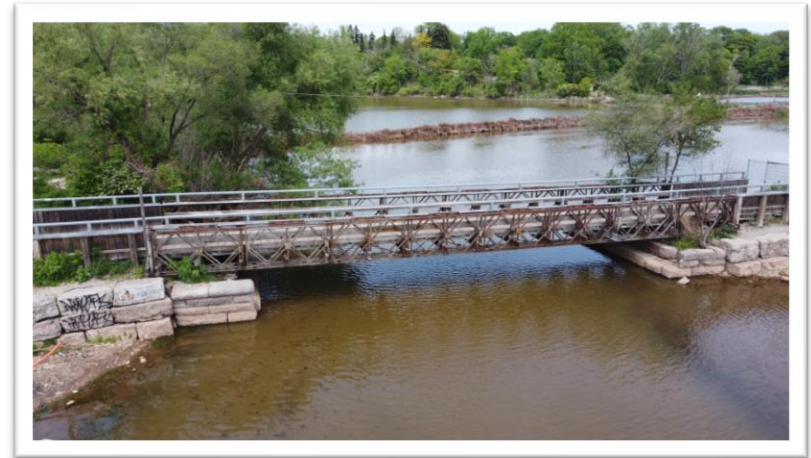
Valley Inn Bridge
