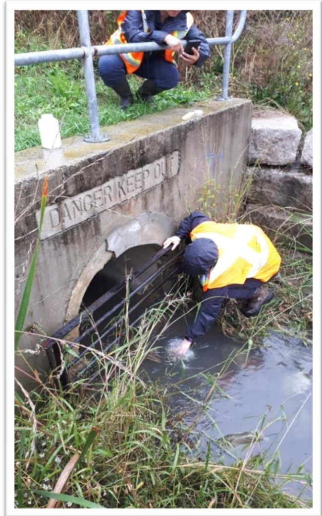
Stormwater outfall
