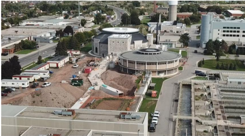
Wastewater pumping stations at the WWTP
