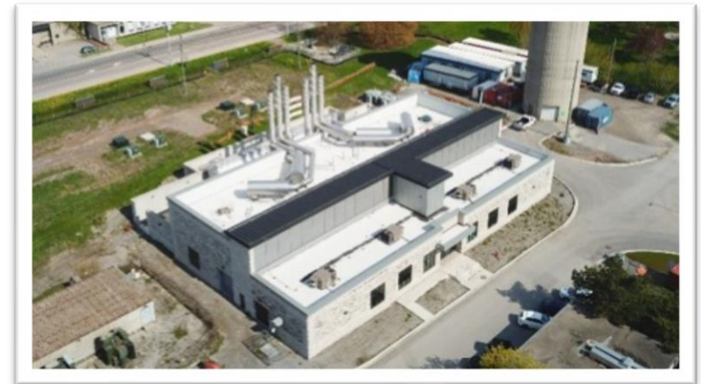
Electrical power centre – Woodward Upgrades
