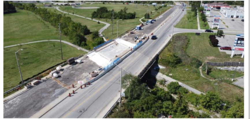
Mudd Street Bridge
