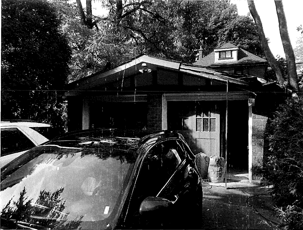
Image 1: Front of Building – Original Brick (October 20, 2020)
