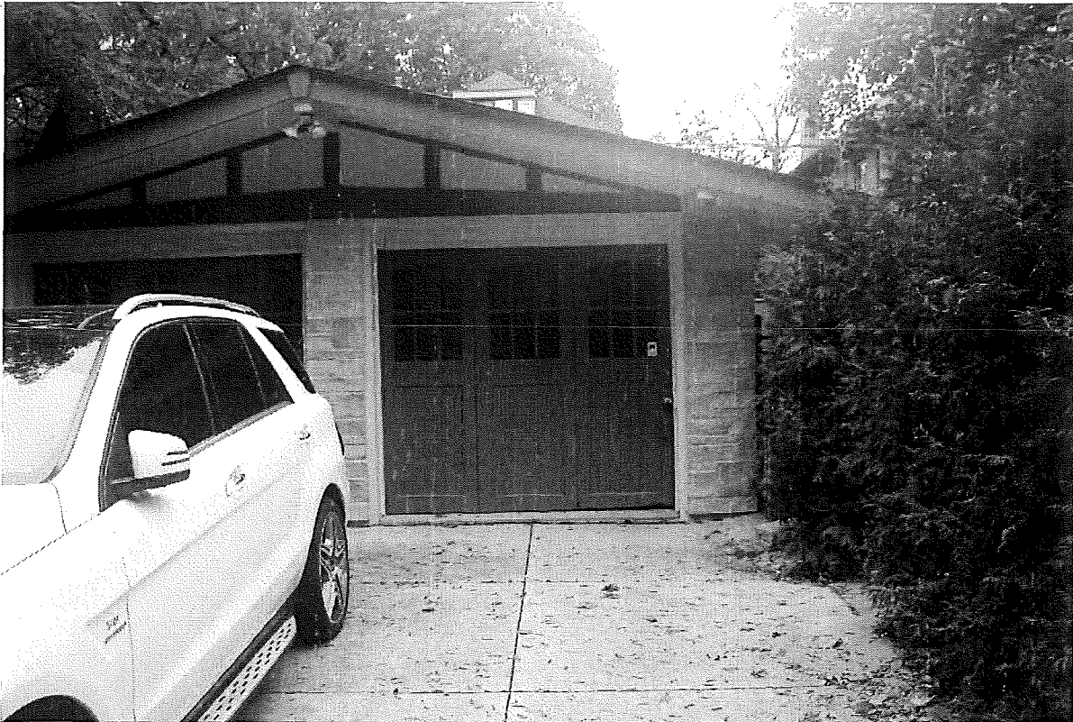
Photograph 4: New Wall Application (October 29, 2021)
