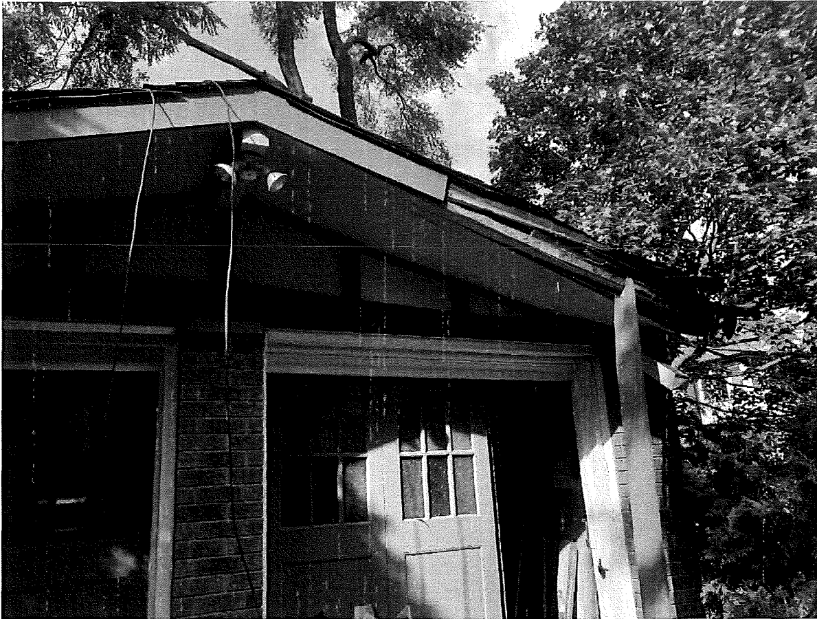
Photograph 2: Front Elevation - Original Brick (October 20, 2020)
